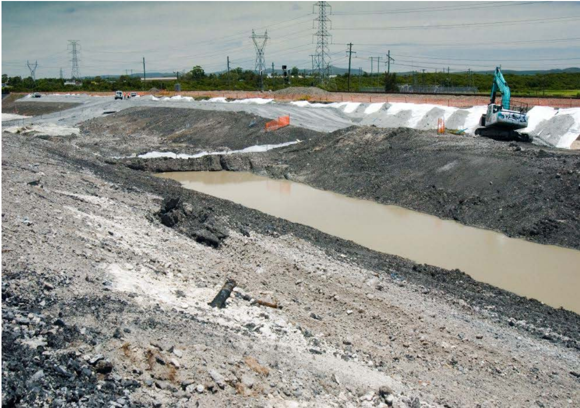
Figure 2.8: Rail Formation Construction
