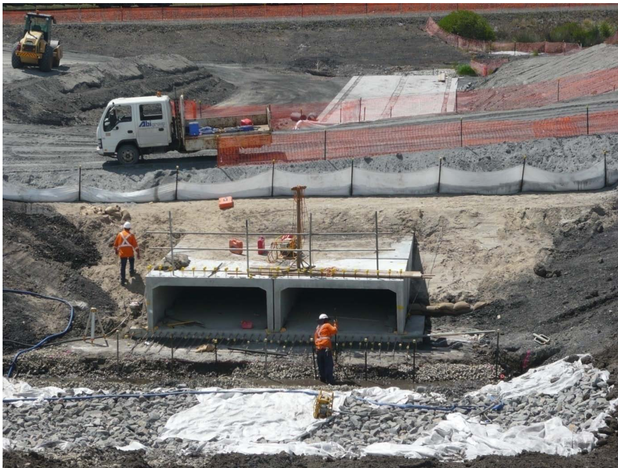
Figure 3.4.1: Construction of Stormwater Infrastructure:
