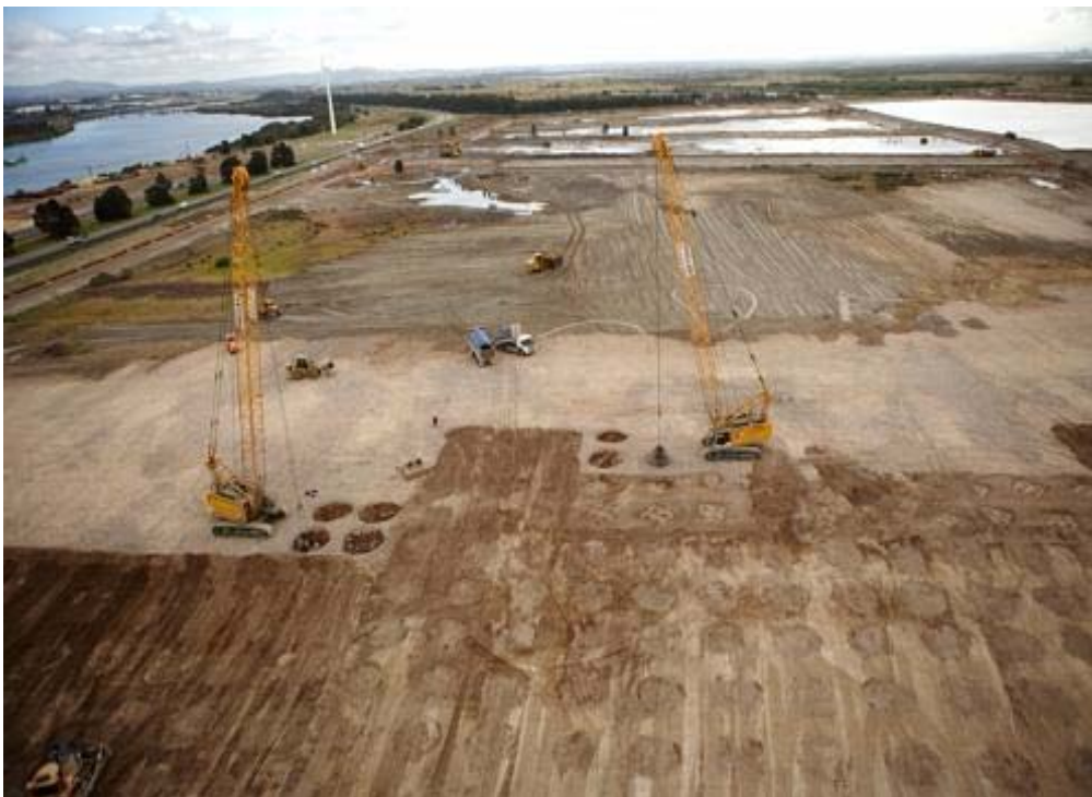
Figure 2.4: Ground Improvement Works
