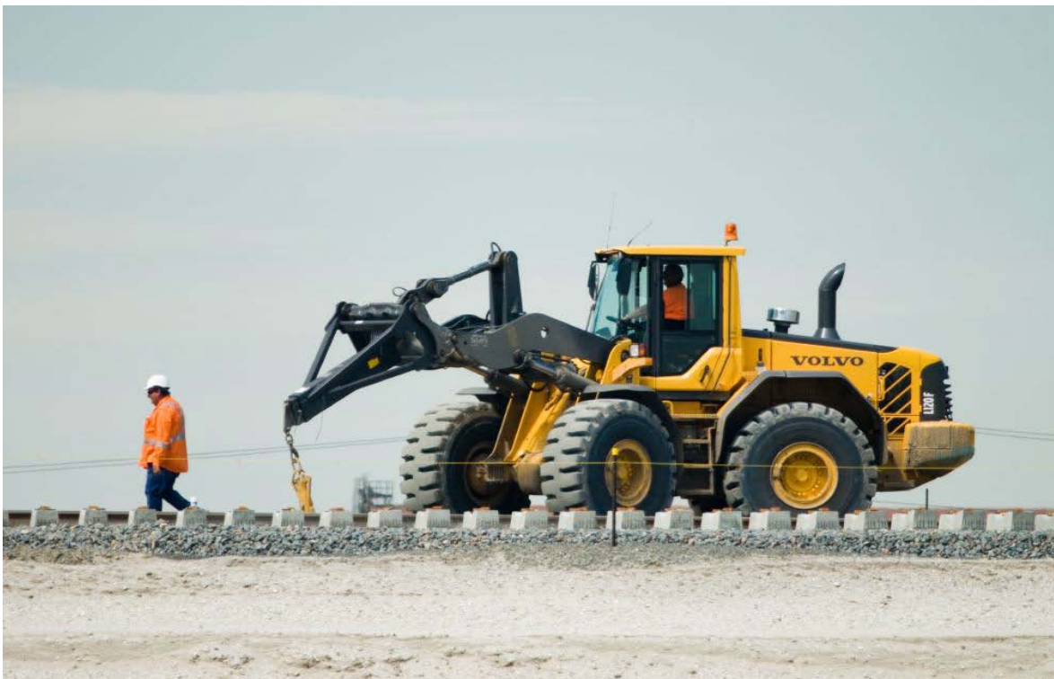
Figure 2.9: Rail Instillation Works
