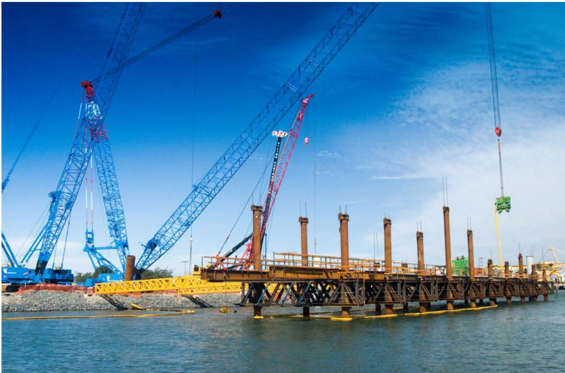
Figure 2.7: Wharf Construction Works
