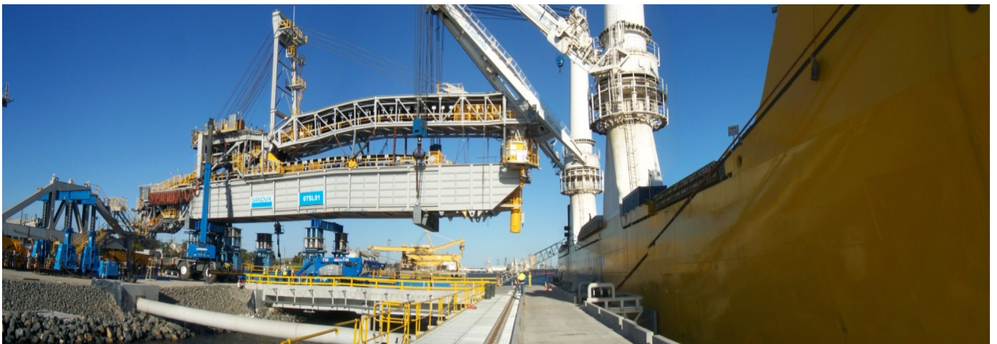
Figure 2.6: Shiploader Unloaded onto NCIG Wharf
