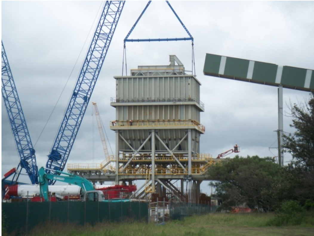
Figure 2.8: Erection of Buffer Bin
