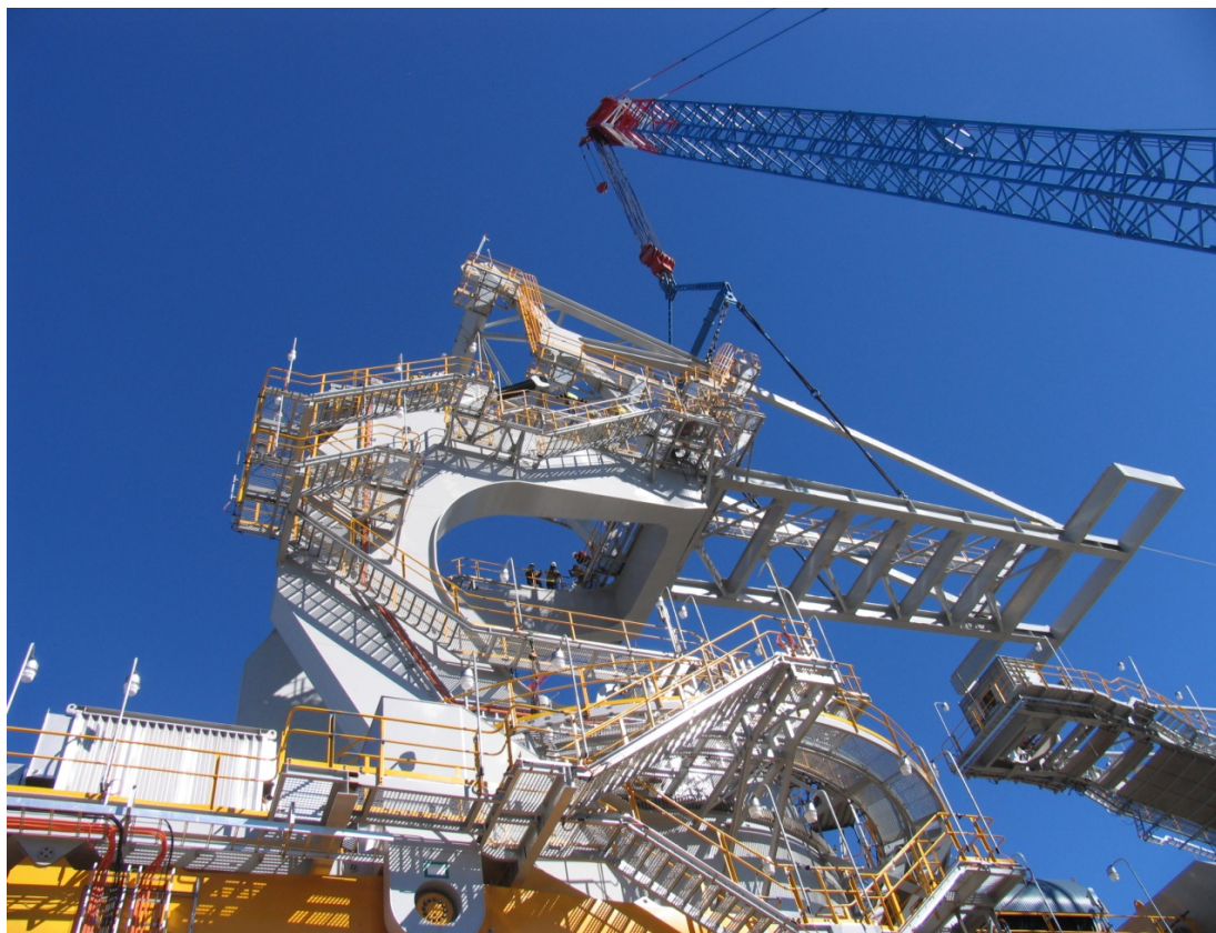
Figure 2.4: Stacker Reclaimer Erection
