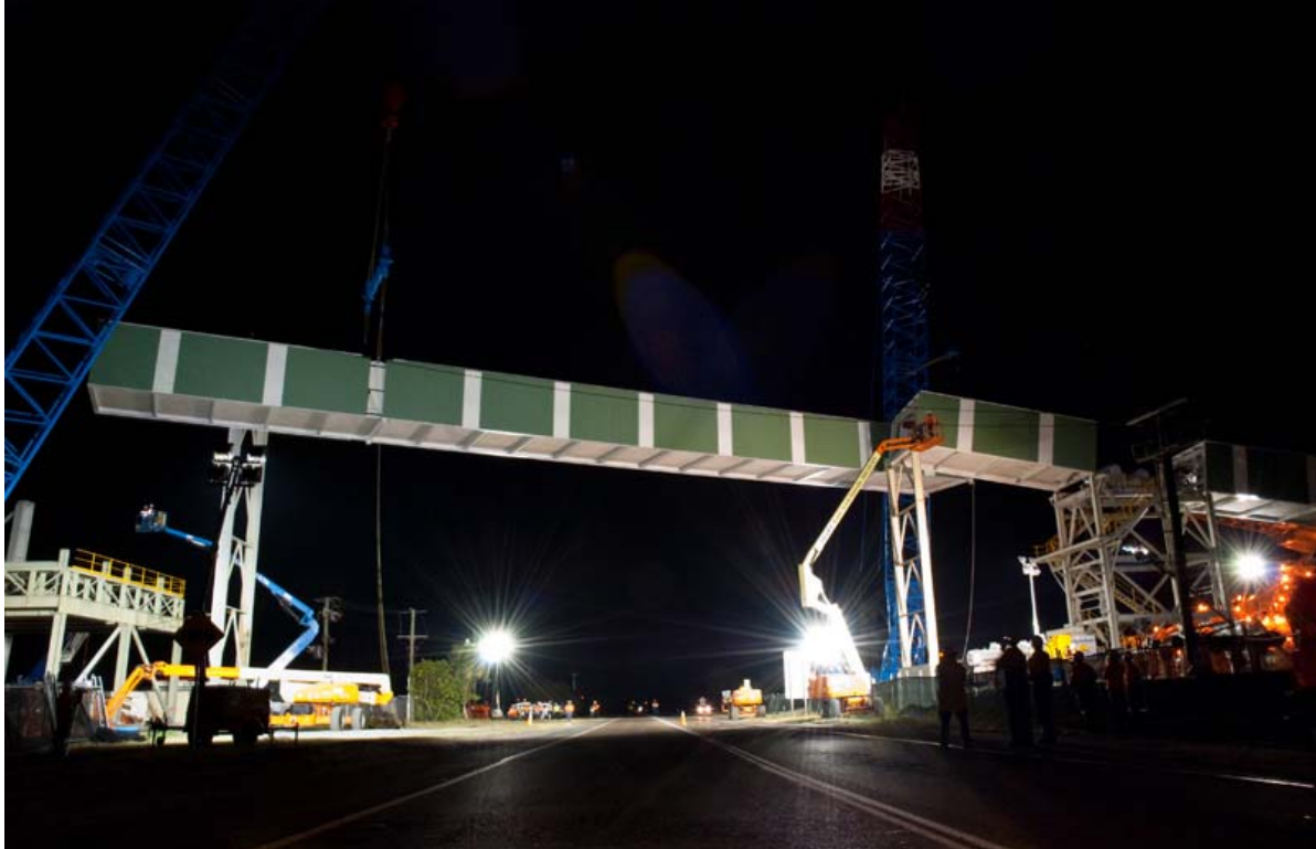
Figure 2.7: Erection of Gantry Linking Stockyard to Wharf
