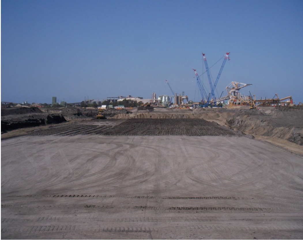
Figure 2.1: Earthworks on SR02 Machine Berm
