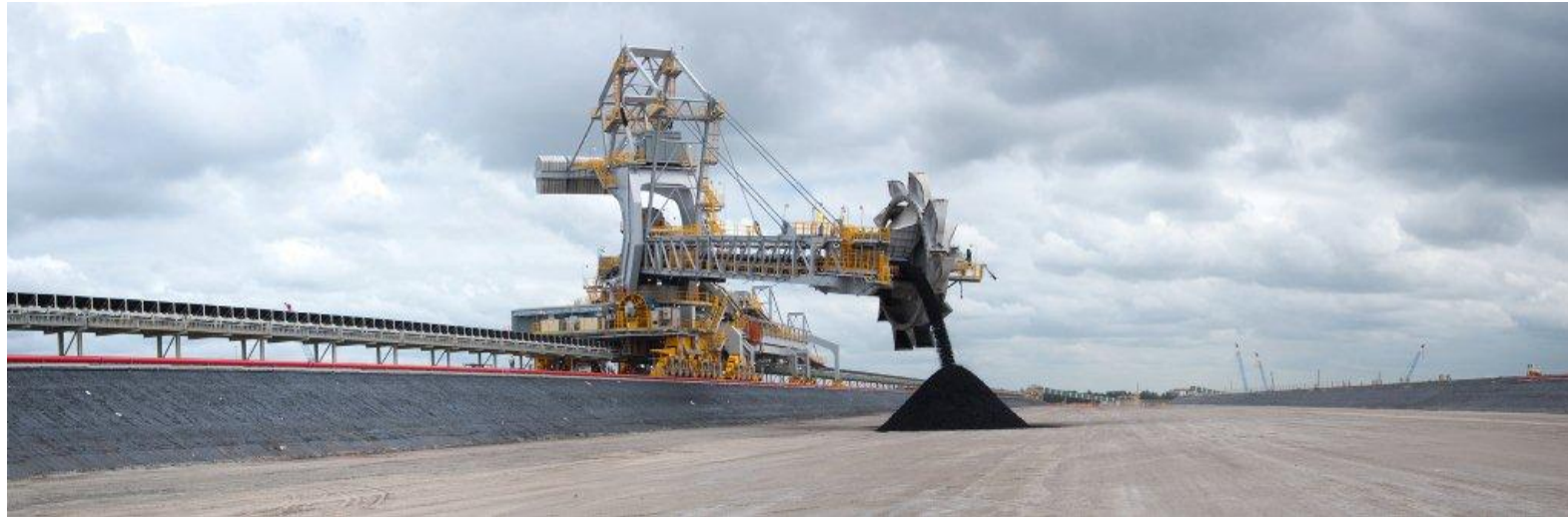
Figure 2.17: Stacking “Sacrificial” Coal on Stockyard
