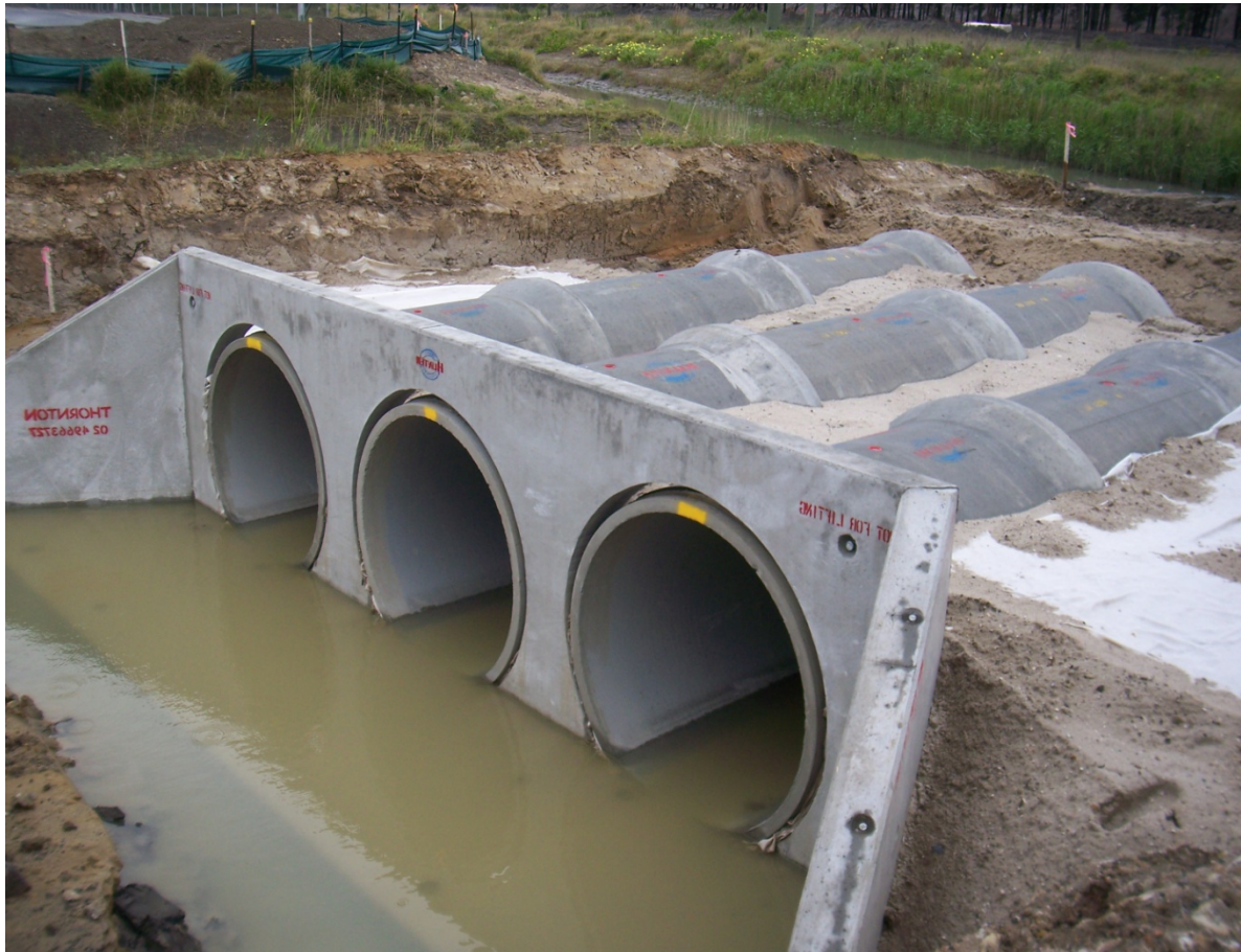
Figure 3.4.1: Construction of Stormwater Infrastructure
