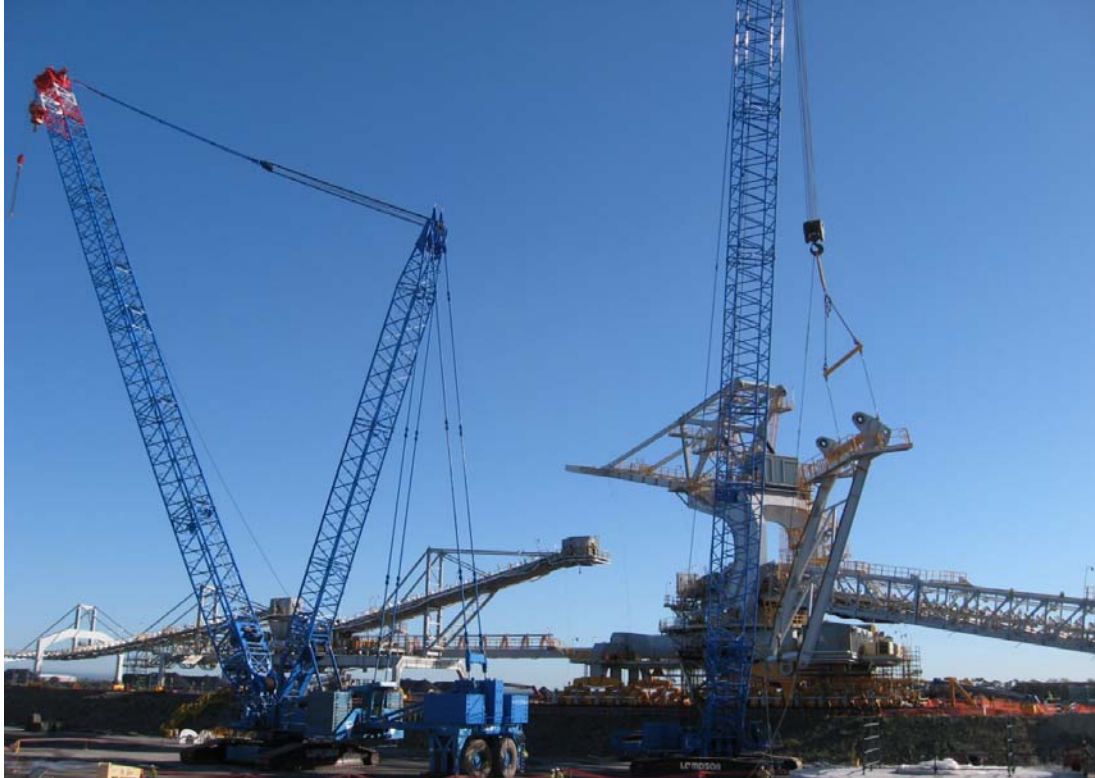
Figure 2.3: Stacker Reclaimer Erection
