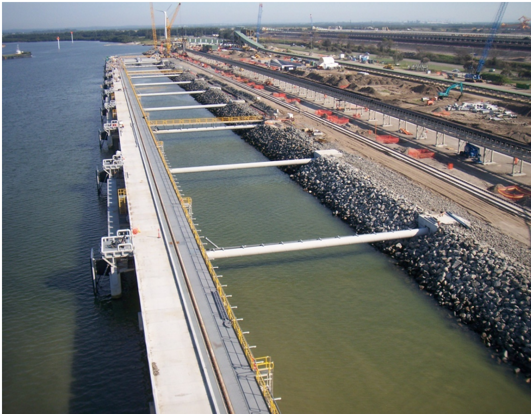
Figure 2.2: Completion of Terminal Berths
