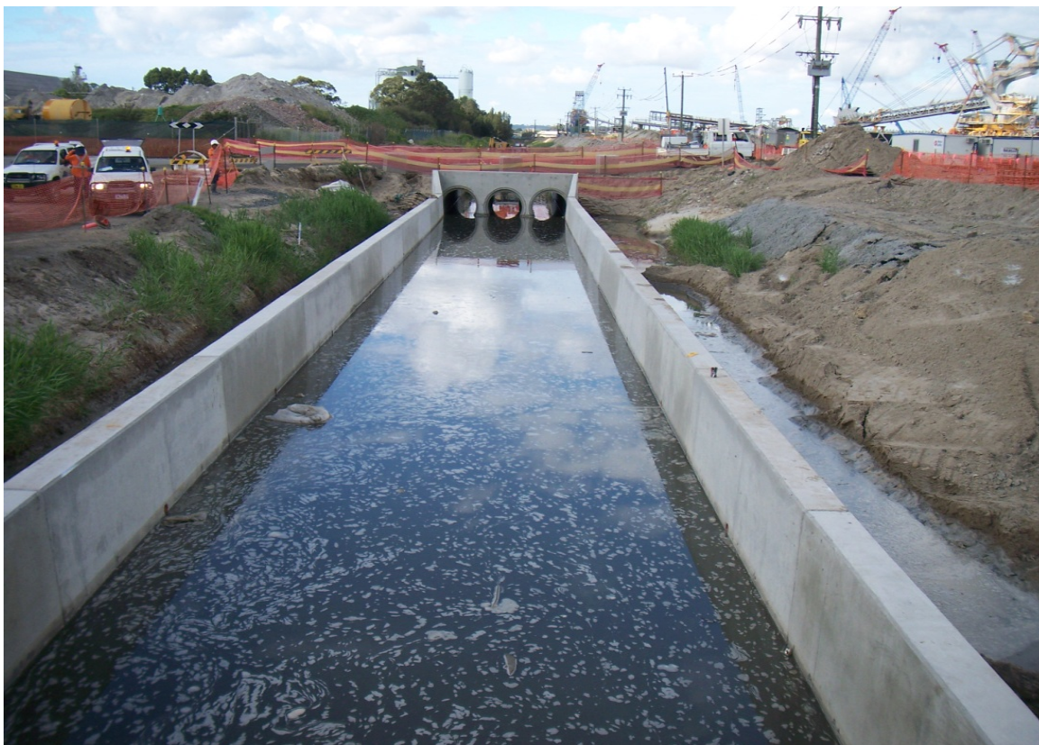
Figure 3.4.2: Completed Stormwater Infrastructure
