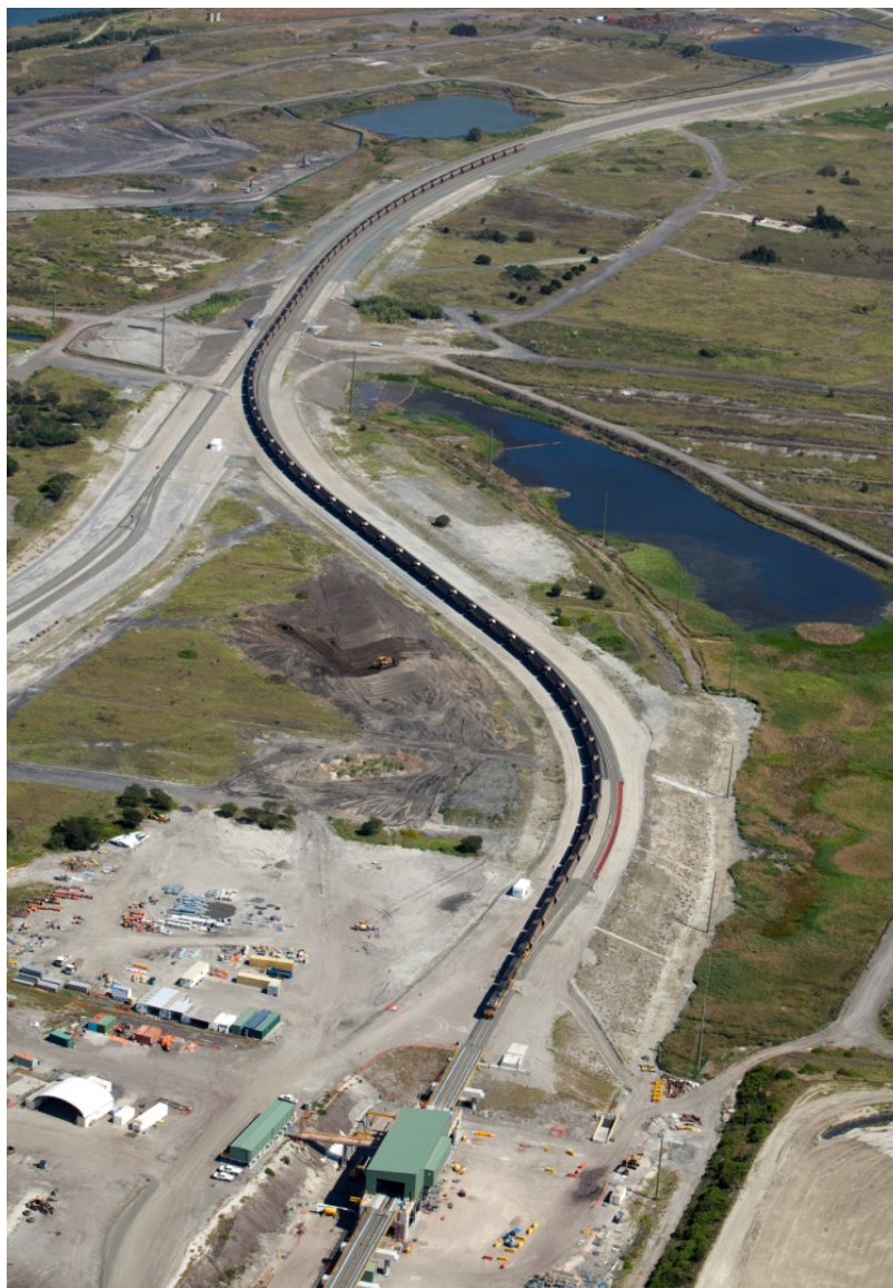
Figure 2.15: Train Arrival at NCIG Terminal
