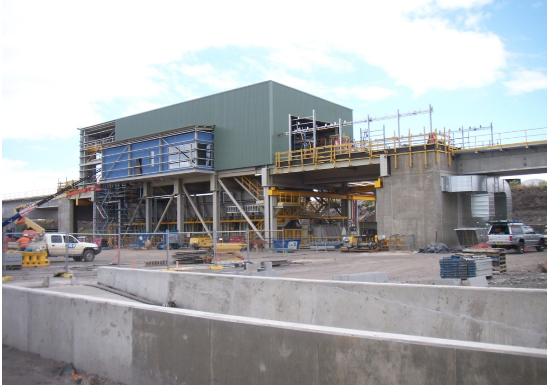
Figure 2.11: Rail Unloading Station Nearing Completion
