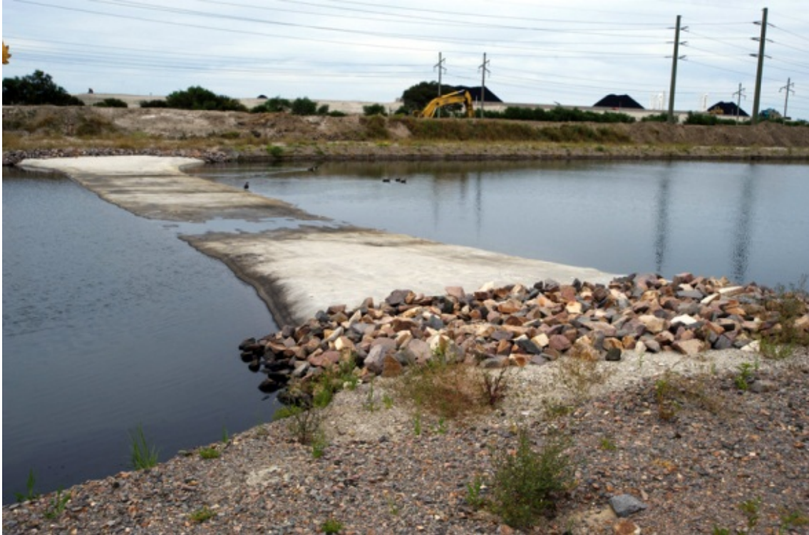
Figure 3.4.1: Settling Pond Infrastructure
