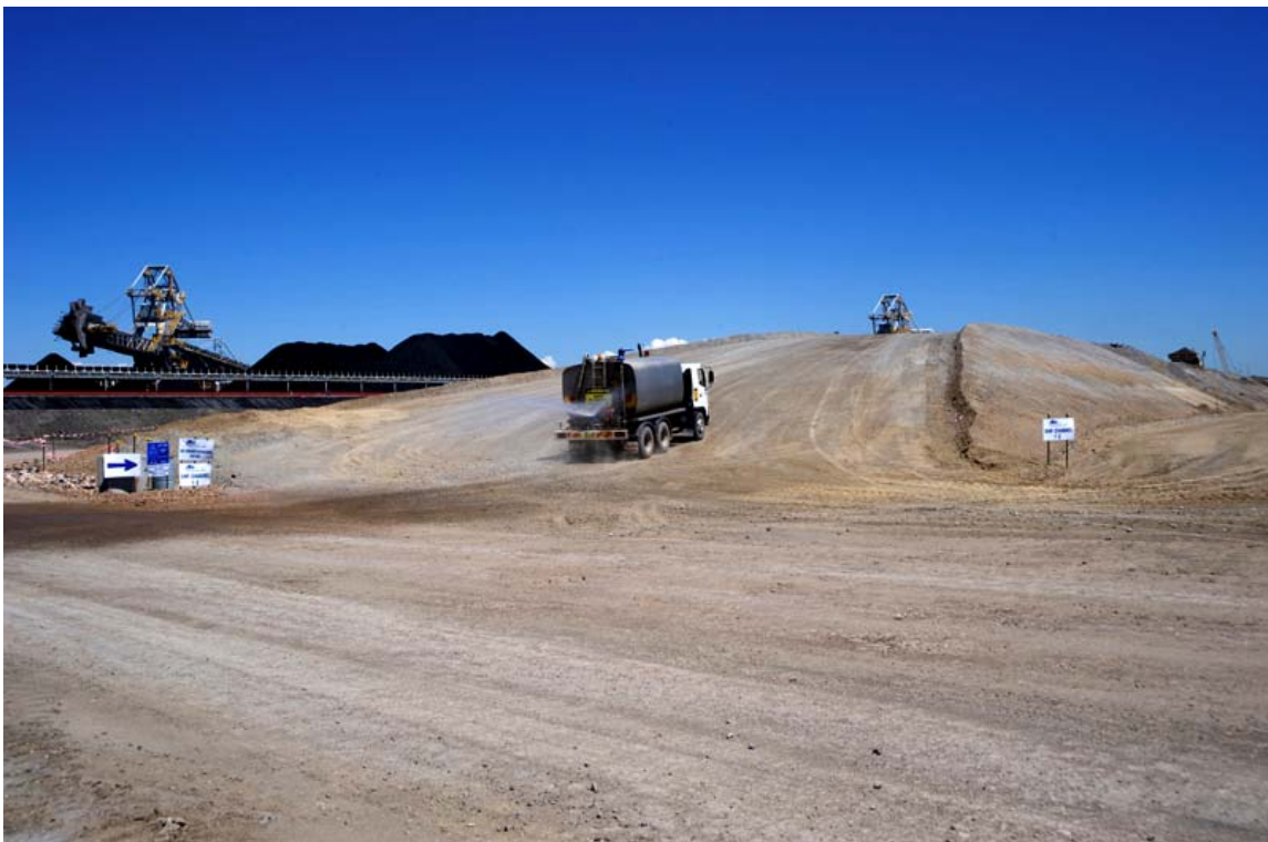
Figure 2.24: Dust Suppression on SR03 Berm
