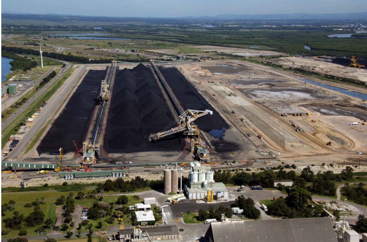
Figure 2.13: NCIG Stockyard, showing operational stockyard and Stage 2AA construction
