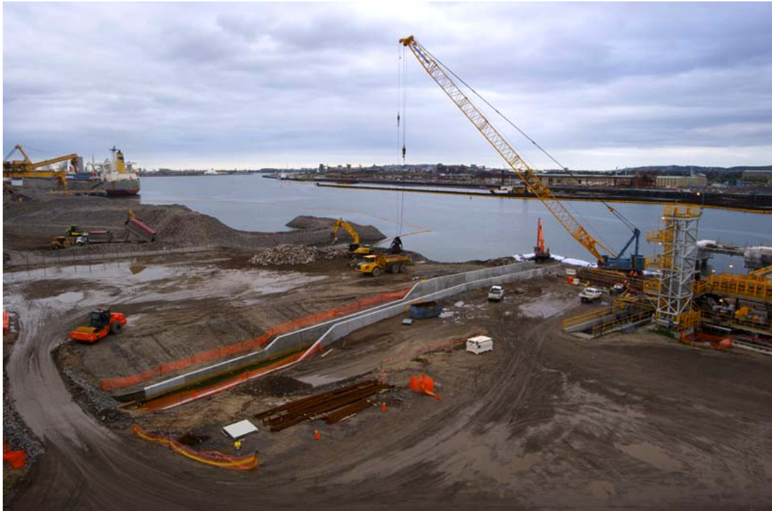
Figure 2.19: Completion of Stage 1 Wharf Structure
