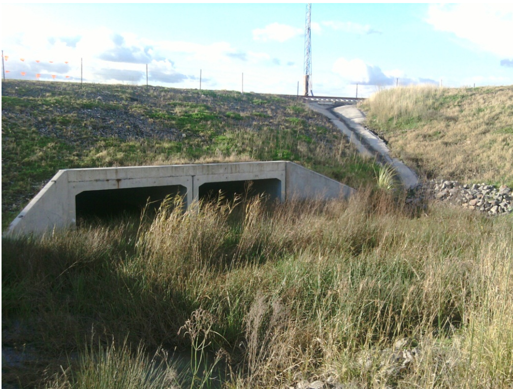
Figure 3.10.2: Installed Rail Culverts for Green and Golden Bell Frog Movement
