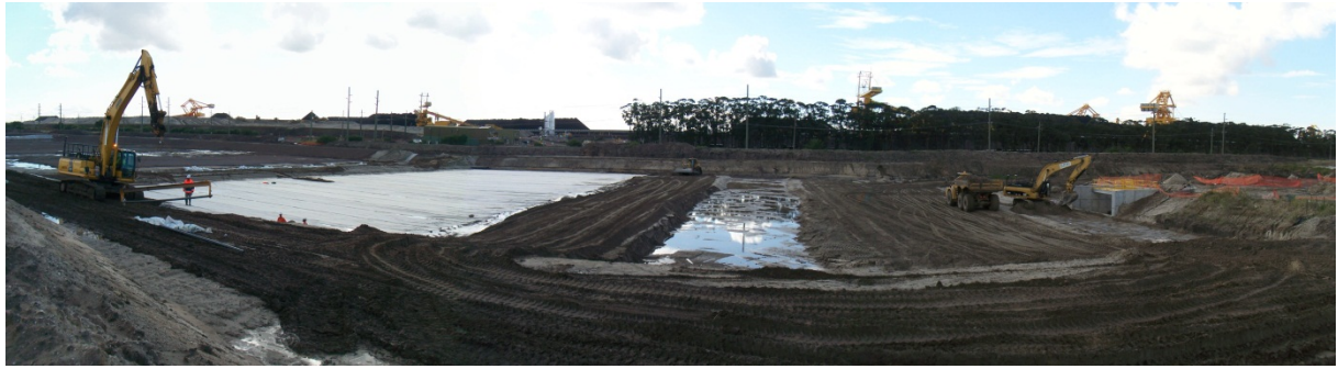
Figure 2.15: Clearwater Pond construction
