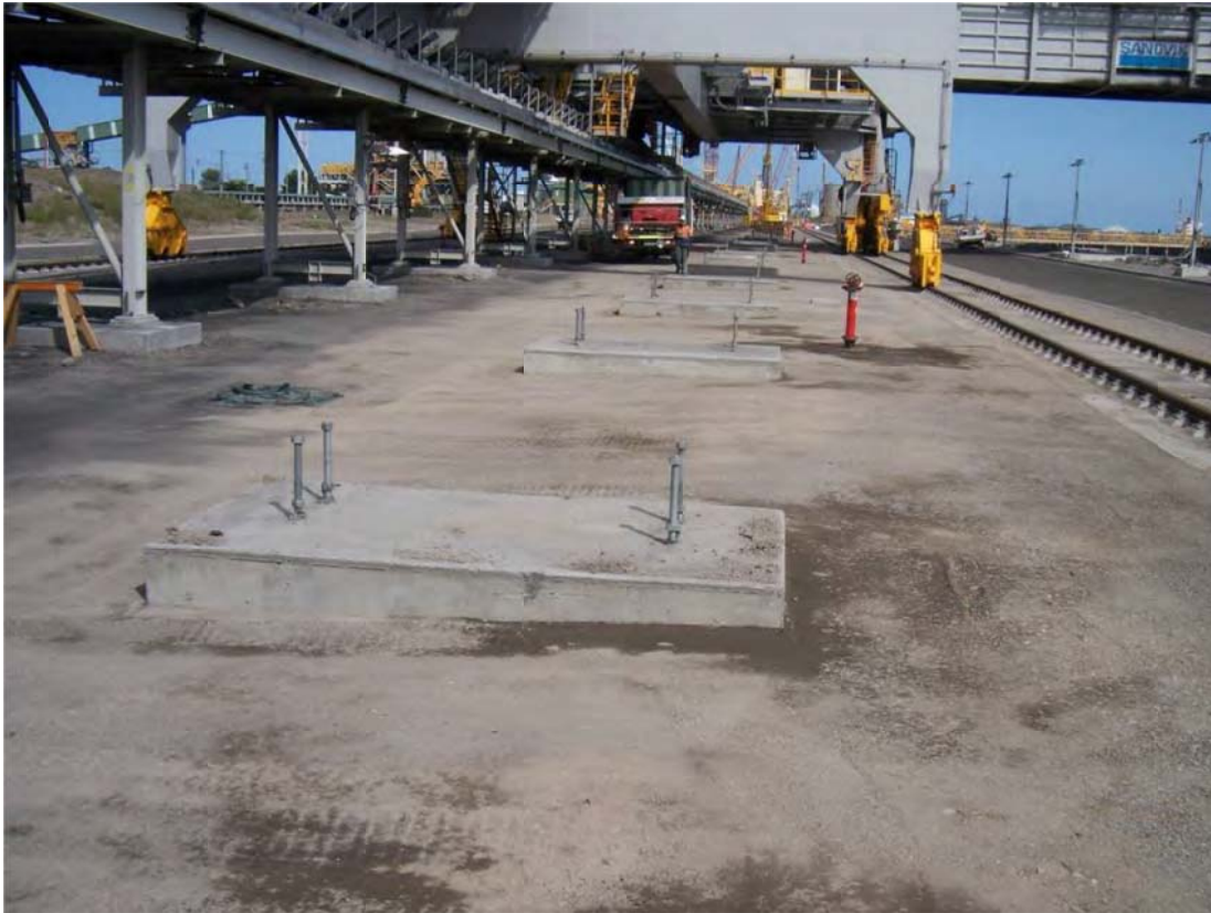
Figure 2.25: Foundations for Conveyor 22
