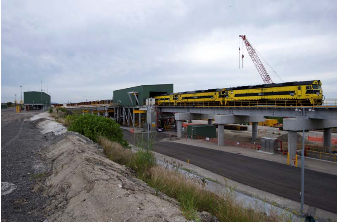
Figure 2.5: Train at Dump Station 1
