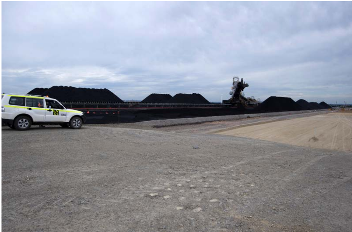
Figure 2.14: Construction of SR03 Berm
