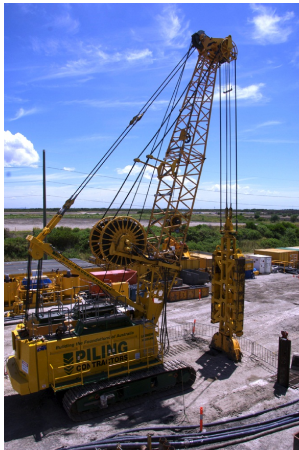
Figure 2.20: Excavation for Diaphragm Wall
