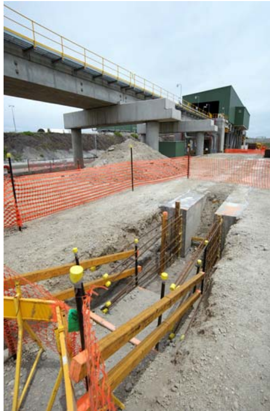
Figure 2.17: Development of Diaphragm Wall for Dump Station 2
