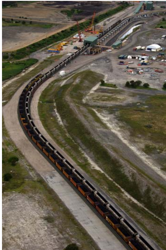
Figure 2.9: Train unloading at Dump Station 1 and Train parked adjacent (left)
