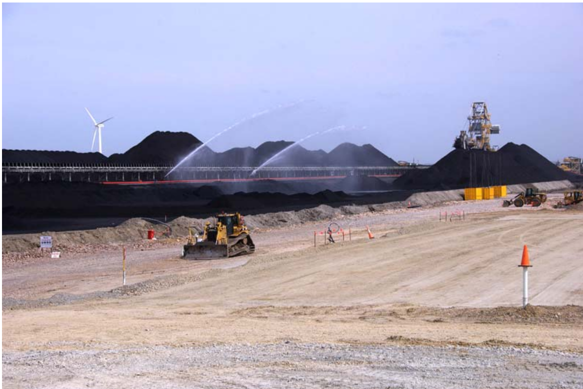
Figure 2.6: Coal Stockyard Dust Suppression Sprays
