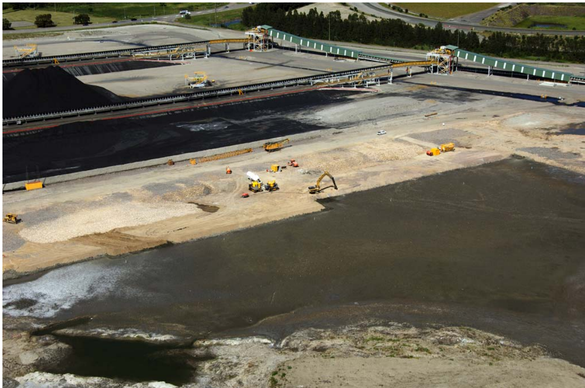
Figure 2.18: Soil Mixing activities
