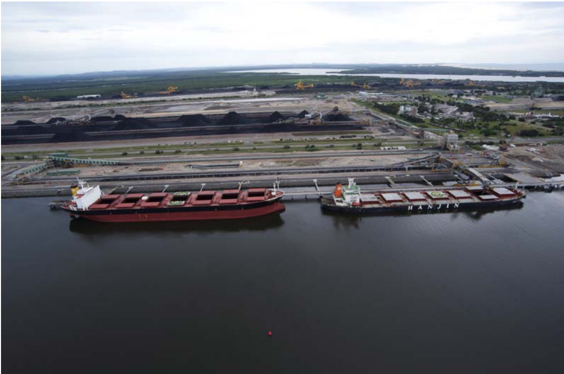
Figure 2.7: Shiploading (K8) and Ship at Berth (K9)
