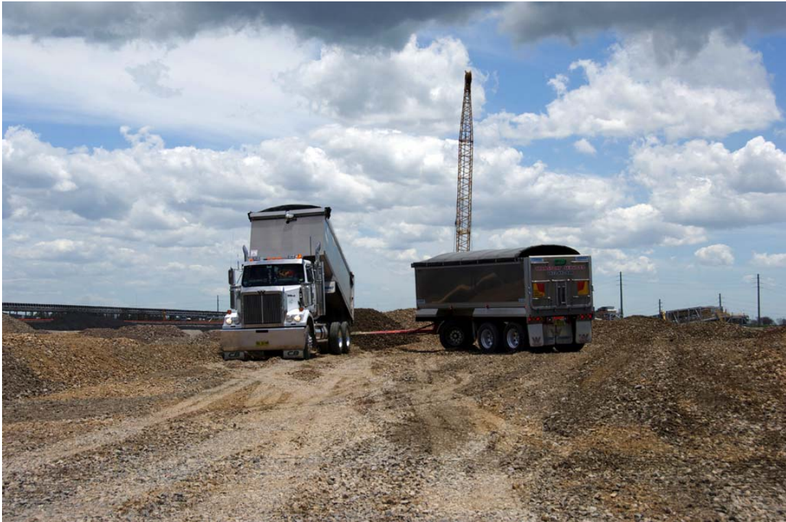
Figure 2.23: Delivery of materials for Dynamic Replacement
