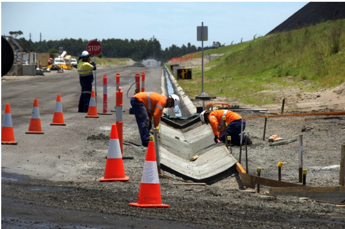
Figure 3.4.2: Construction of Stormwater Infrastructure
