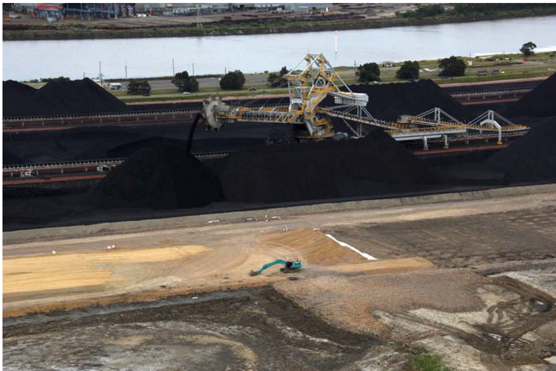
Figure 2.8: Stacking Operations over SR02
