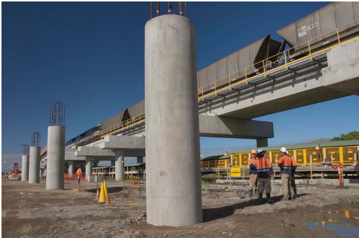
Figure 2.21: Piling/Viaduct for duplication of rail track
