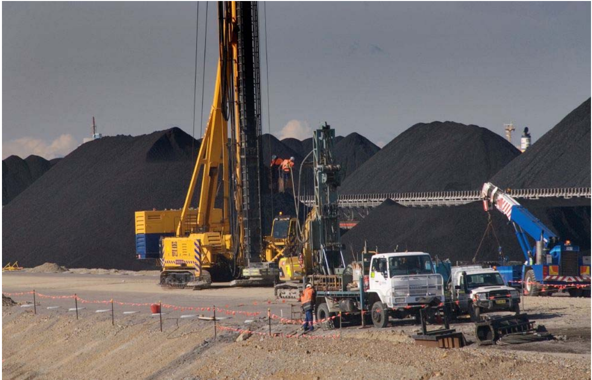
Figure 2.16: Concrete piling for CV10
