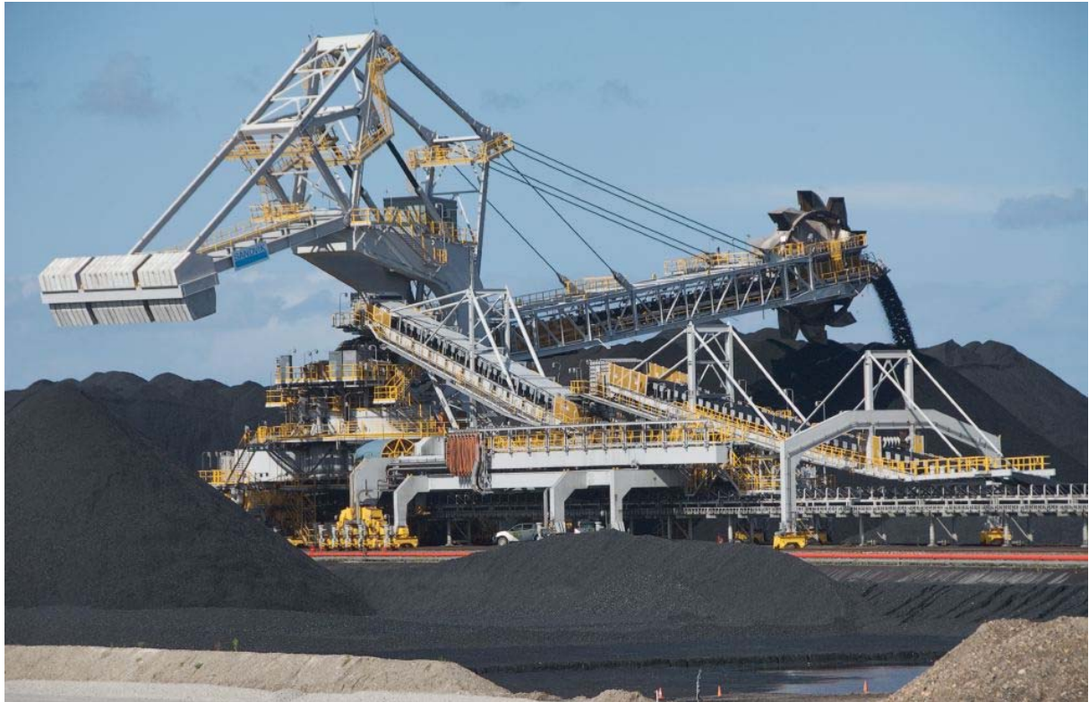
Figure 2.4: Stacking over SR02 at NCIG Terminal
