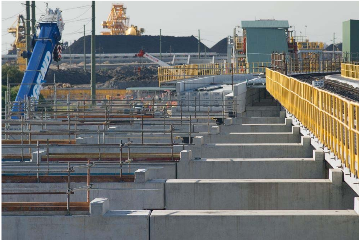
Figure 2.14: Extension of Viaduct for duplication of rail track
