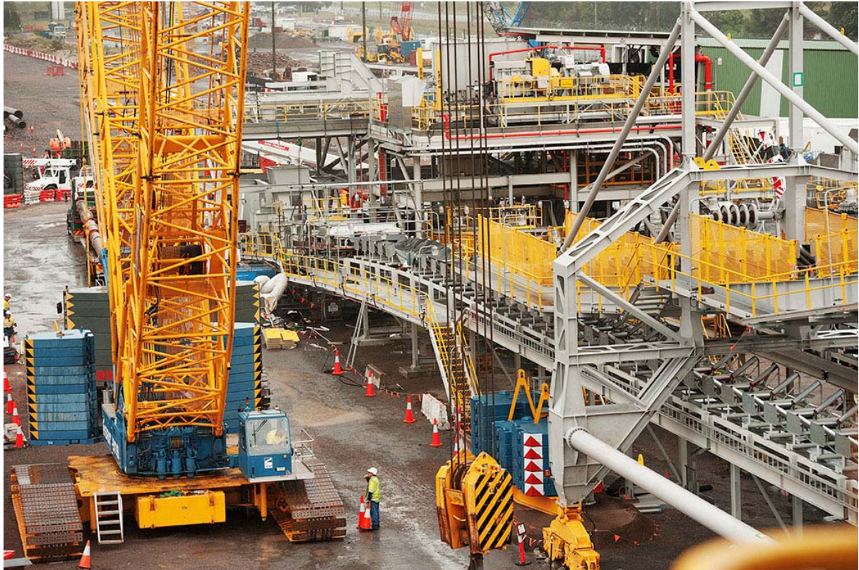
Figure 2.12: Construction of CV22 and extension of TH12
