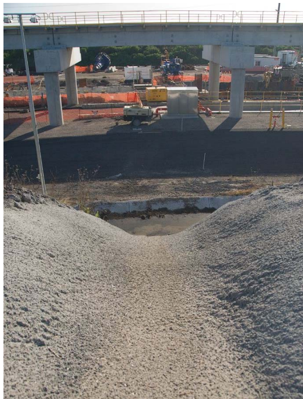
Figure 3.4.2: Concrete-lined drain leading to Concrete-lined Water Management Pond
