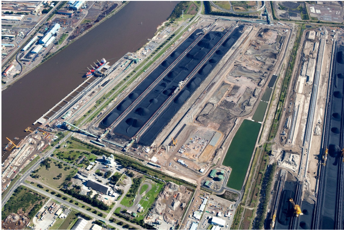
Figure 2.8: Overview of NCIG Terminal (June 2011)
