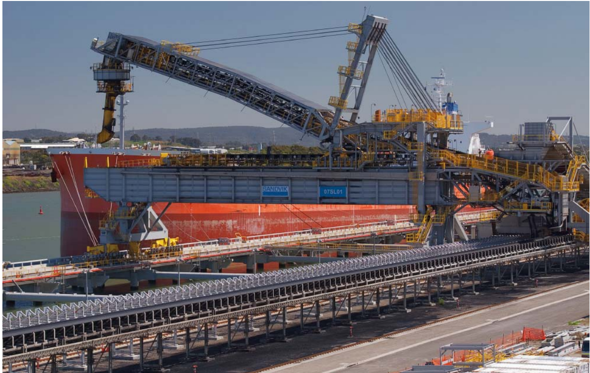
Figure 2.6: Shiploader 1 in operation at K9 Wharf
