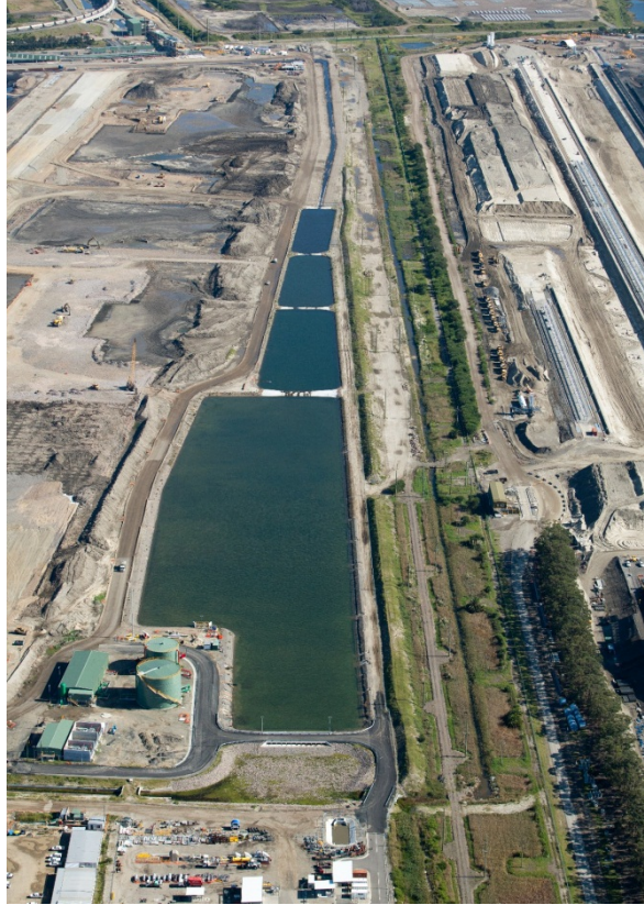
Figure 3.4.1: Settling Pond Infrastructure
