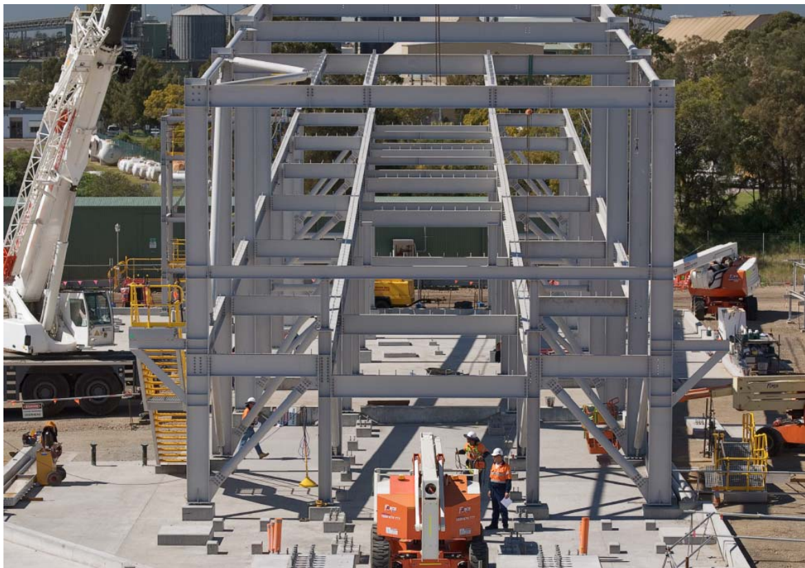
Figure 2.23: Construction of TH08
