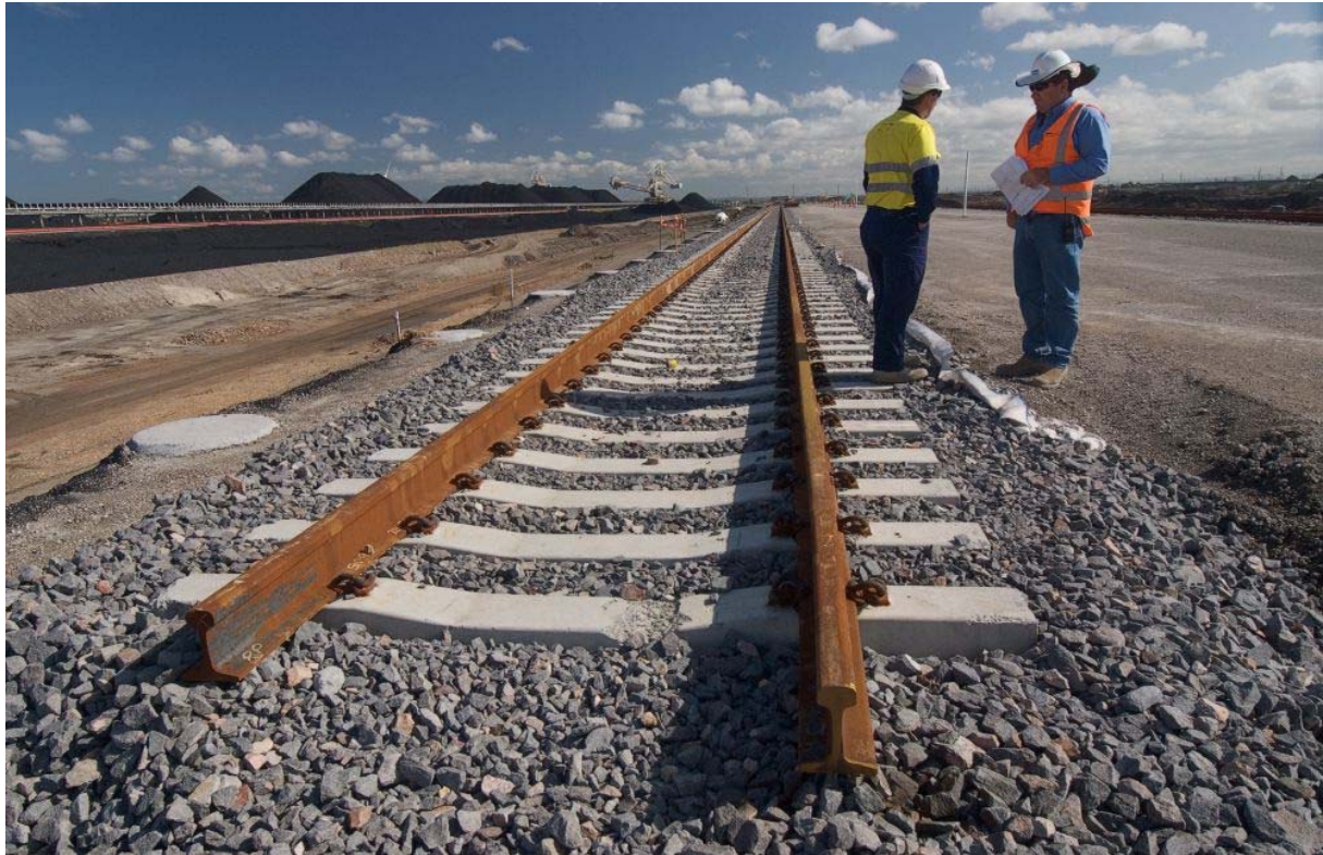
Figure 2.20: SR03 Rail Track
