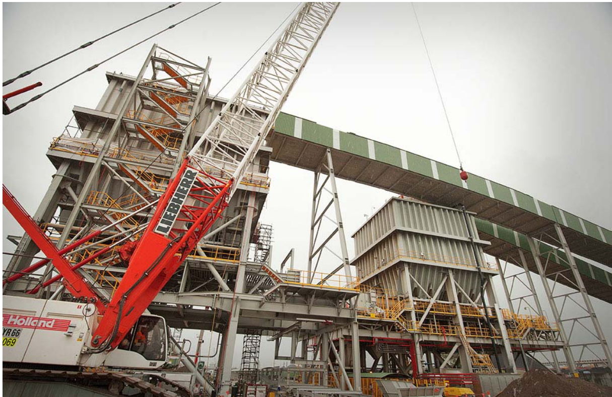
Figure 2.24: Construction of BN02 and CV13 gallery
