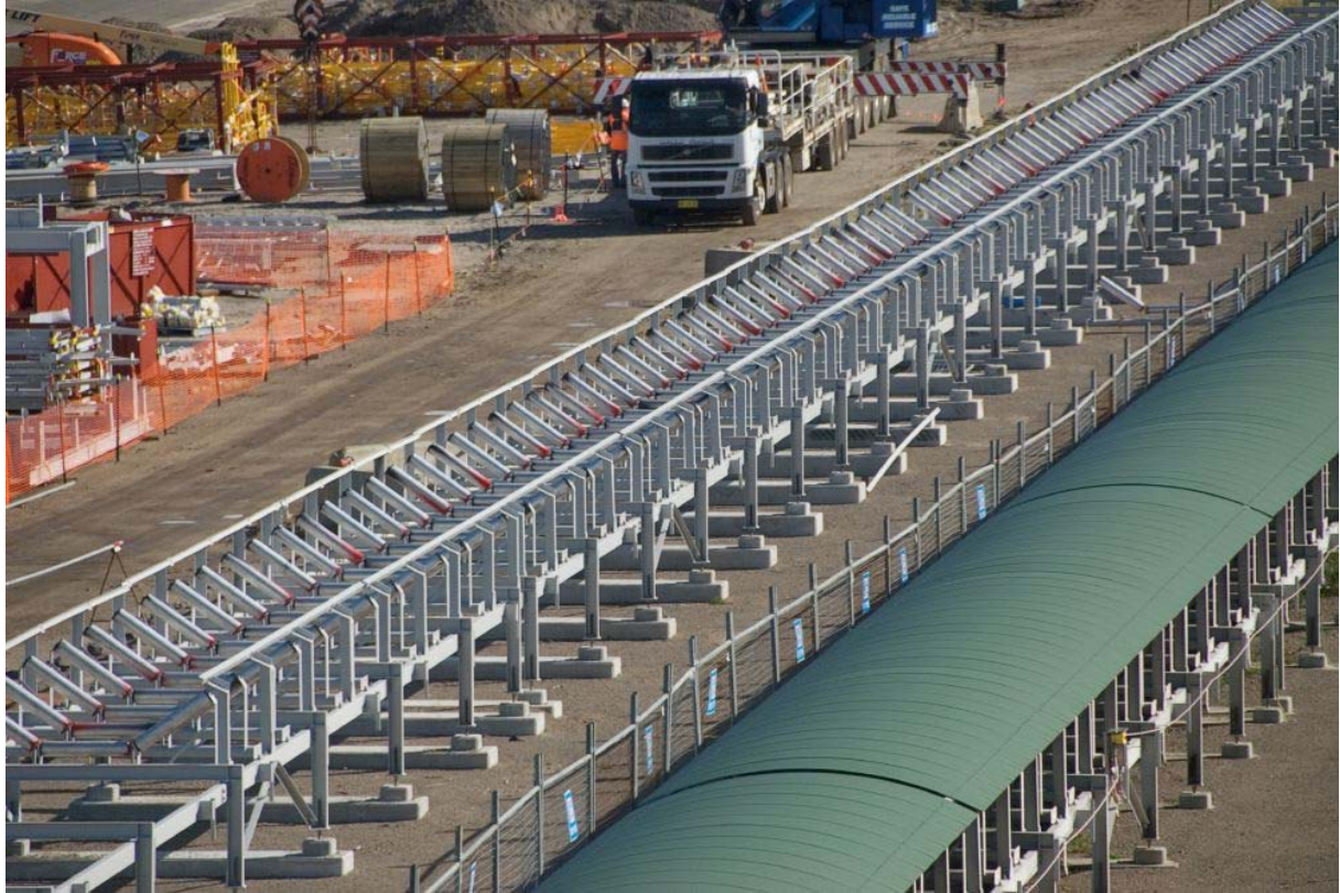
Figure 2.18: Construction of CV16
