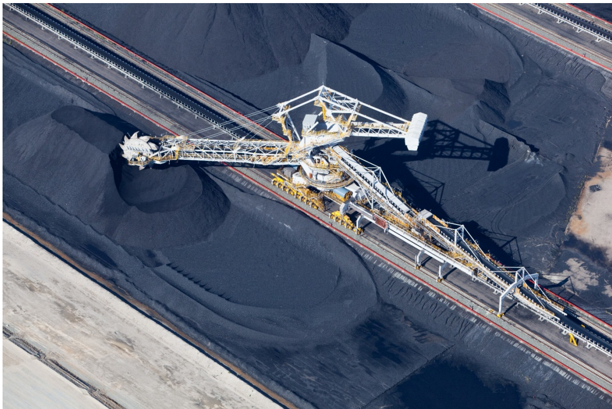
Figure 2.3: SR02 Reclaiming at NCIG Terminal
