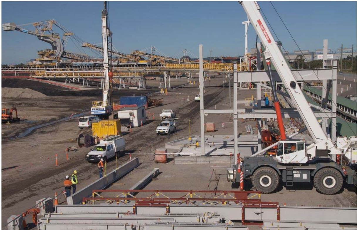
Figure 2.17: Construction of TH04
