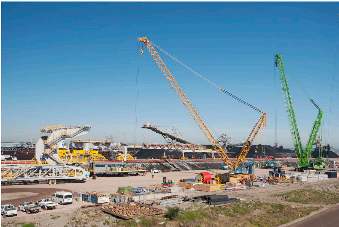
Figure 16: Construction of Stacker Reclaimer 4.
