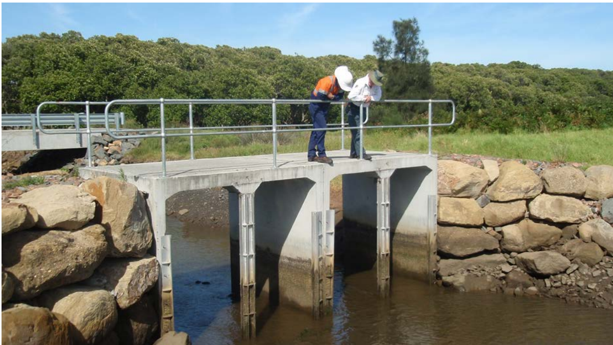
Figure 34: Creek 5 Drop board support structure prior to fitting of drop boards
