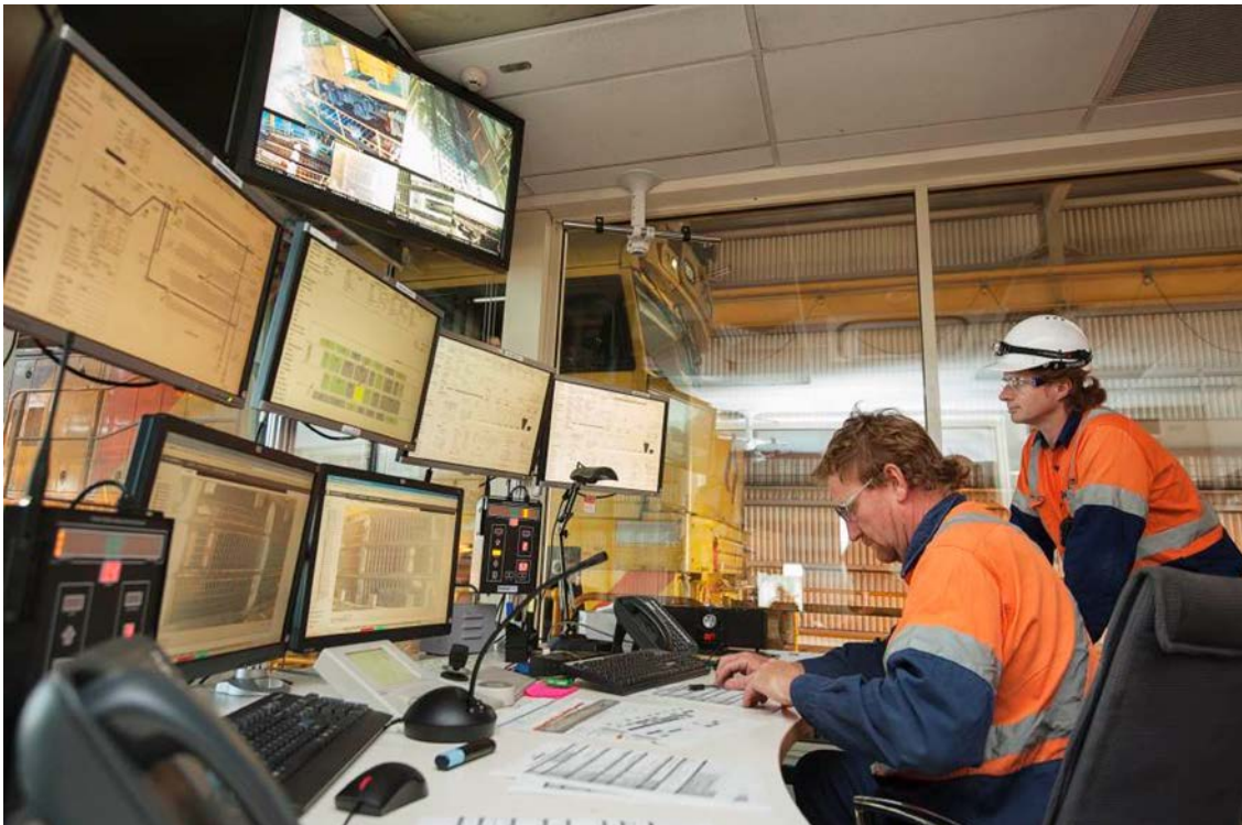
Figure 9: Dump Station Control Room.
