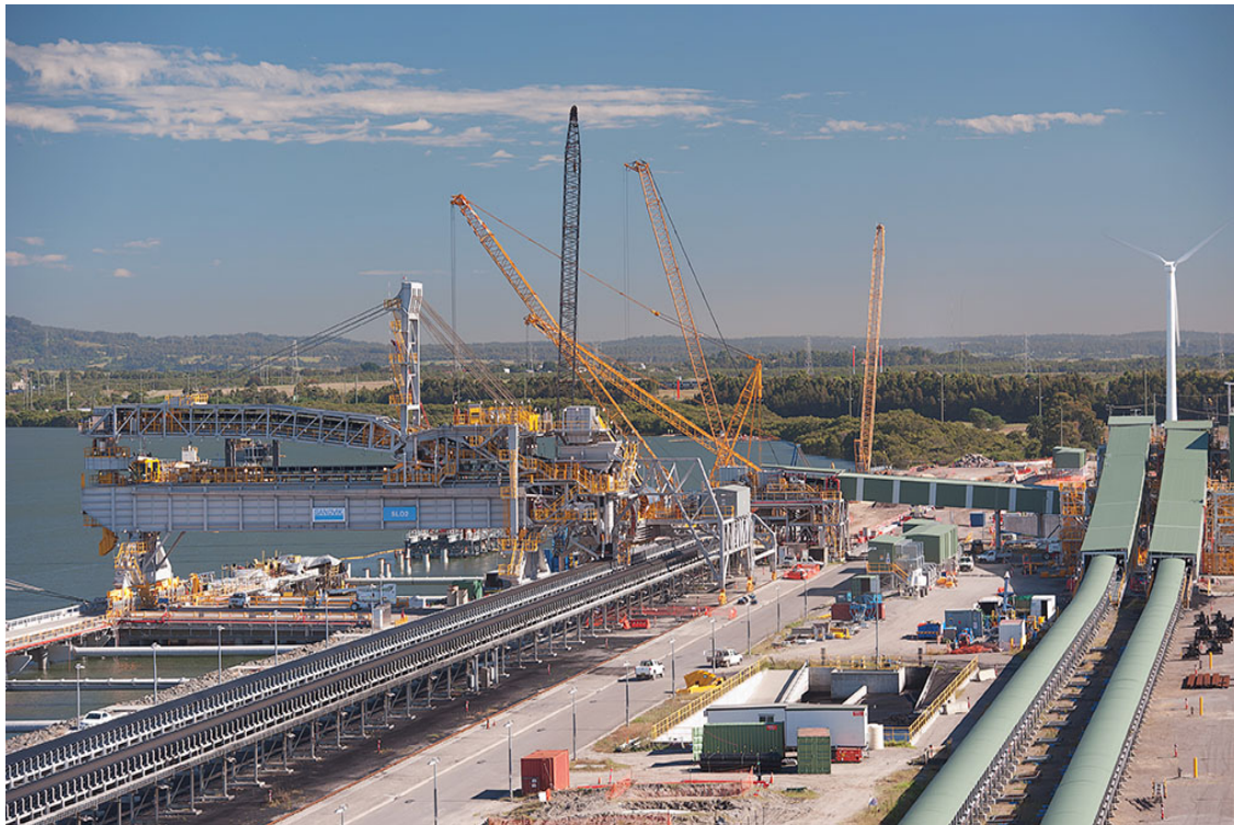
Figure 10: Construction of Ship Loader 2.
