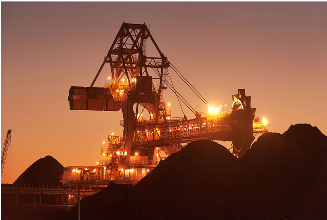
Figure 3: Operation of Stacker Reclaimer 3.
