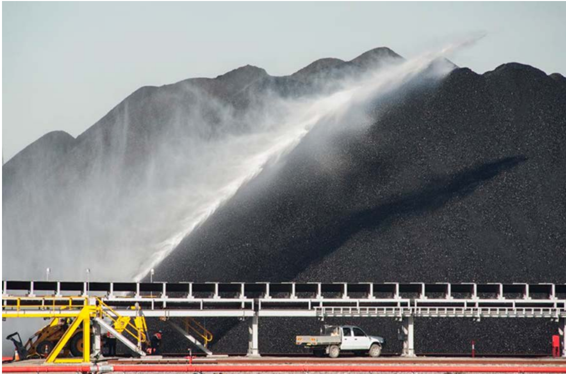
Figure 6: Operation of Stockyard Dust Suppression.
