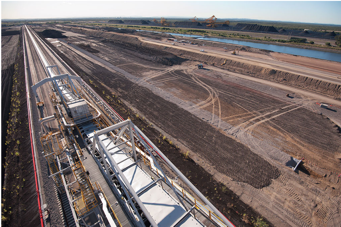
Figure 15: Construction of Stock pad 4 and SR04 Berm.
