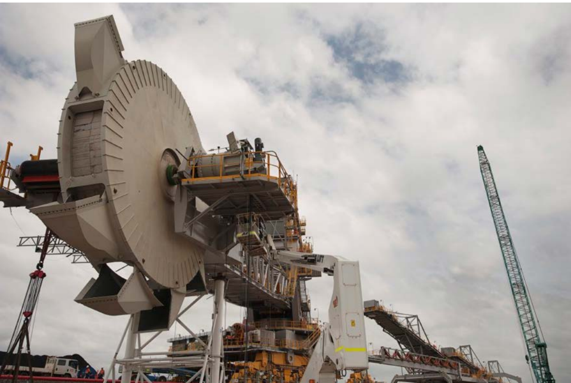
Figure 18: Construction of Stacker Reclaimer 4 Bucket Wheel.
