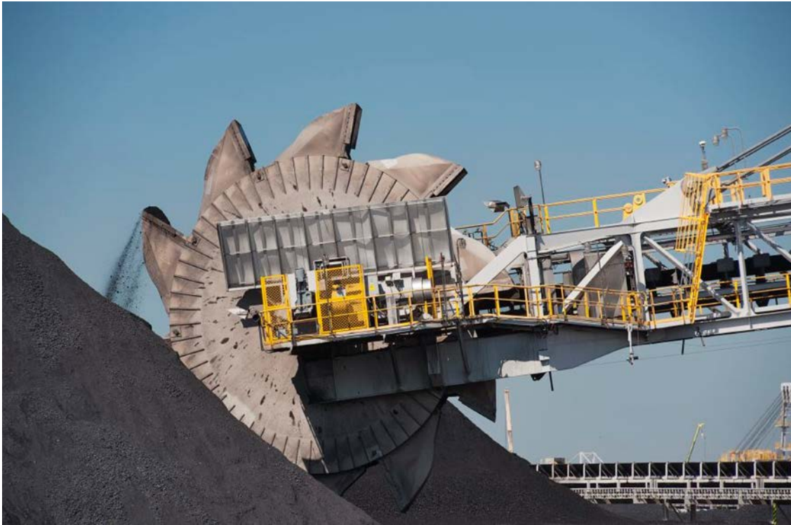
Figure 8: Reclaiming of Coal Stockpile.
