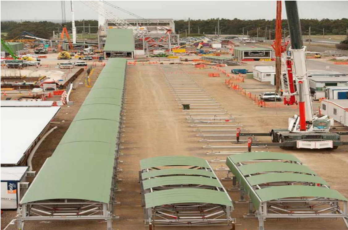
Figure 17: Construction of Conveyors 17 and 18.
