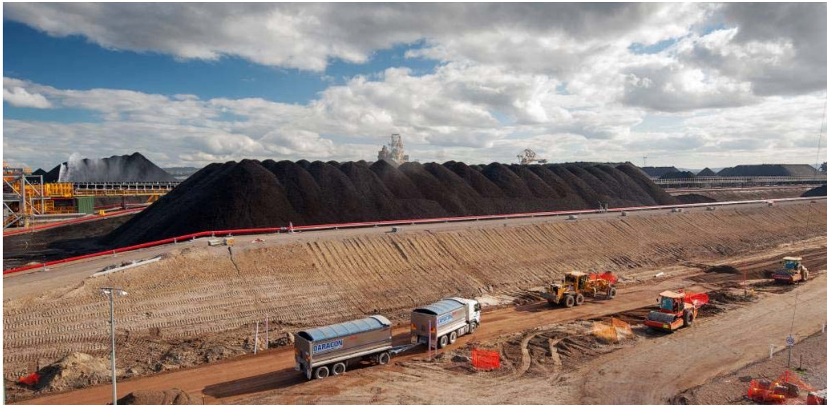
Figure 5: Completion of Northern Haulage Road and minor earthworks.
