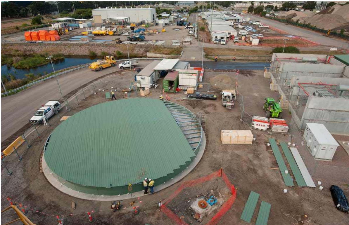
Figure 3: Construction of new Raw Water Tank.
