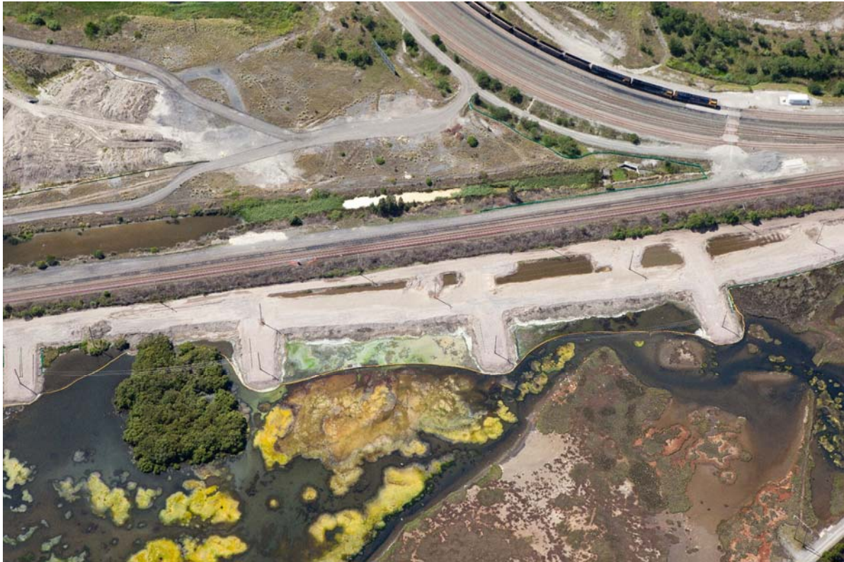
Figure 9: Construction of Western Deviation (Rail Flyover).
