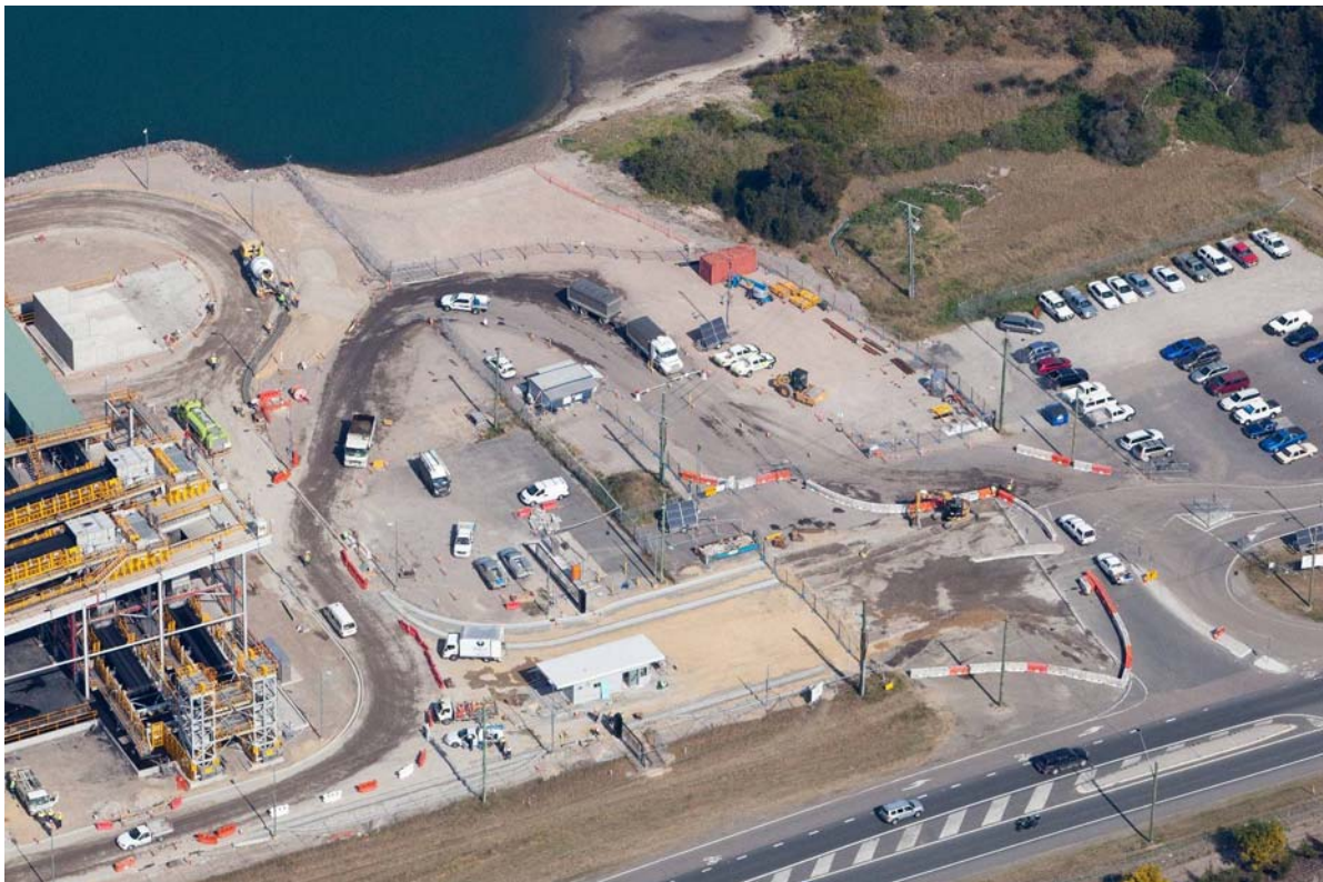
Figure 6: Completion of new Wharf Security Area.
