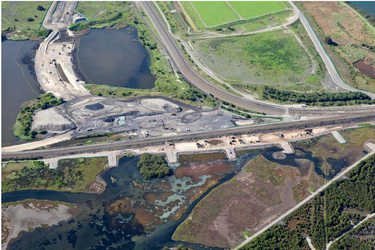
Figure 11: Rail Flyover Construction (flyover and western deviation).
