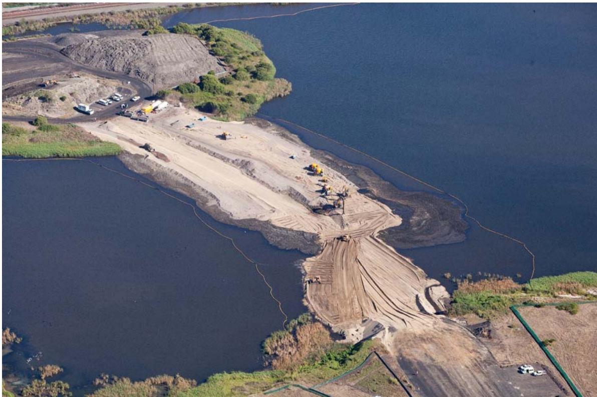
Figure 10: Continuation of Rail Flyover Embankment Construction.
