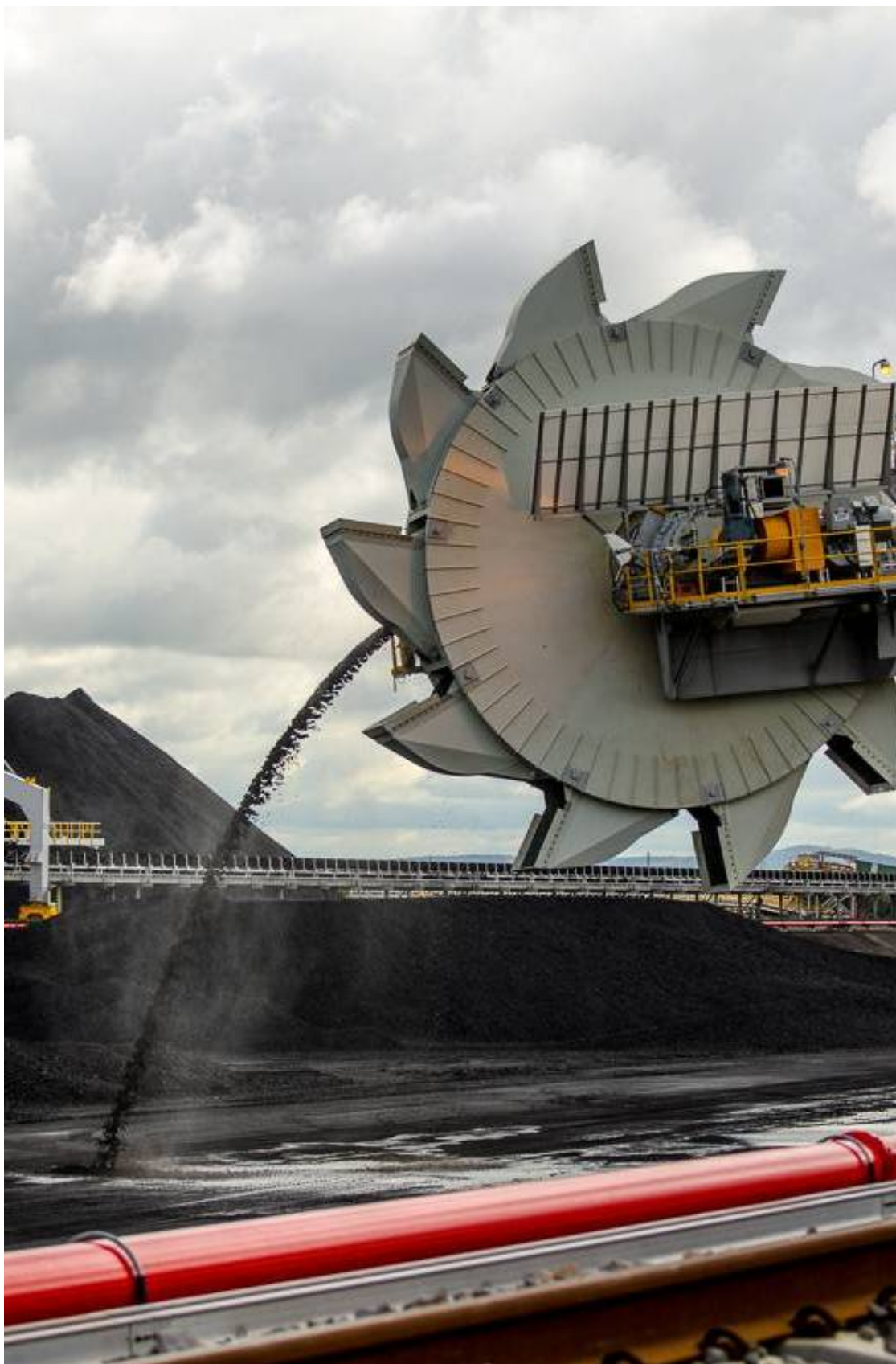
Figure 15: First coal delivered over Stacker Reclaimer 4.
