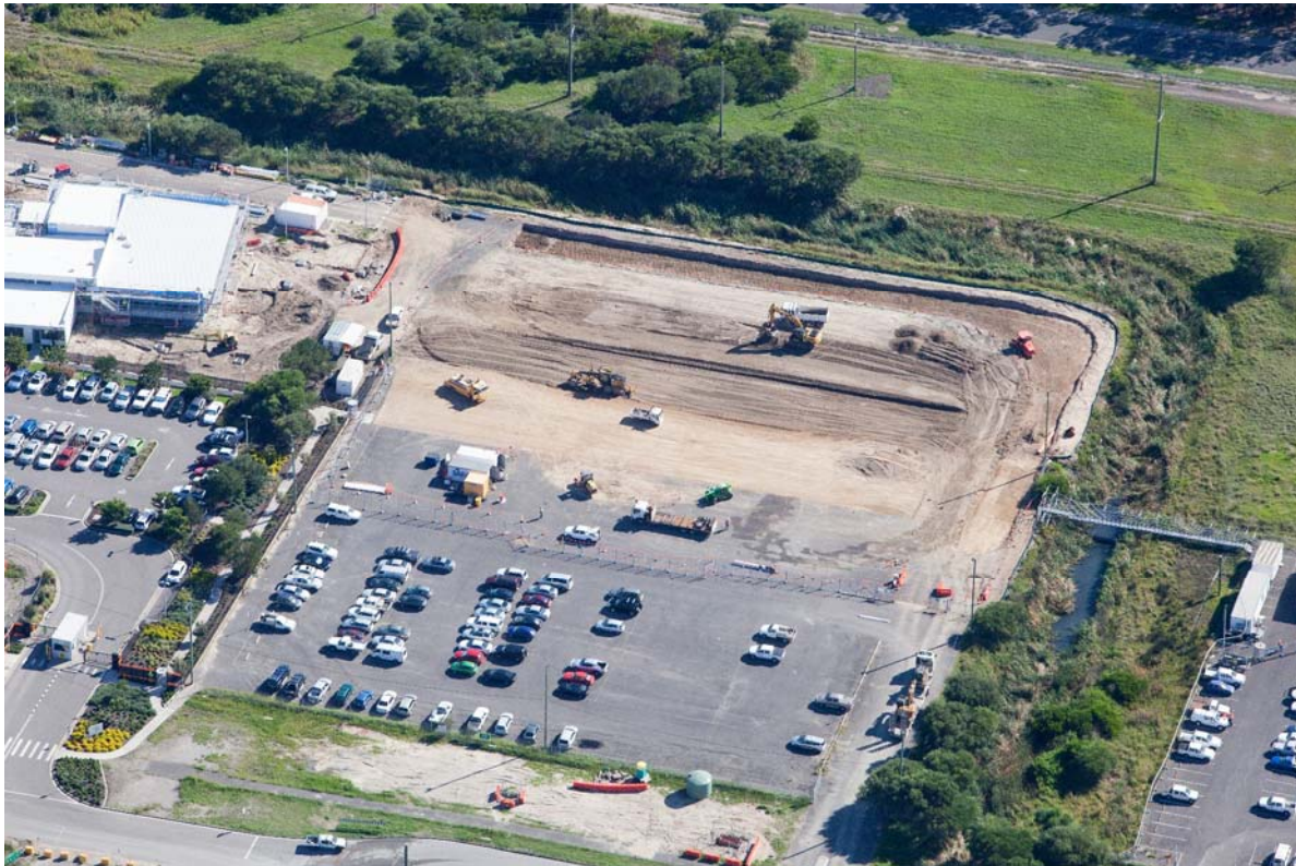
Figure 13: Construction of new Stores Building
