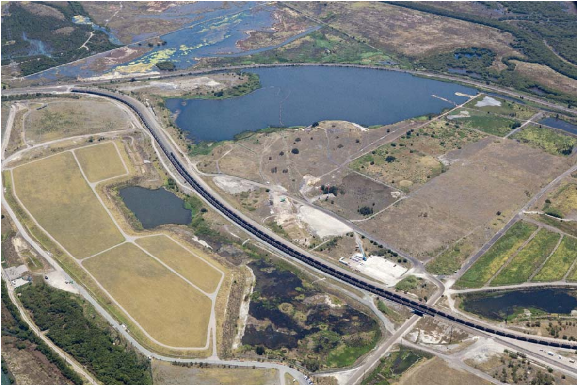
Figure 7: Commencement of Rail Flyover construction, including site compound.
