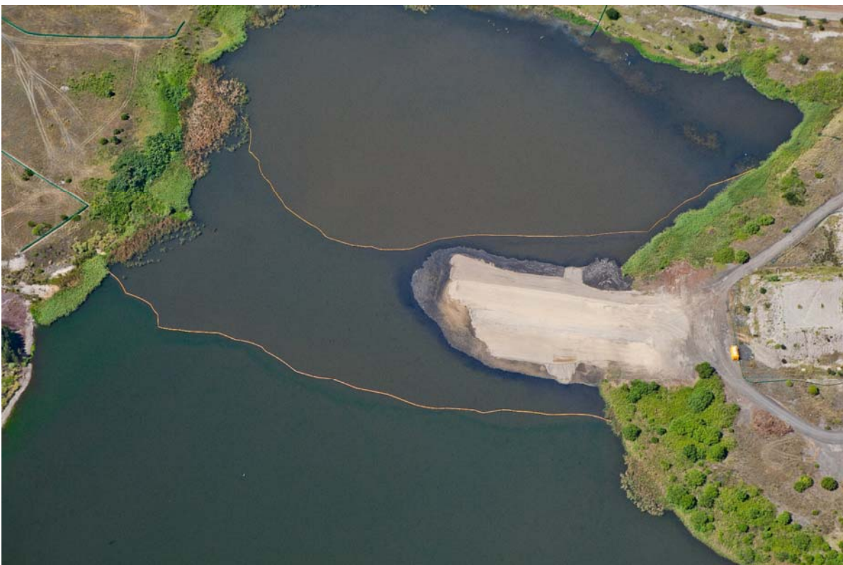
Figure 8: Commencement of Rail Flyover Embankment (western end).
