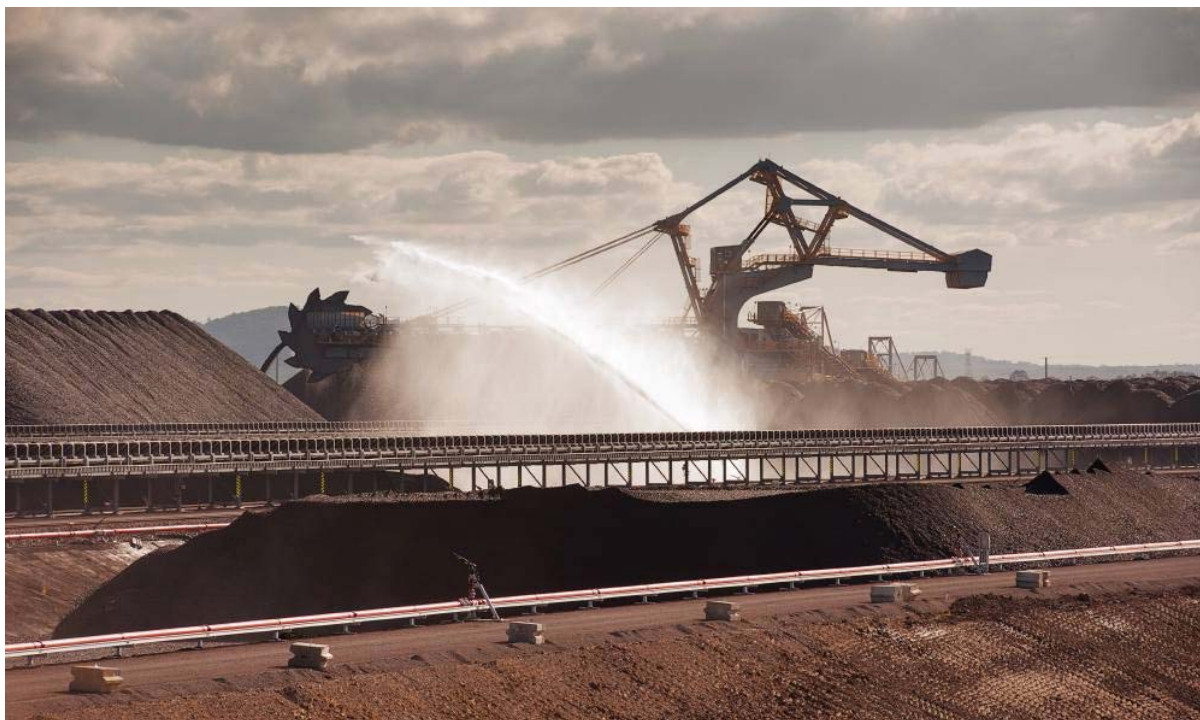
Figure 14: NCIG Dust Suppression System in operation.
