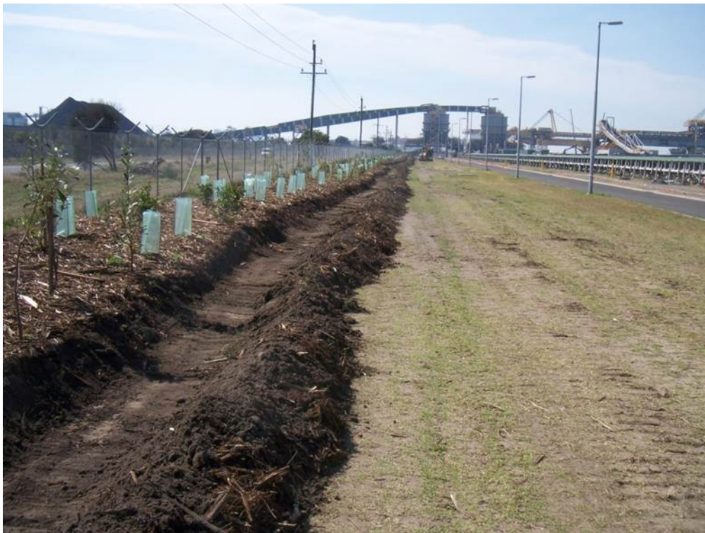
Figure 12: Landscaping and construction of irrigation
