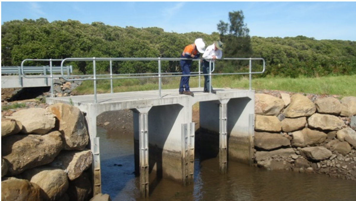
Figure 36: Creek 5 Drop board support structure prior to fitting of drop boards
