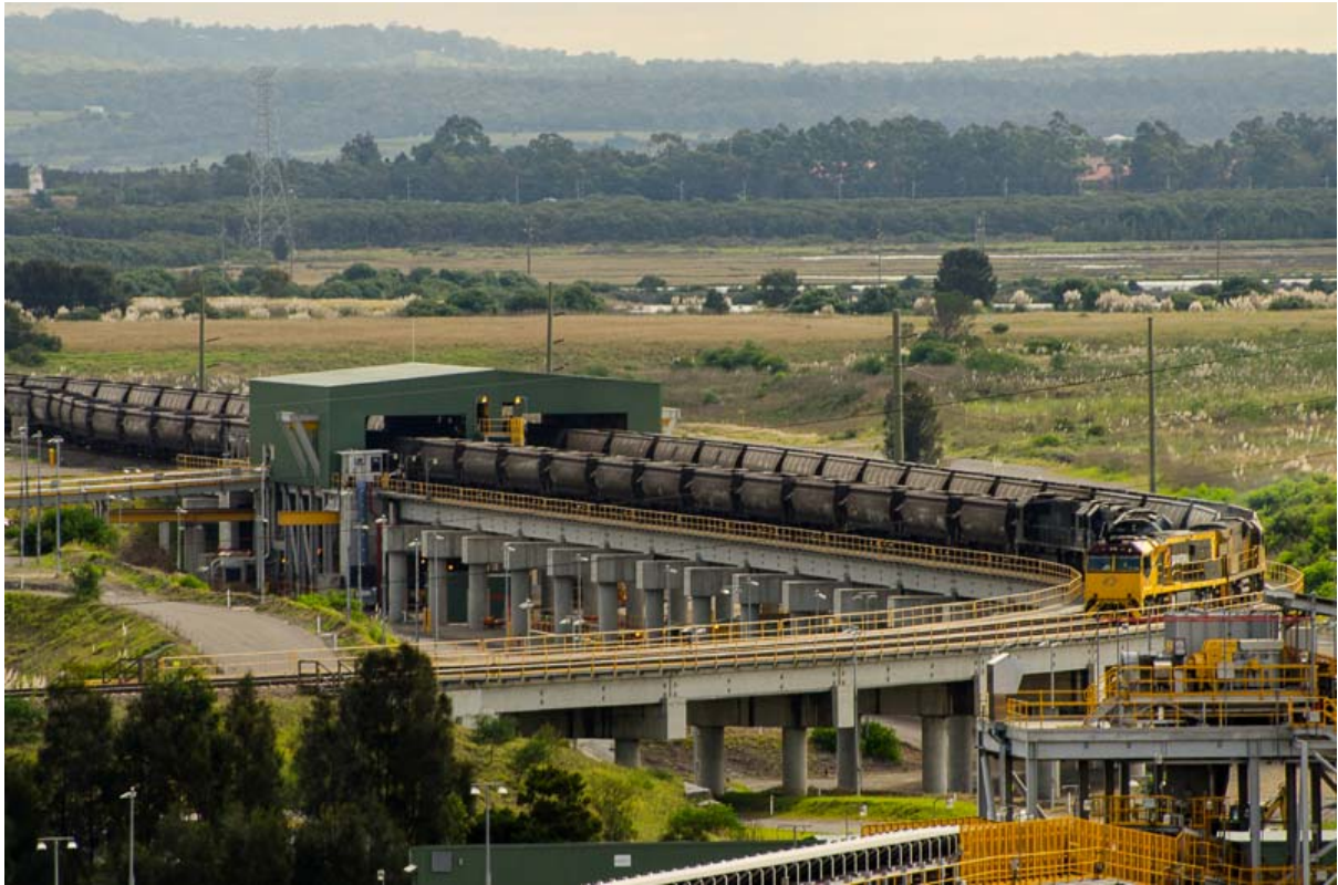
Figure 16: First train delivery stacked to Stacker Reclaimer 4.
