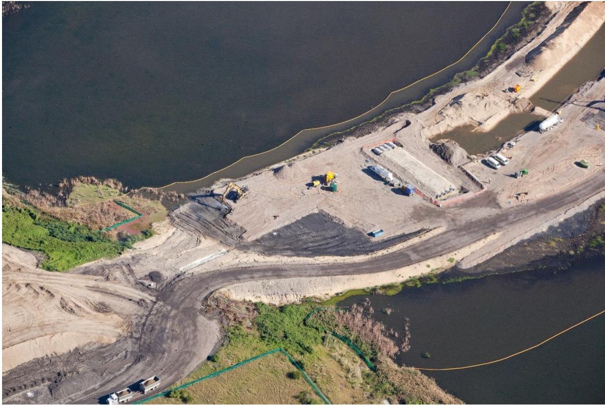
Figure 15: Rail Flyover Construction, including Ground Improvement works
