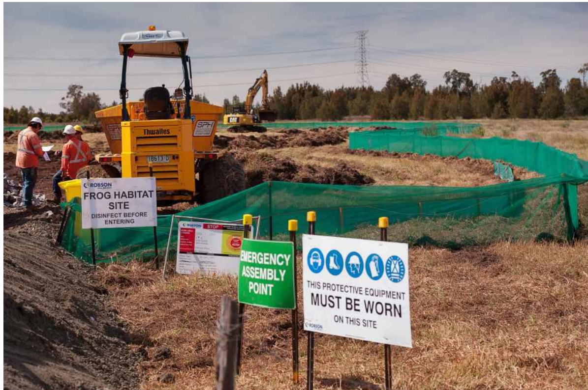
Figure 39: Construction at new CHEMP site, Ash Island
