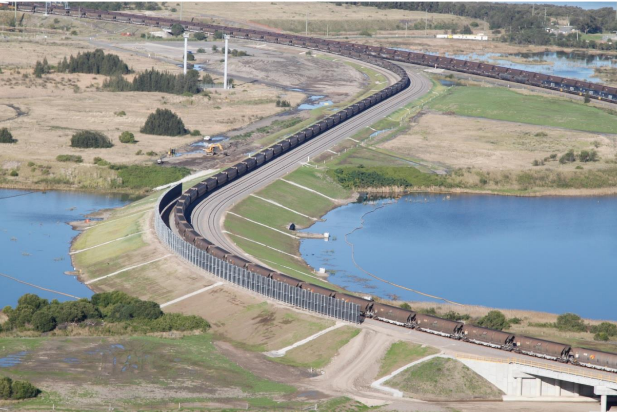
Figure 9: Completed Screen to mitigate train light impacts on birds using Deep Pond
