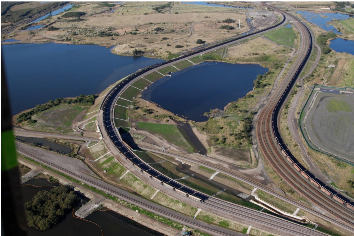
Figure 5: Rail Flyover in Operation, June 2015
