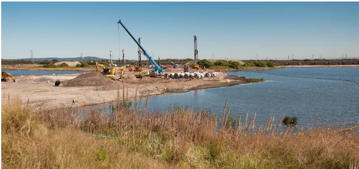
Figure 18: Rail Flyover Construction
