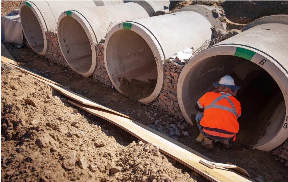
Figure 17: Rail Flyover Construction - Culvert Installation
