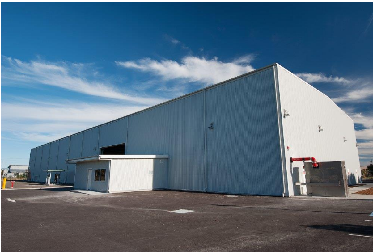
Figure 11: New Stores Building Exterior
