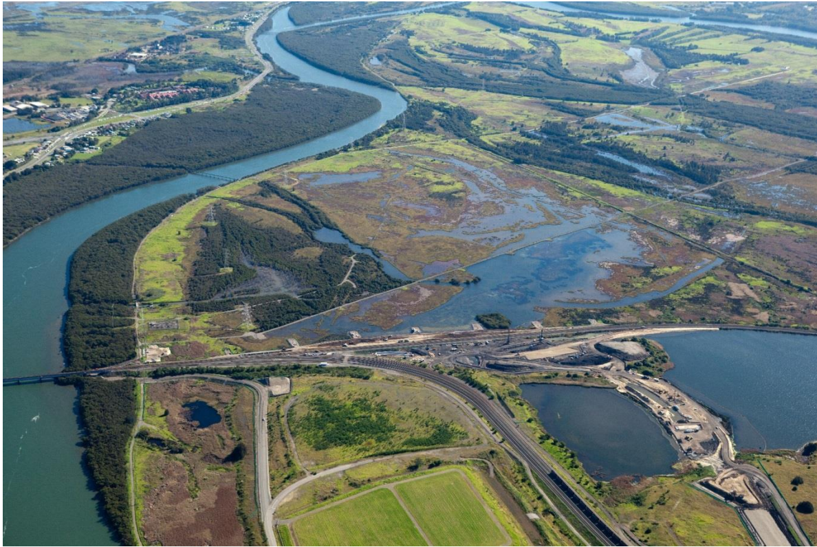
Figure 19: Western Deviation and Flyover Construction
