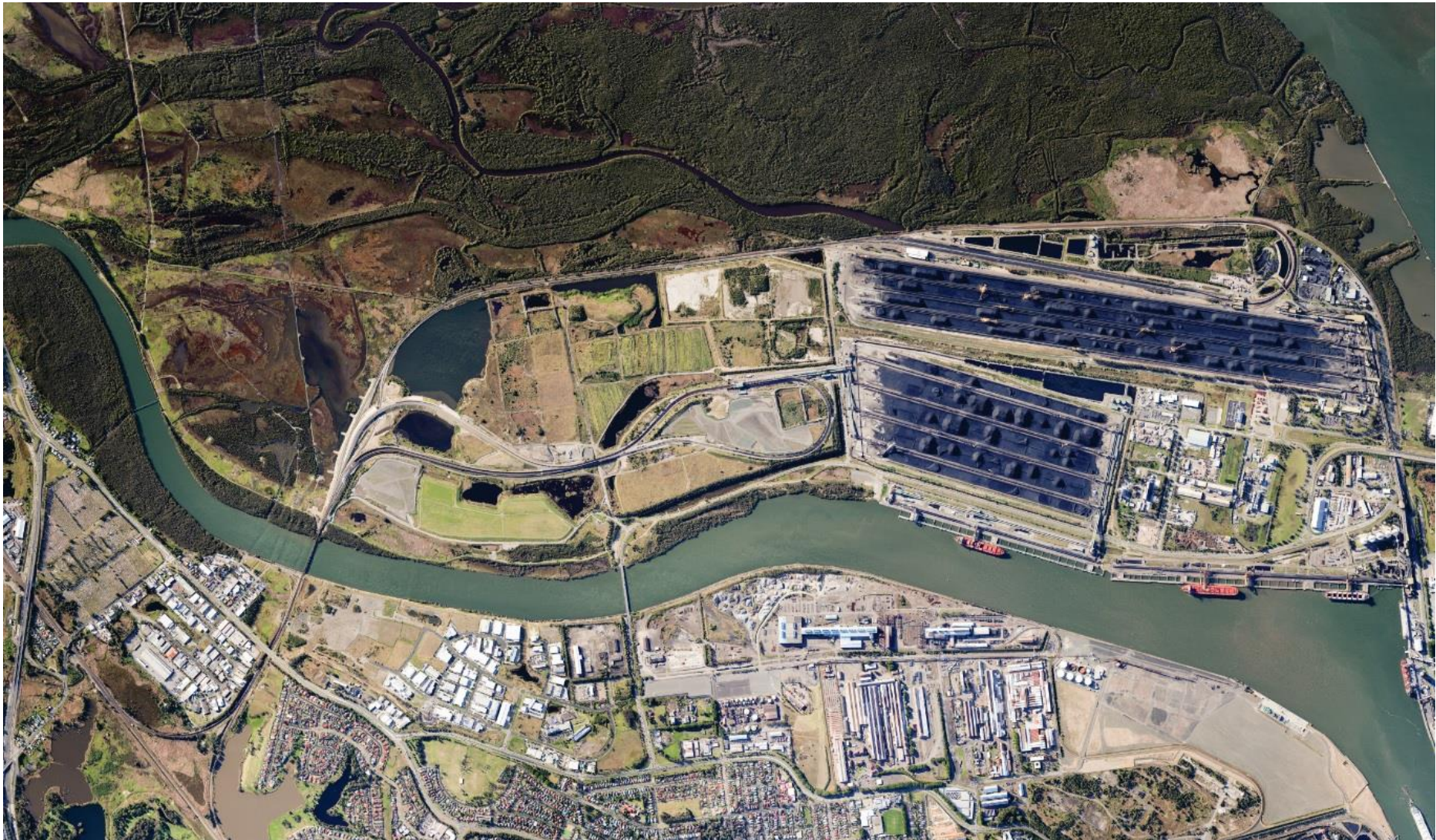
Figure 22: May 2015 Aerial Photograph of Project
