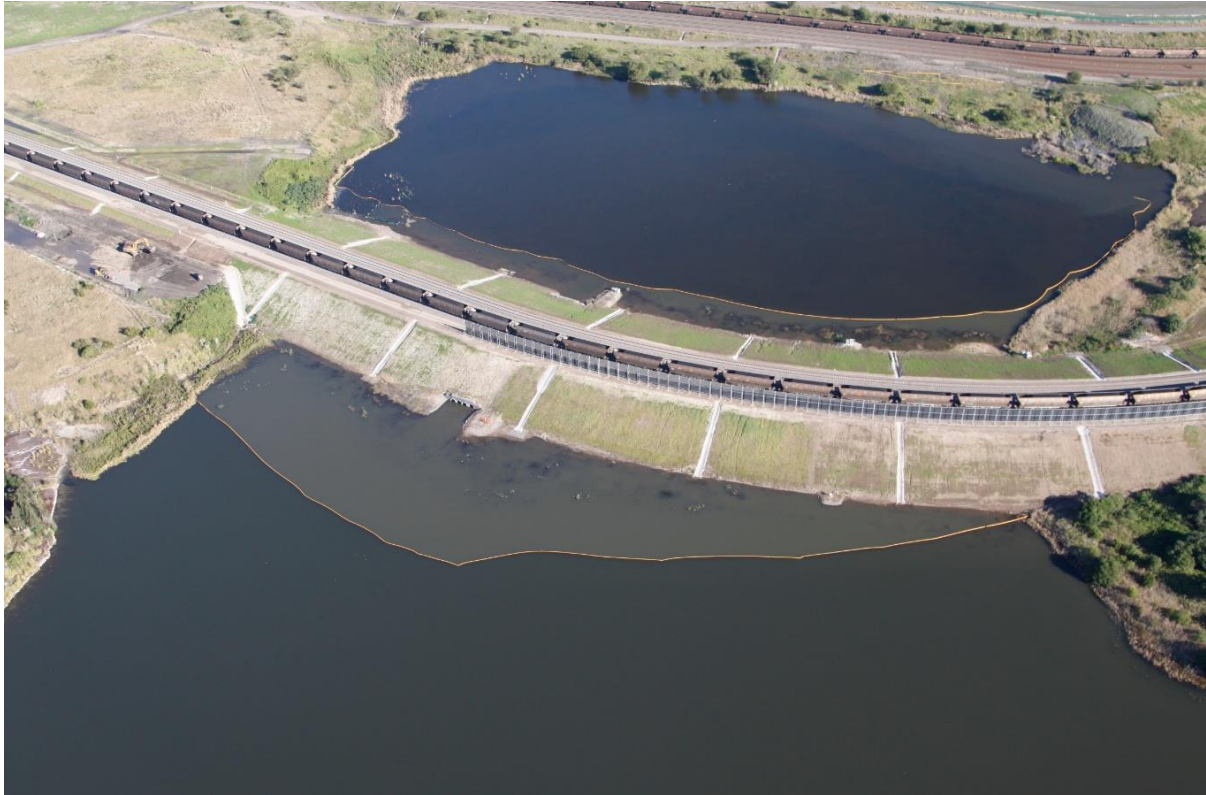
Figure 14: Rail Flyover Construction - Sediment and Erosion Control
