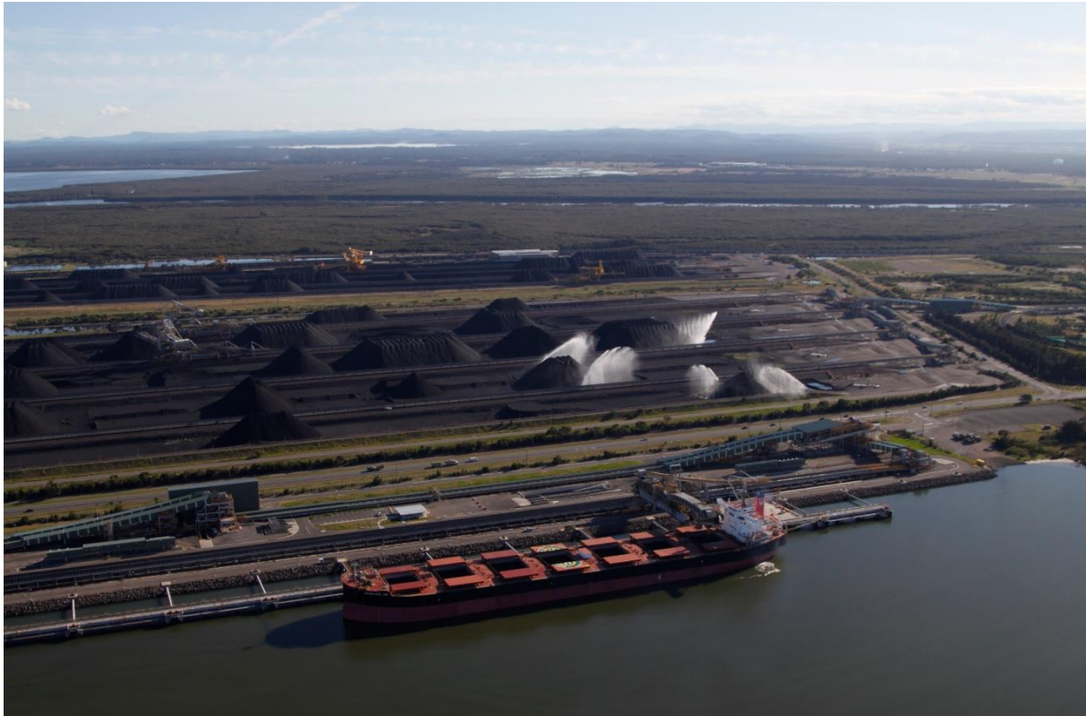
Figure 6: Stockyard with Dust Suppression System
