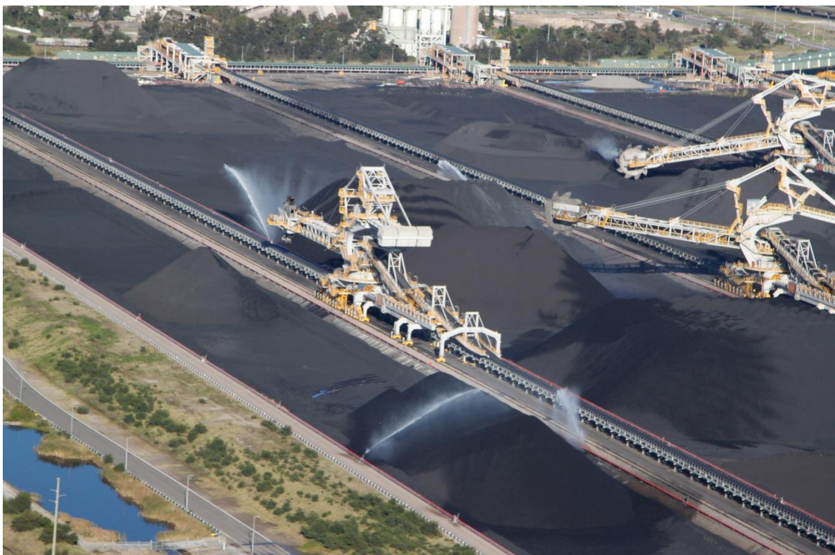
Figure 7: Stockyard with Stacker Reclaimers in Operation
