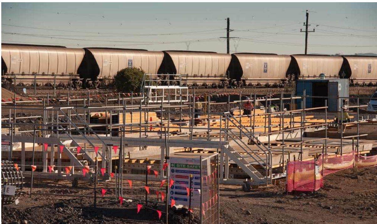
Figure 16: Rail Flyover Foundation Construction
