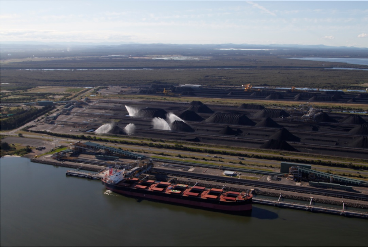
Photo 2-2: NCIG Site Overview Facing North
