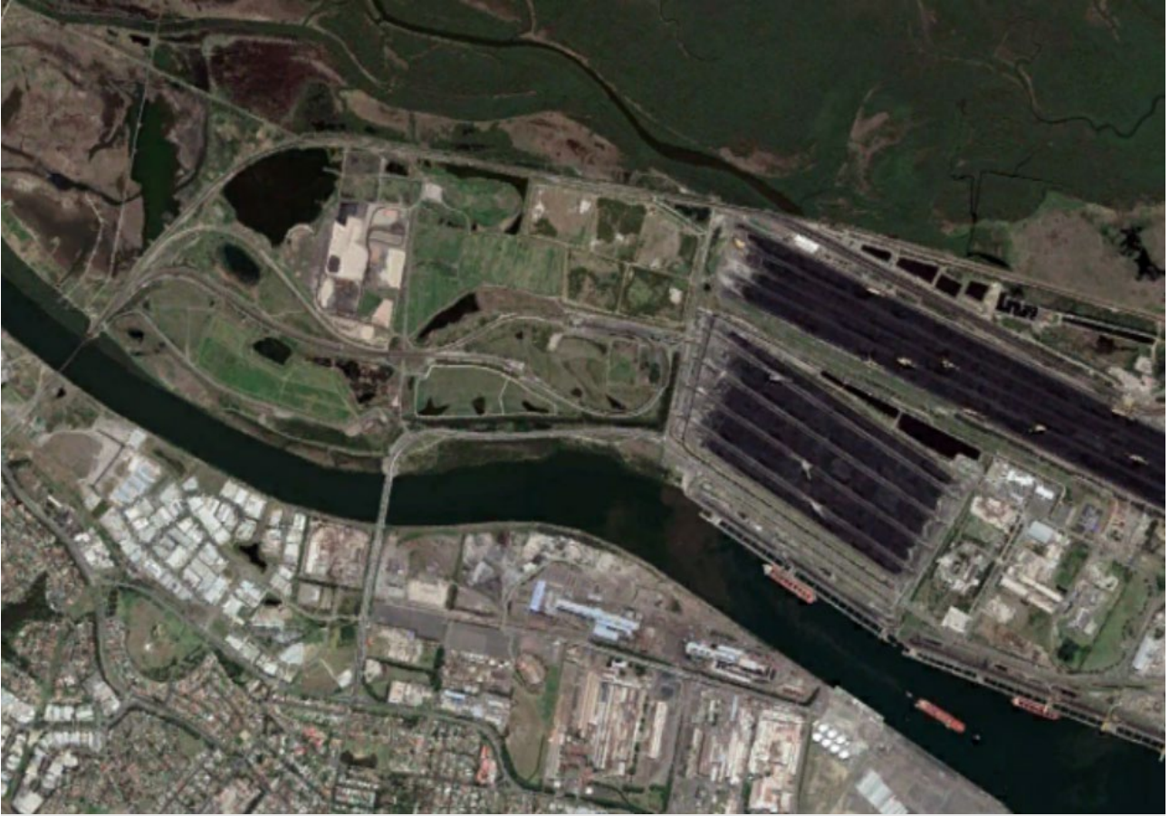
Photo 2-4: Aerial Photograph of NCIG Terminal (October 2019)
