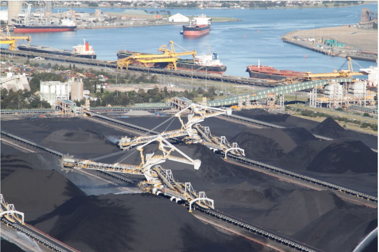
Photo 2-3: Stockyard with Stacker Reclaimers in Operation
