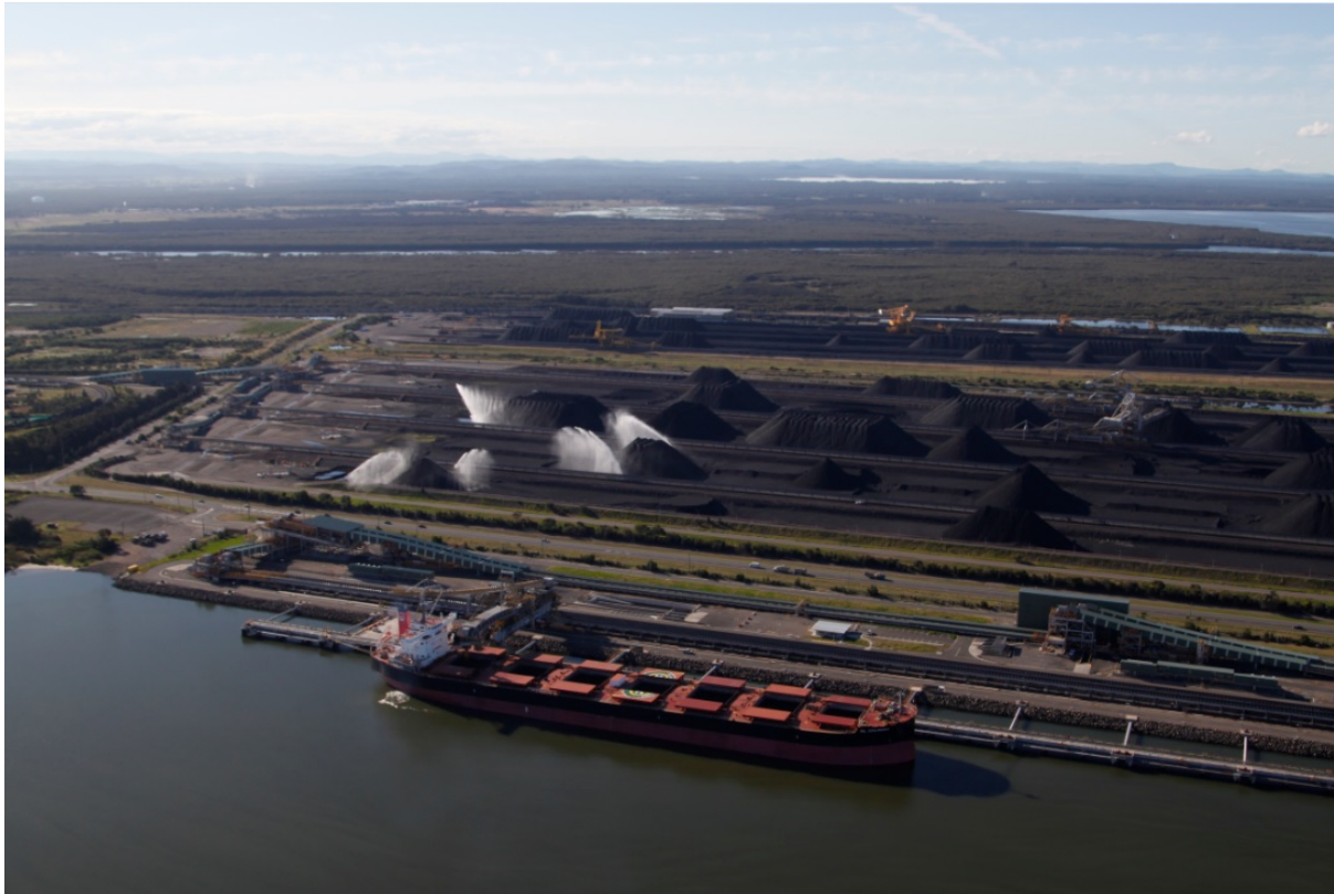
Figure 4: NCIG Site Overview Facing North
