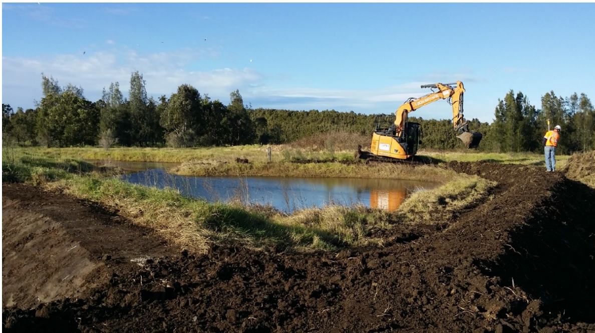
Figure 26: Creation of bunds around Stage 7 to control Gambusia
