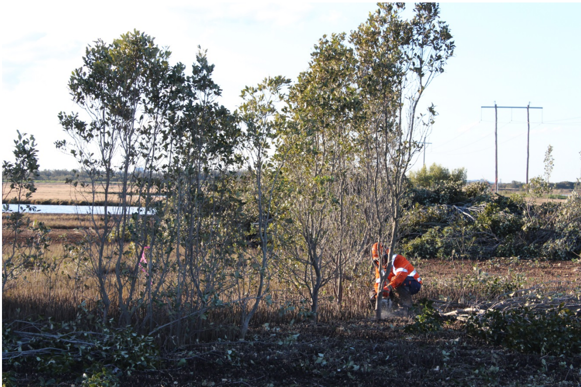
Plate 11: Chainsaw being used for Phase 1 clearing
