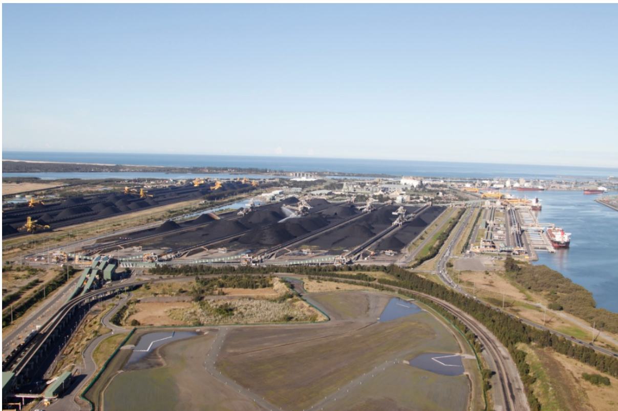
Figure 3: NCIG Site Overview Facing East
