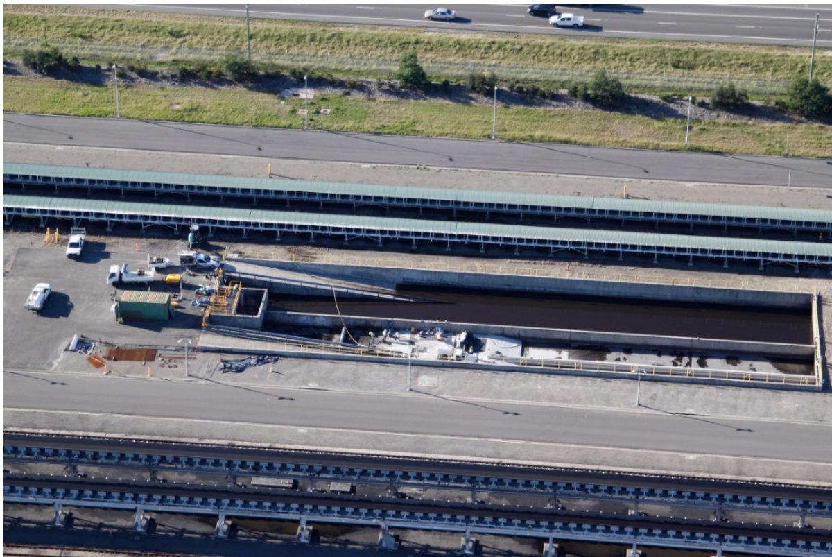
Figure 20: Modifications to Wharf Settling Basin 1
