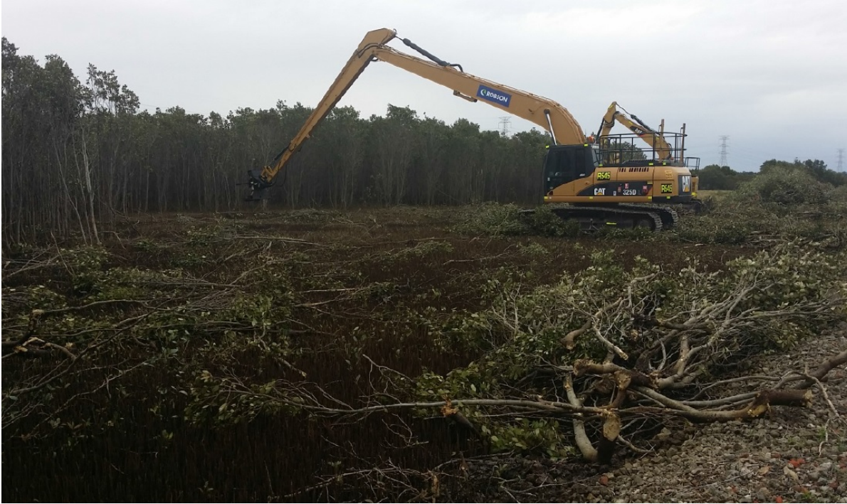
Figure 28: Long reach excavator removing mangroves with hydraulic shear
