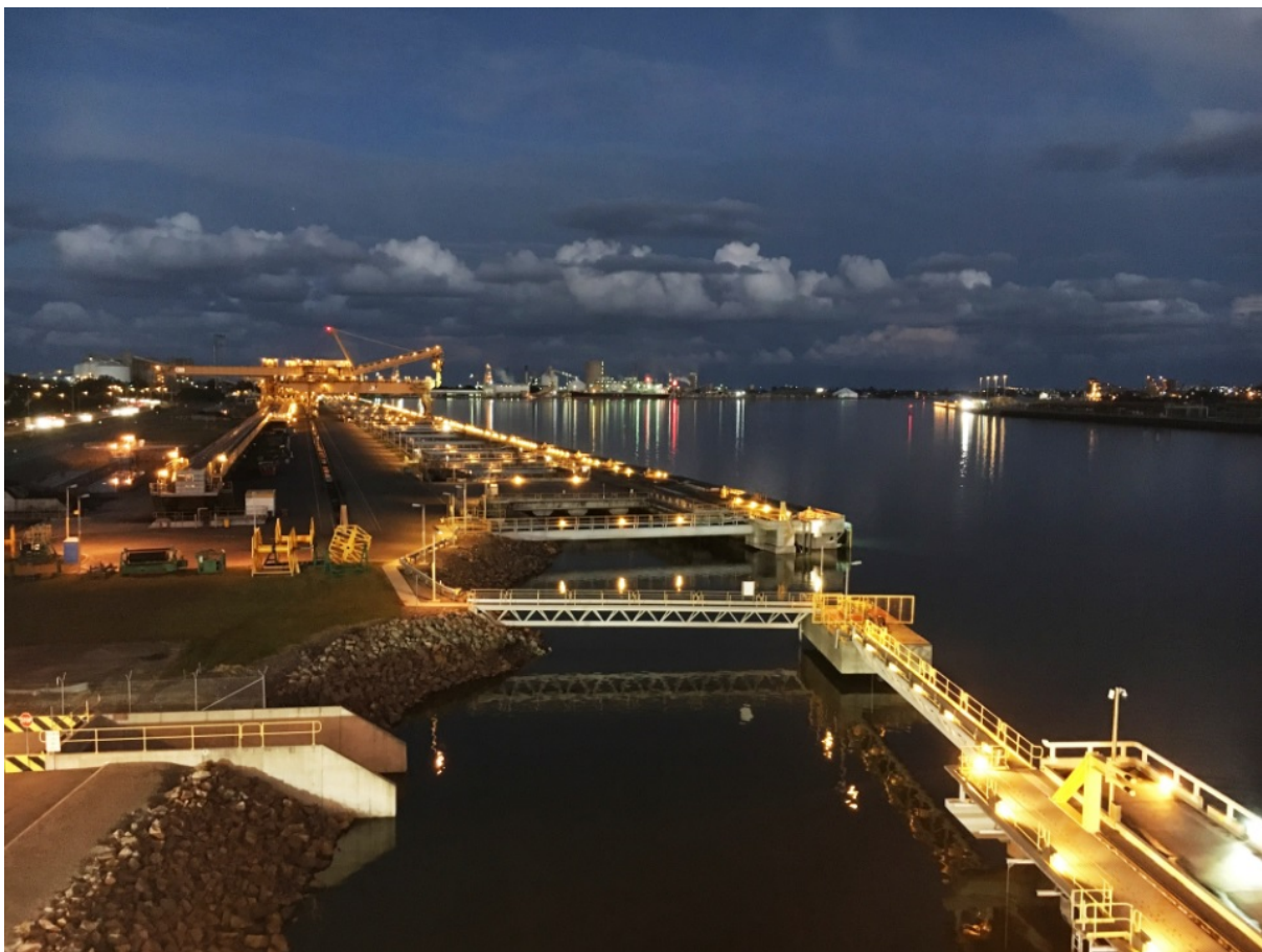
Figure 5: NCIG Site Overview at Night
