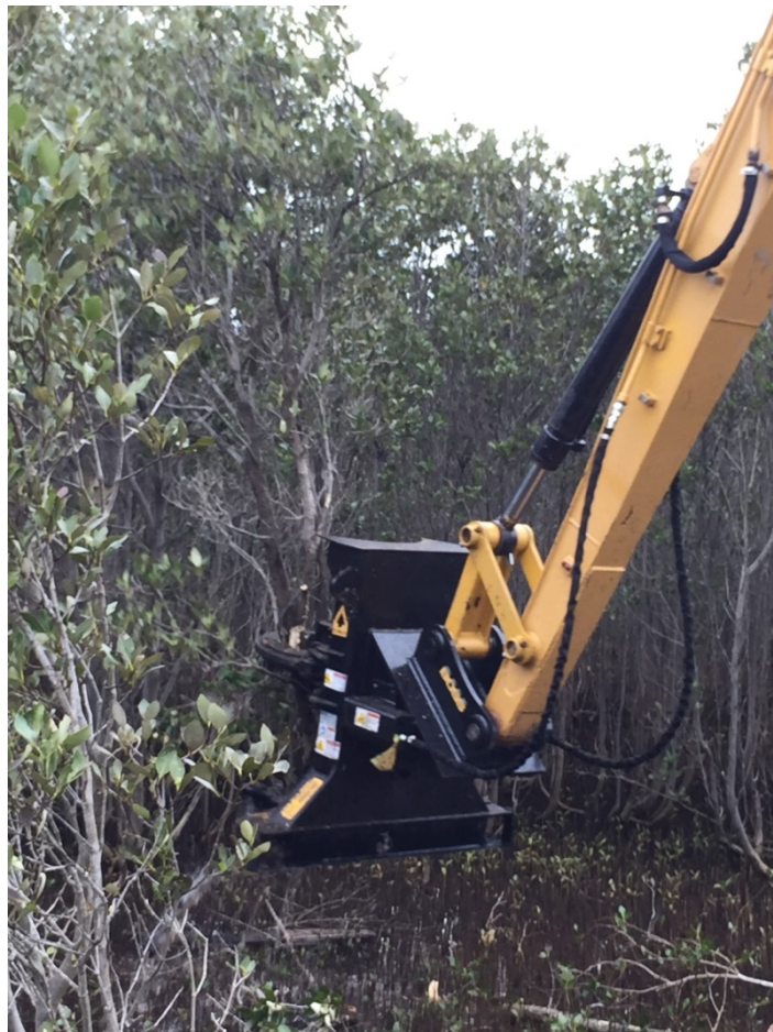
Plate 4: Hydraulic shear attachment removing mangroves
