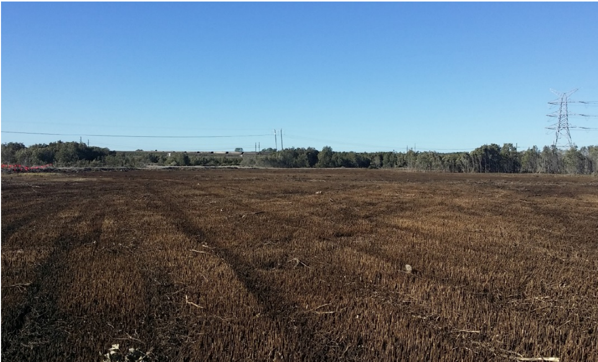
Figure 29: Completed Phase 2 clearing area
