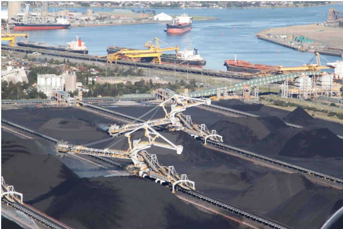
Figure 7: Stockyard with Stacker Reclaimers in Operation
