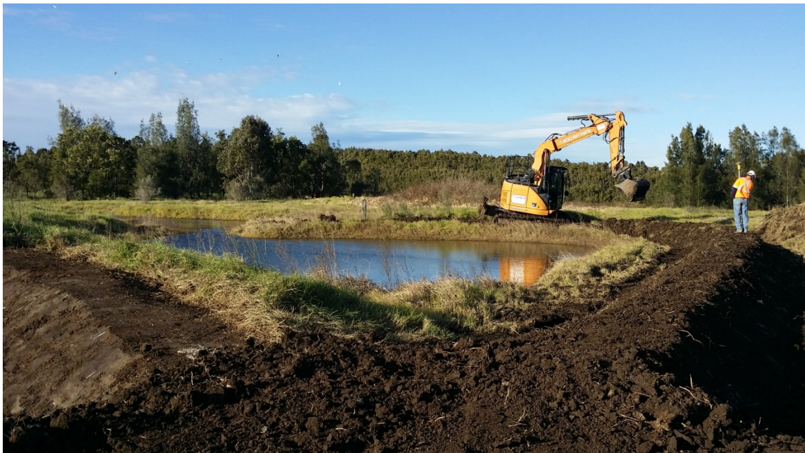
Plate 1: Creation of Bunds around Stage 7 Ponds to control Gambusia
