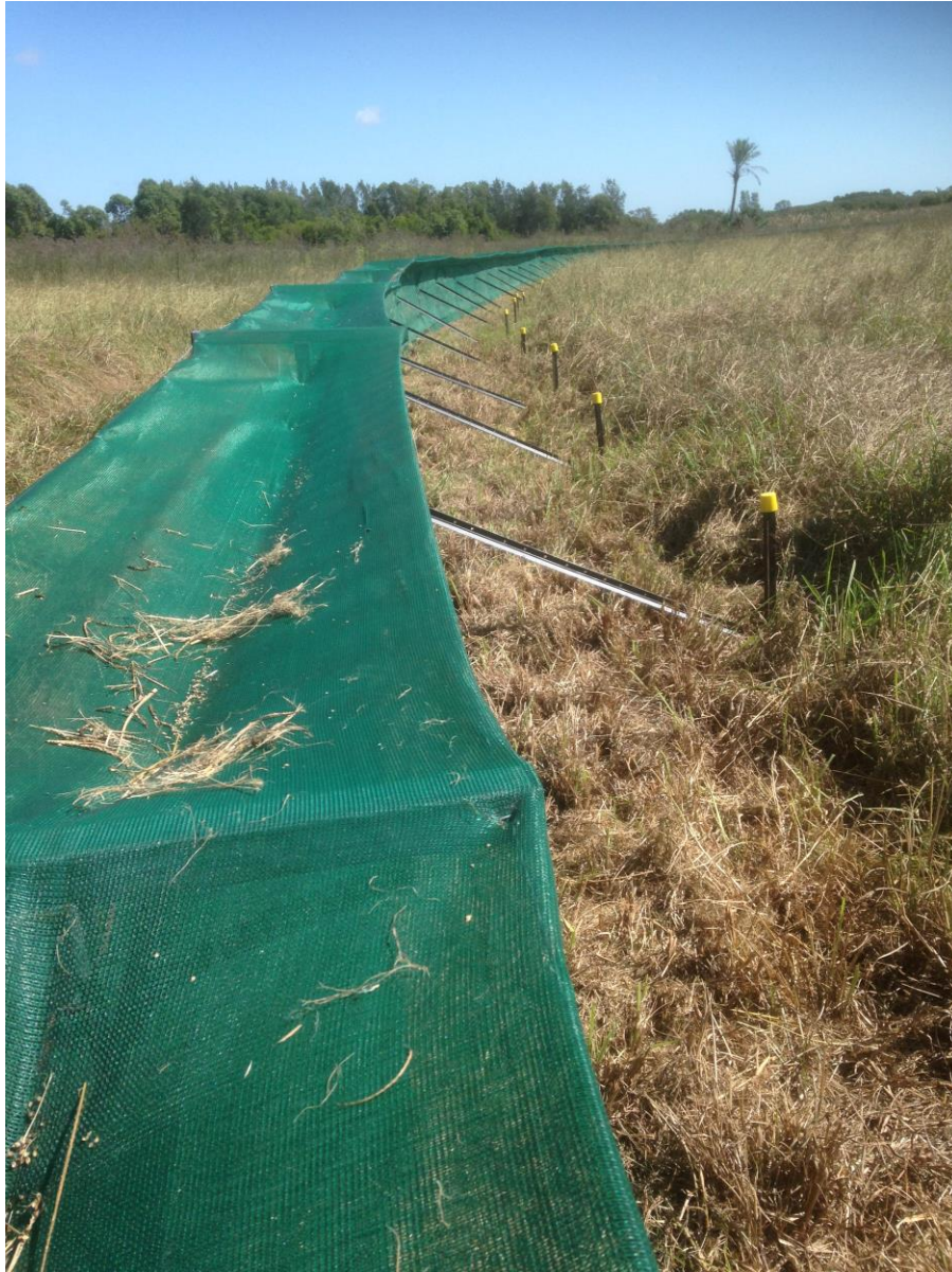
Fence repairs and slashing
