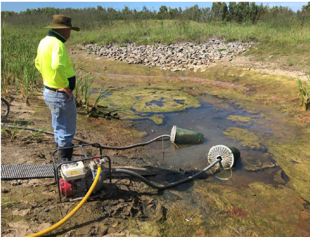
Plate 4: Pond dewatering setup (with screen on inlet)
