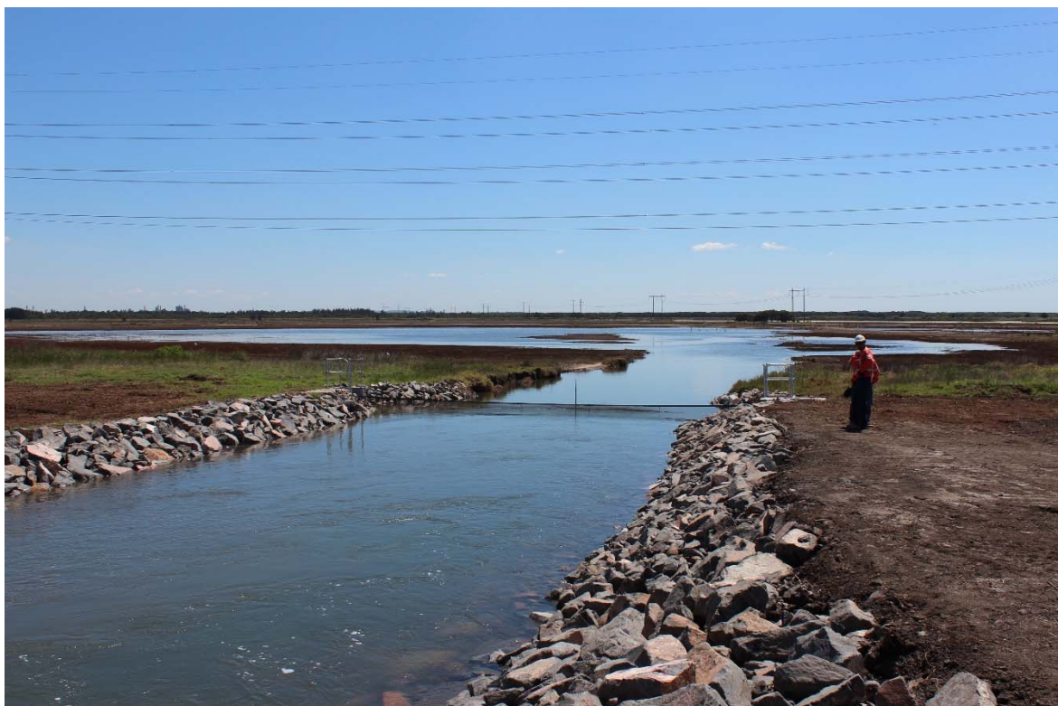
Figure 23: Rock protection along Fish Fry Creek.
