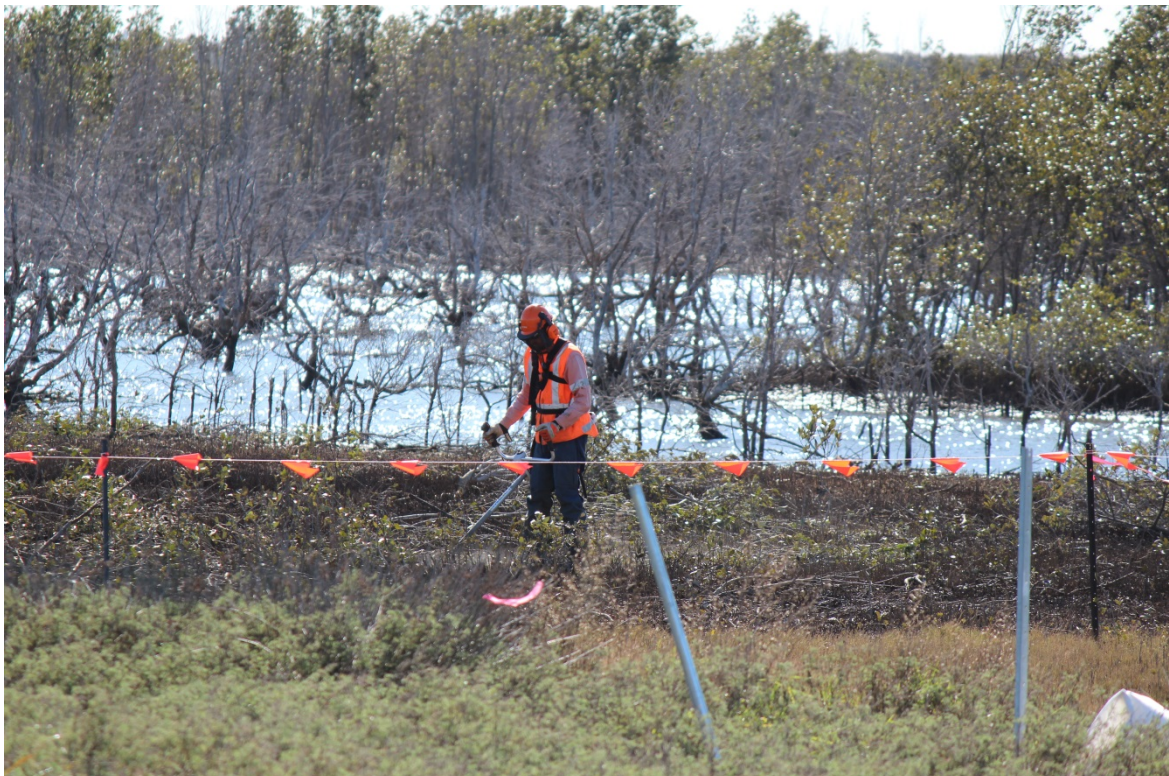
Plate 10: Forestry saw being used for Phase 2 clearing
