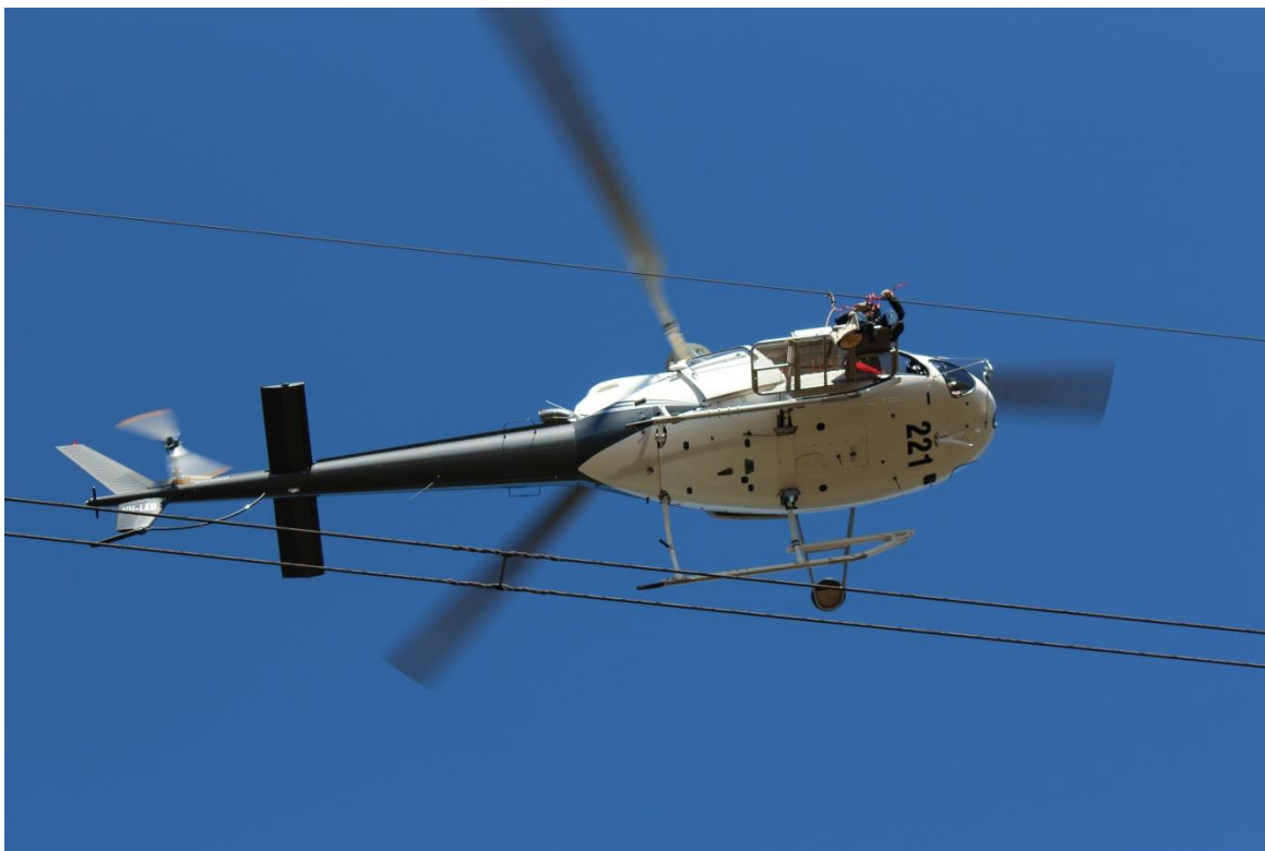
Plate 24: Intallation of Transgrid bird diverters
