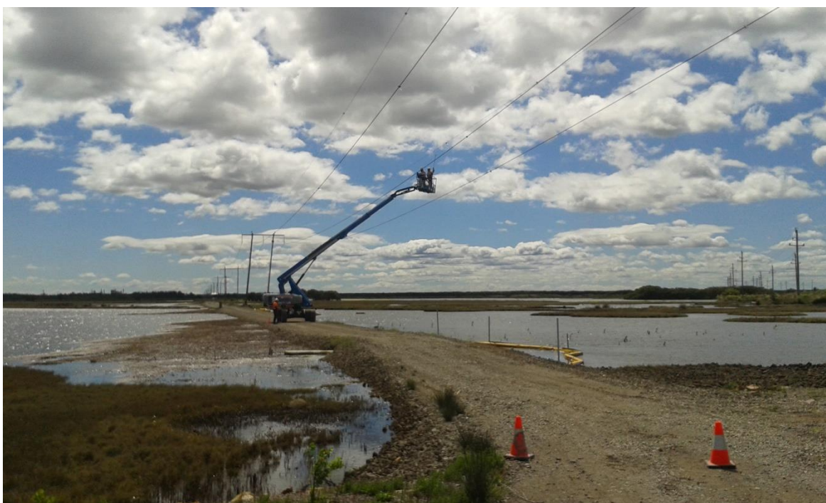
Plate 23: Intallation of Ausgrid bird diverters
