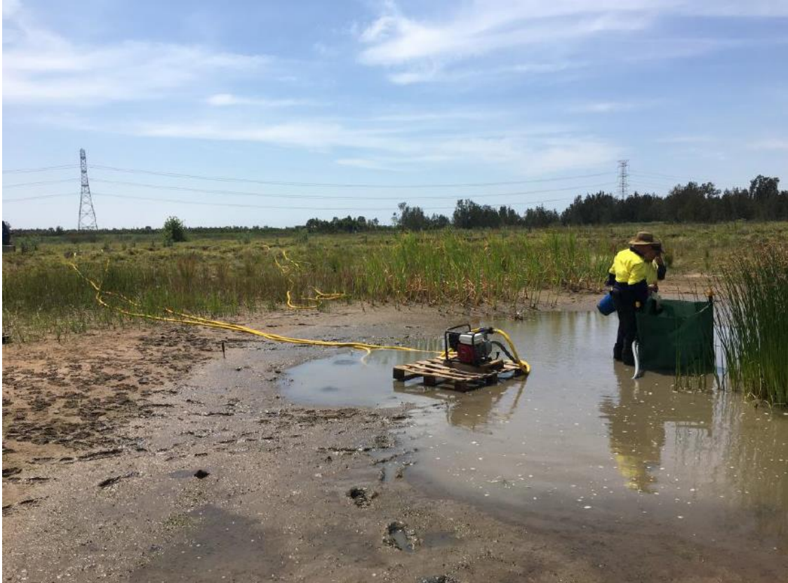
Plate 1: Pond dewatering setup (Pond 16)
