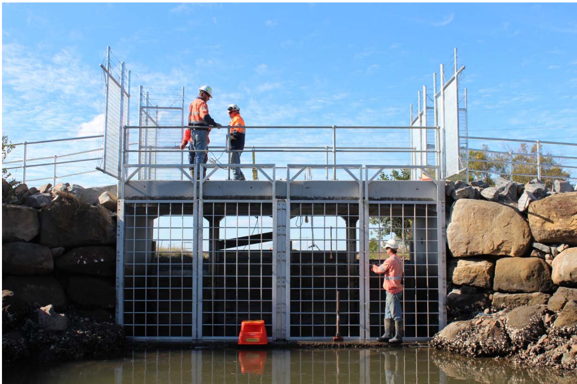
Figure 21: MPED 2 screen installed at Fish Fry Creek.
