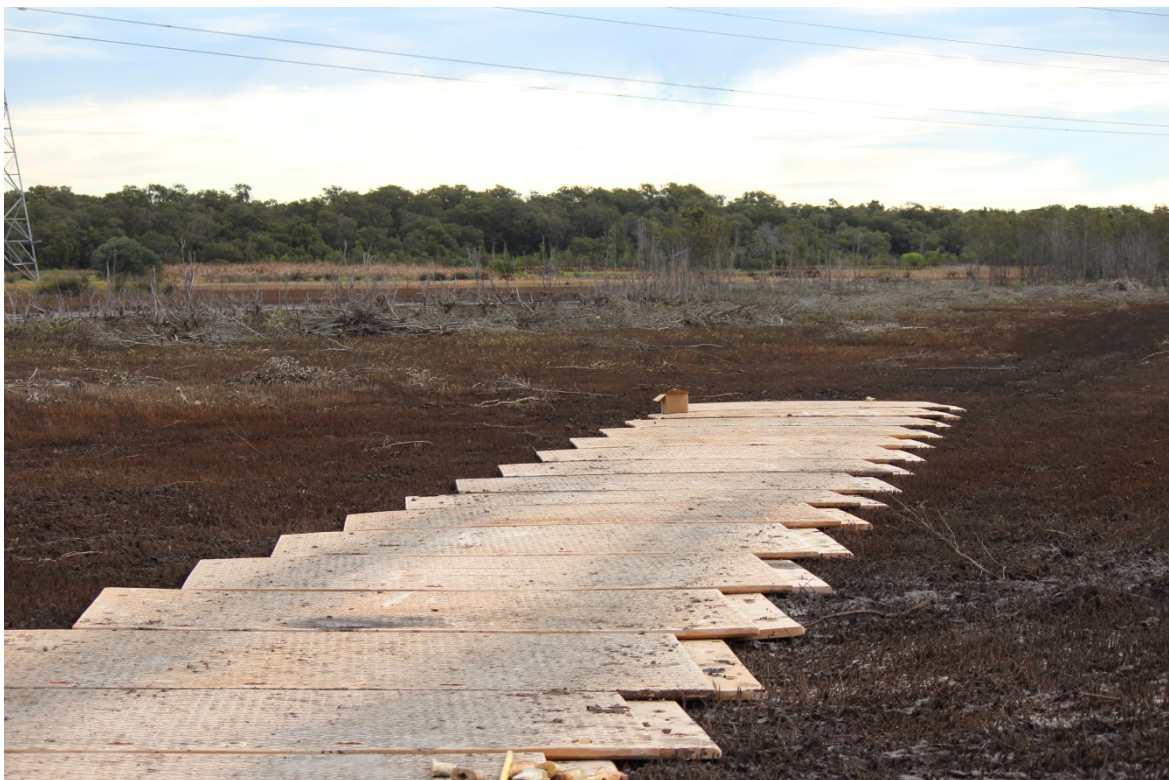
Plate 12: "Bog mats" used by trucks for accessing felled trees
