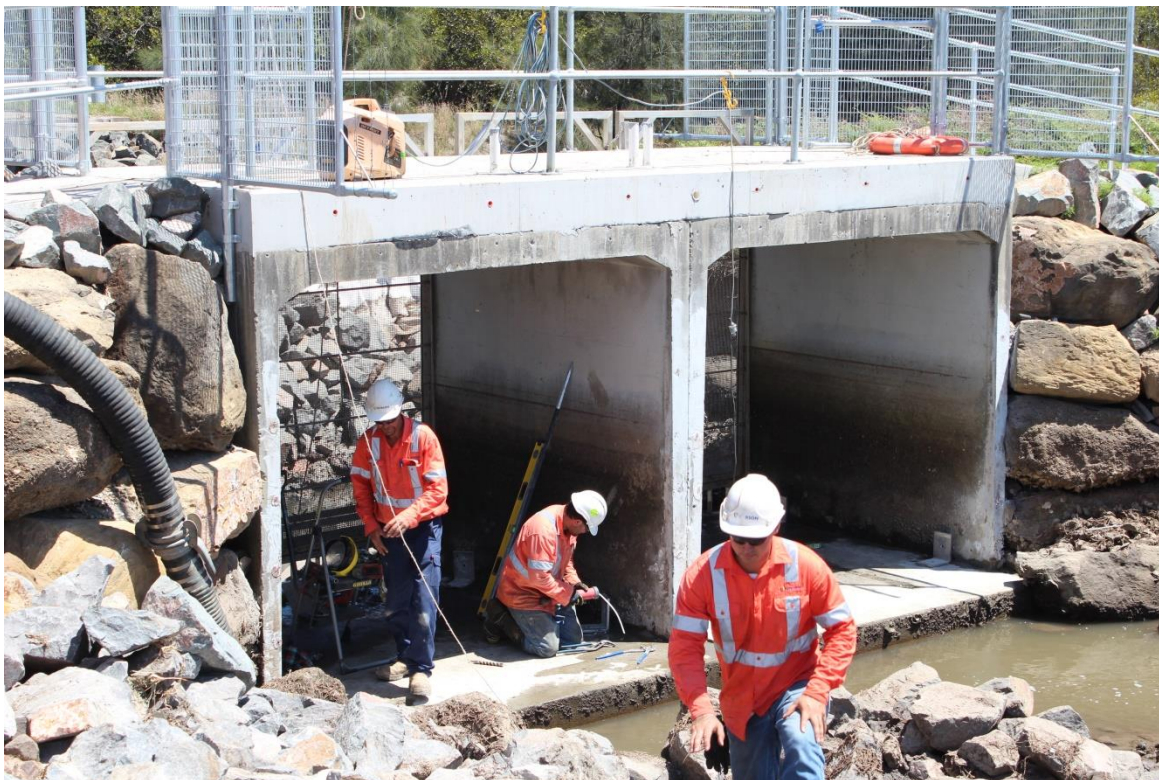
Plate 25: Preparation for installation of Smart Gate
