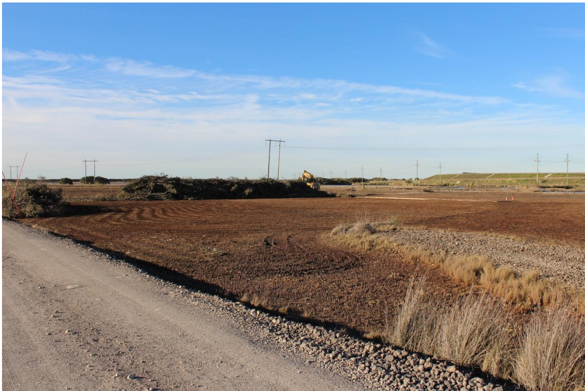
Plate 4: Completed phase 2 clearance
