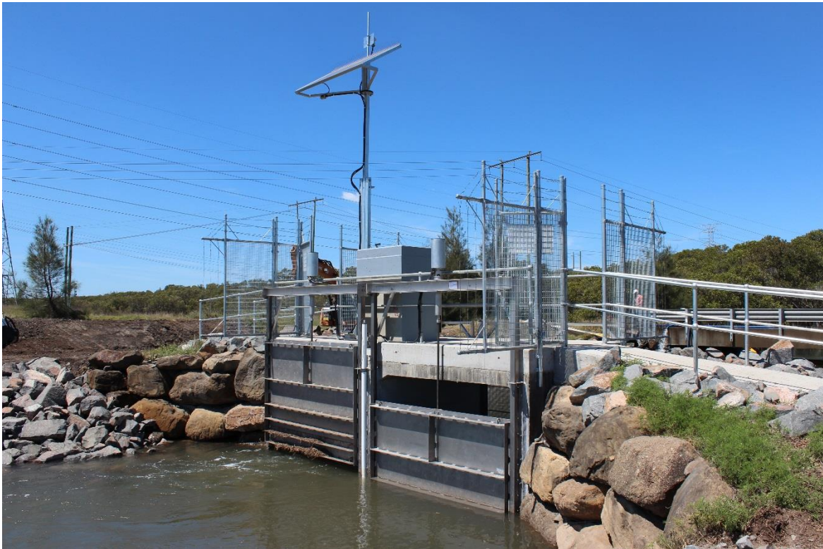
Plate 28: Completed Smart Gate installation, Fish Fry Creek
