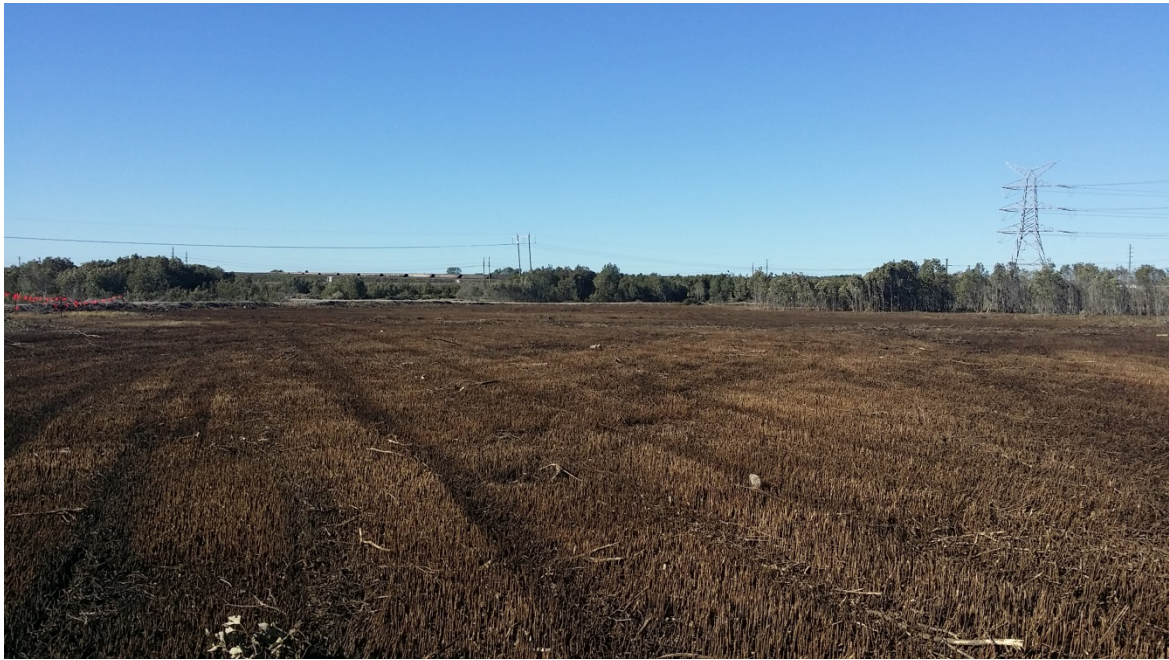
Plate 7: Completed Phase 2 clearing area
