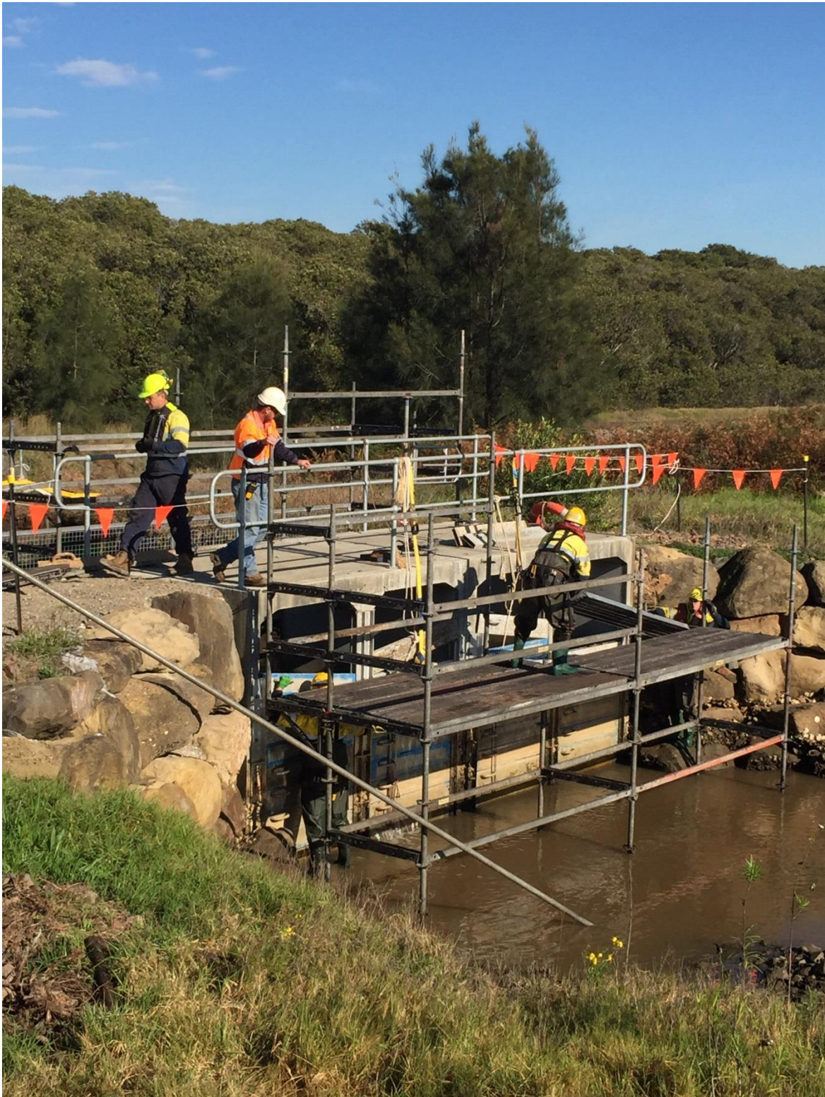
Plate 13: Preparation of Fish Fry Creek culvert
