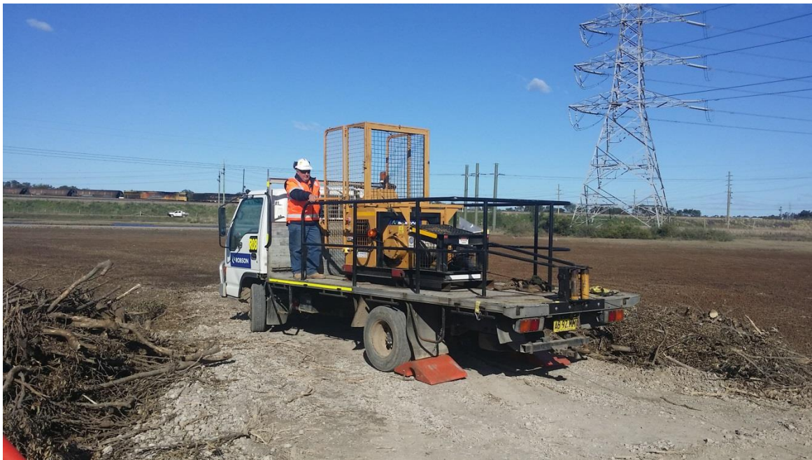
Plate 7: Retrieval of felled mangroves using winch
