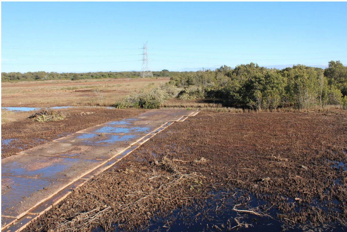
Plate 5: Dura-mat use to remove felled mangroves
