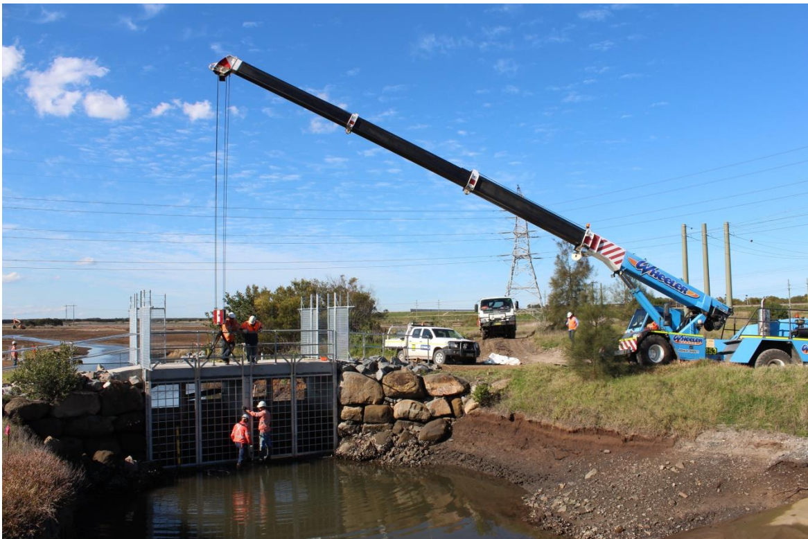
Plate 17: Installation of MPED 2 screens
