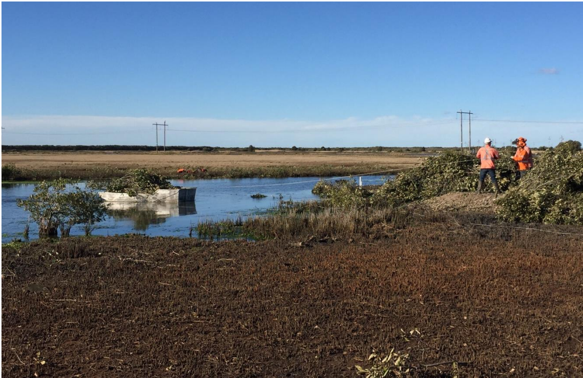
Plate 11: Removal of felled mangroves with boat
