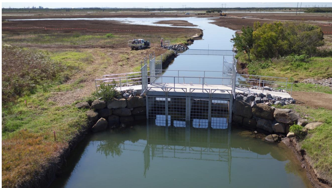
Plate 21: Completed MPED 1 and MPED 2 instal
