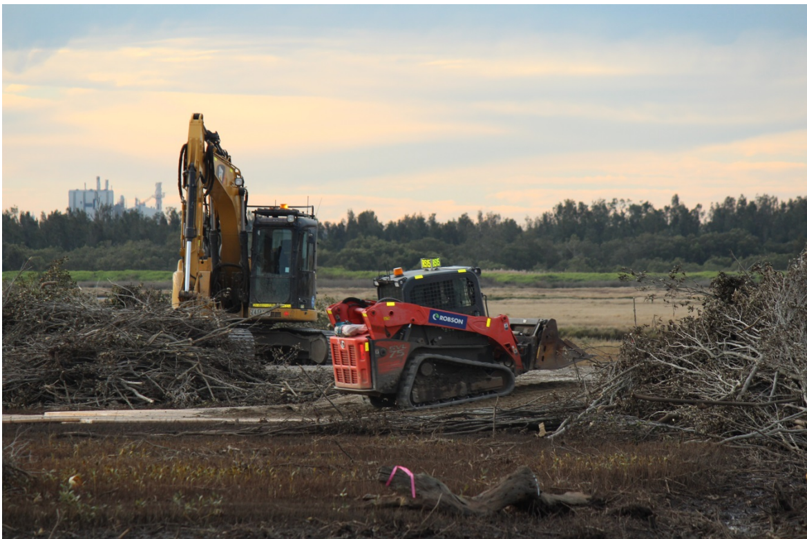
Plate 19: Excavator and positrack removing felled mangroves
