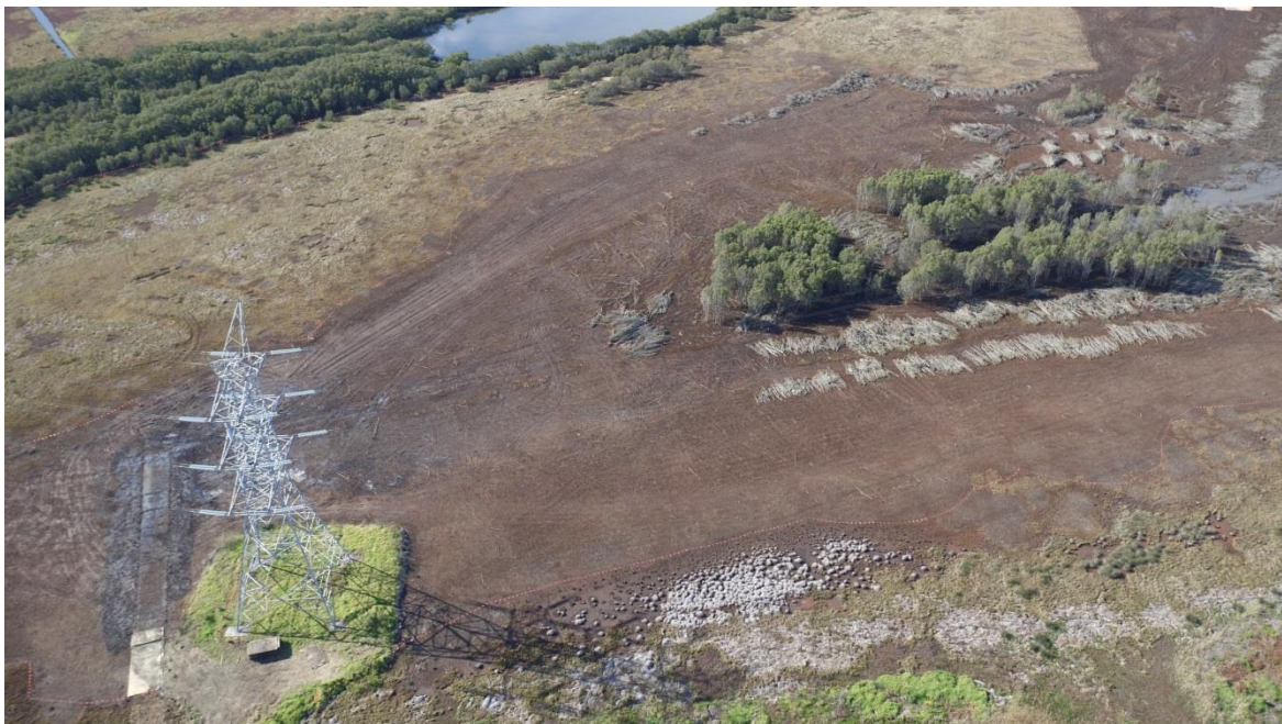
Plate 2: Progressive mangrove removal, Area E
