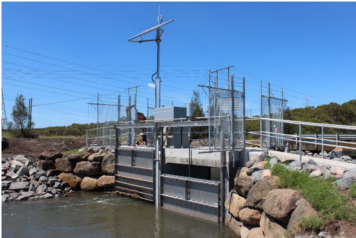
Figure 22: Completed Smart Gate at Fish Fry Creek.
