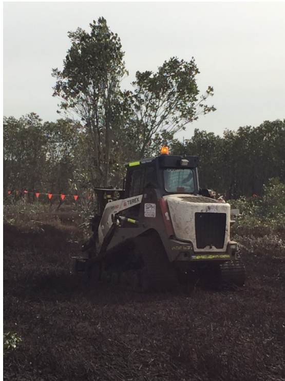
Plate 5: Positrack removing mangroves with hydraulic shear
