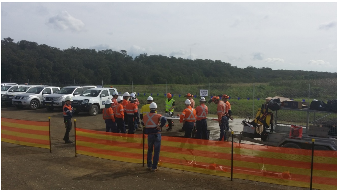
Plate 2: Competency training for manual removal crews
