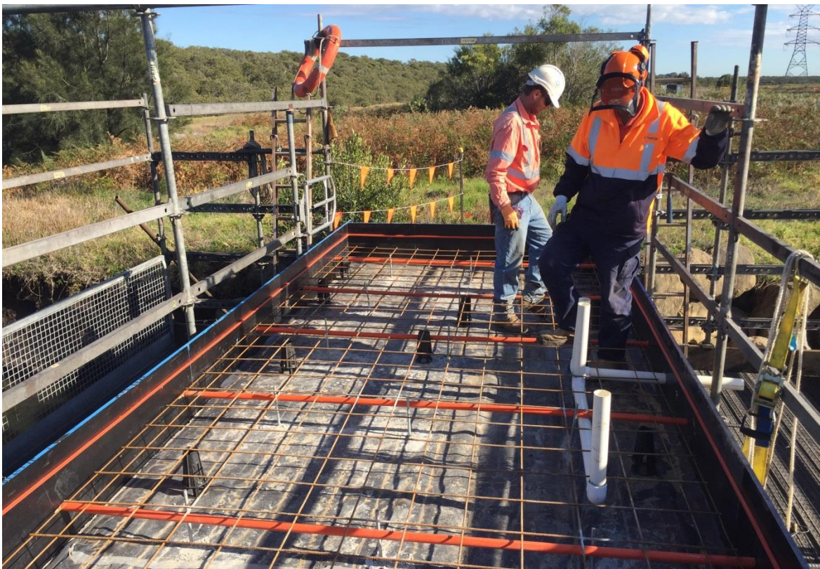
Plate 12: Surcharge concrete loading of Fish Fry Creek culvert
