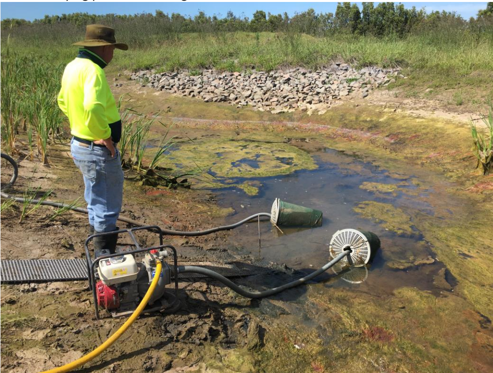
Pond 8 dewatering setup
