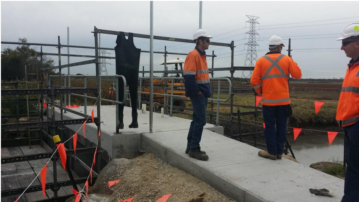
Plate 16: Completed surcharge loading and concrete path to Fish Fry Creek culvert
