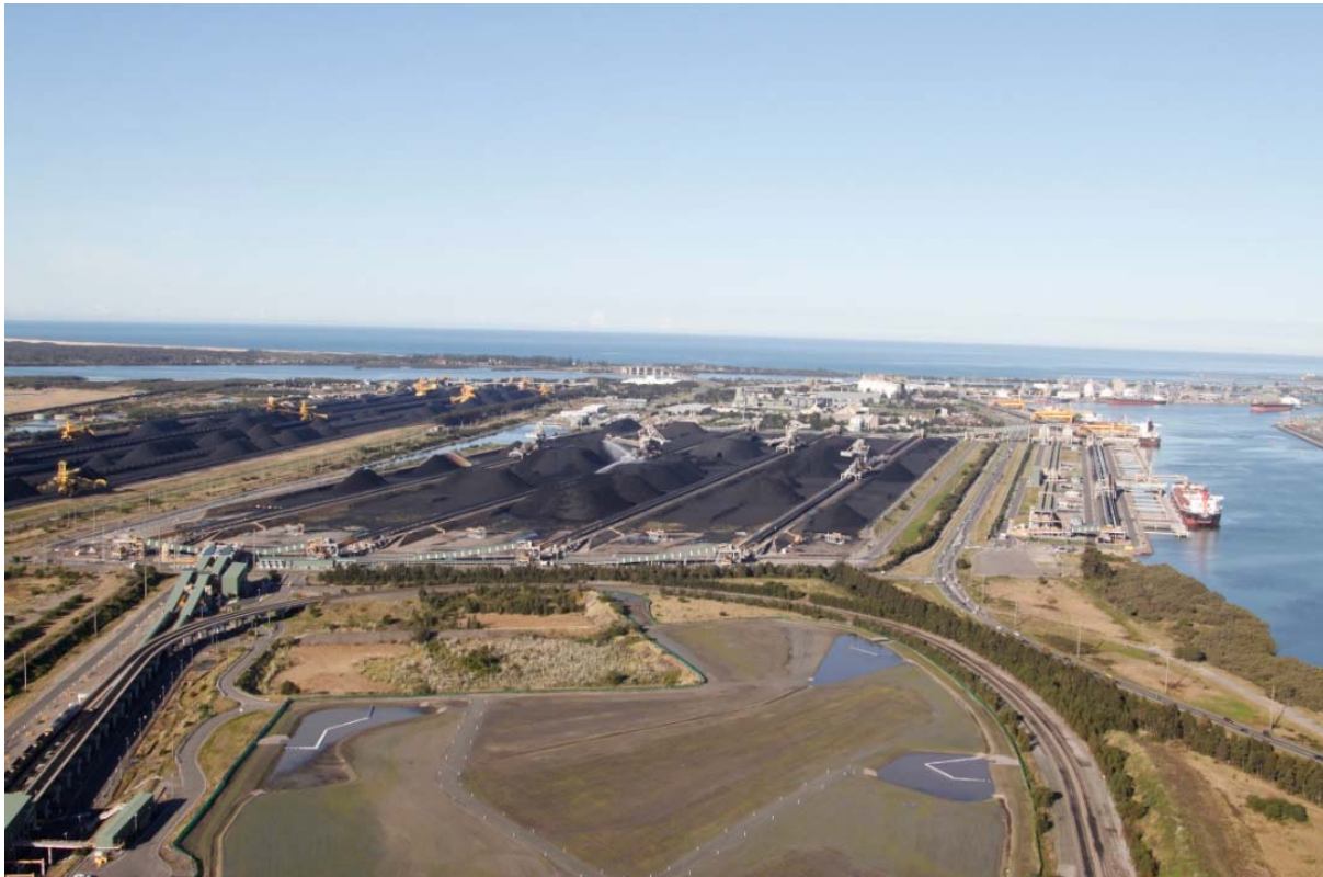
Figure 3: NCIG Site Overview Facing East
