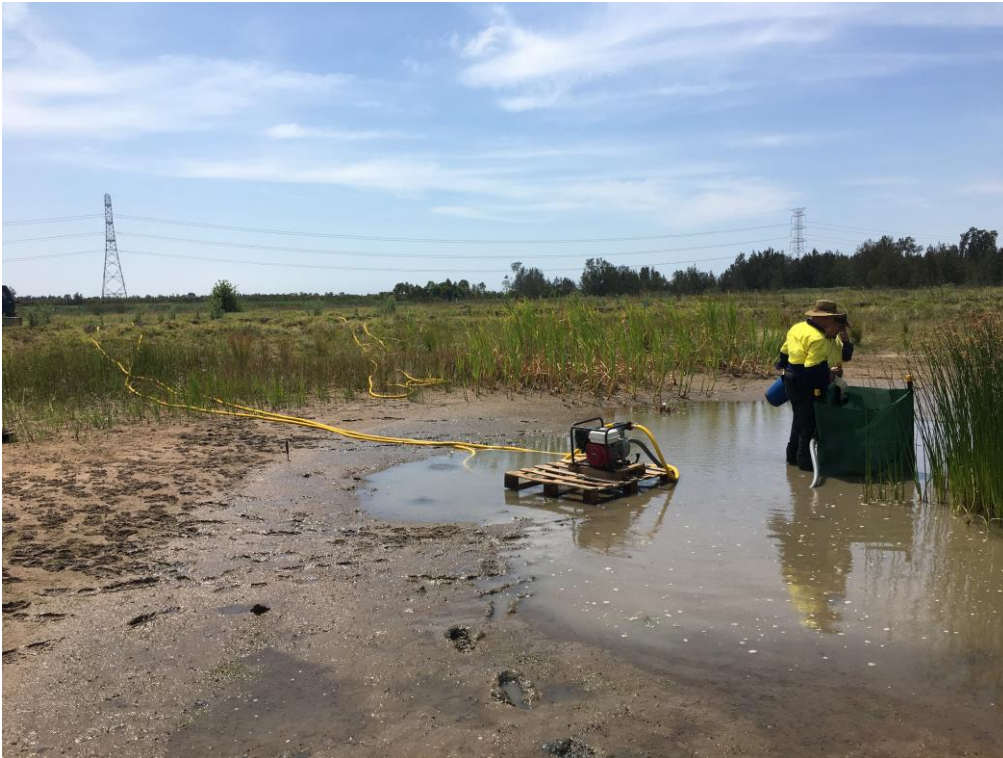
Pond 16 dewatering setup
