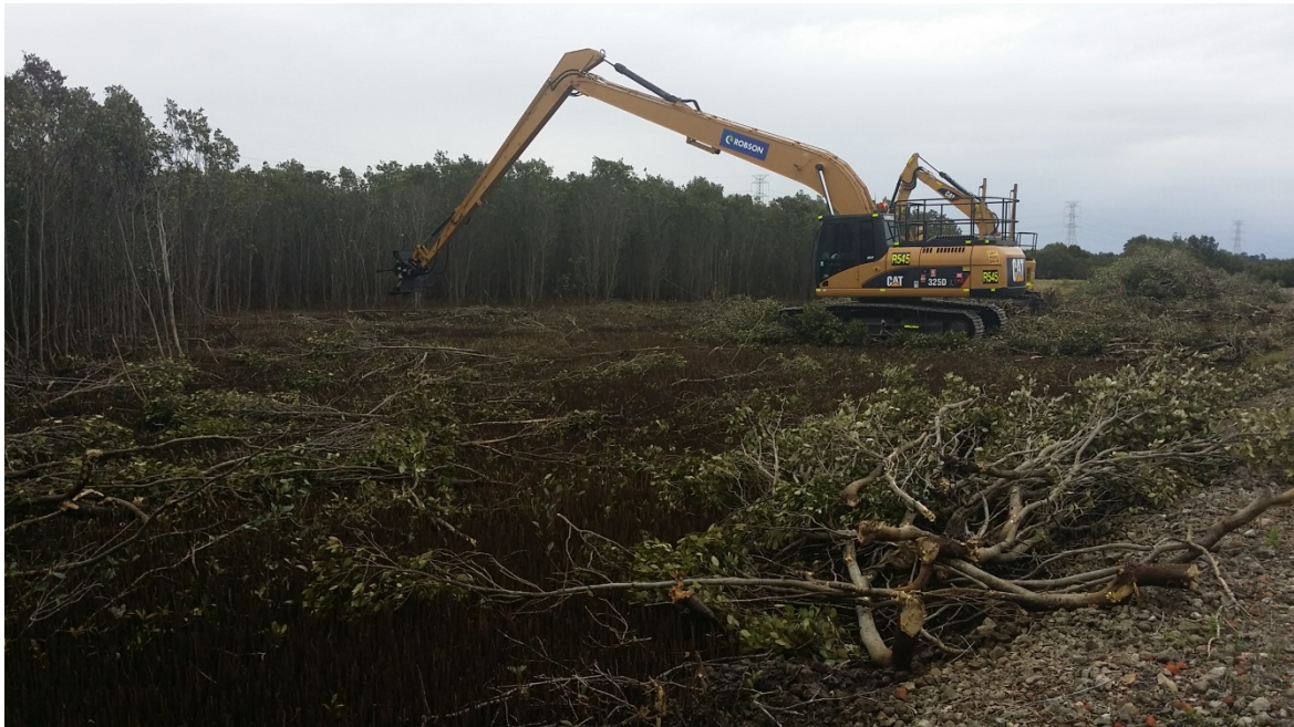
Plate 3: Long reach excavator removing mangroves with hydraulic shear
