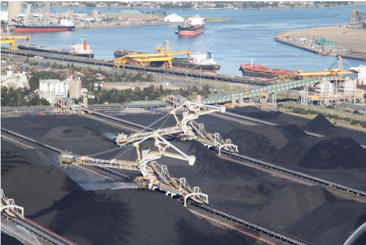
Figure 5: Stockyard with Stacker Reclaimers in Operation
