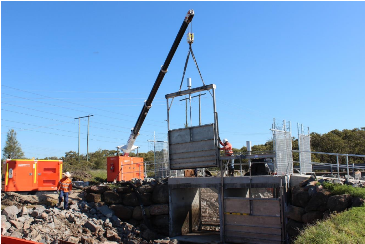
Plate 26: Intallation of Smart Gate
