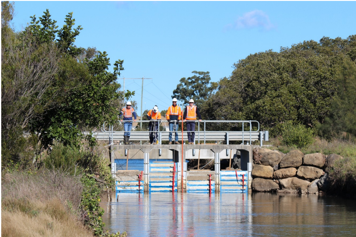
Plate 13: Utilisation of drop boards at Fish Fry Creek to manipulate tide level in work zone
