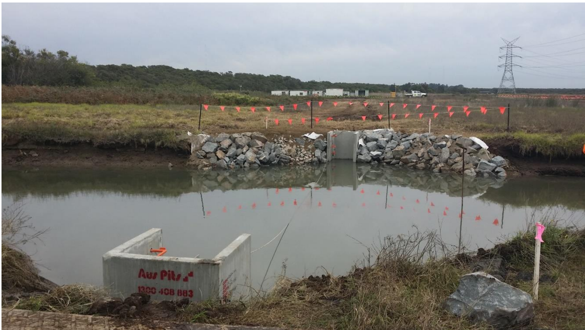
Plate 15: Installation of concrete pits for MPED 1
