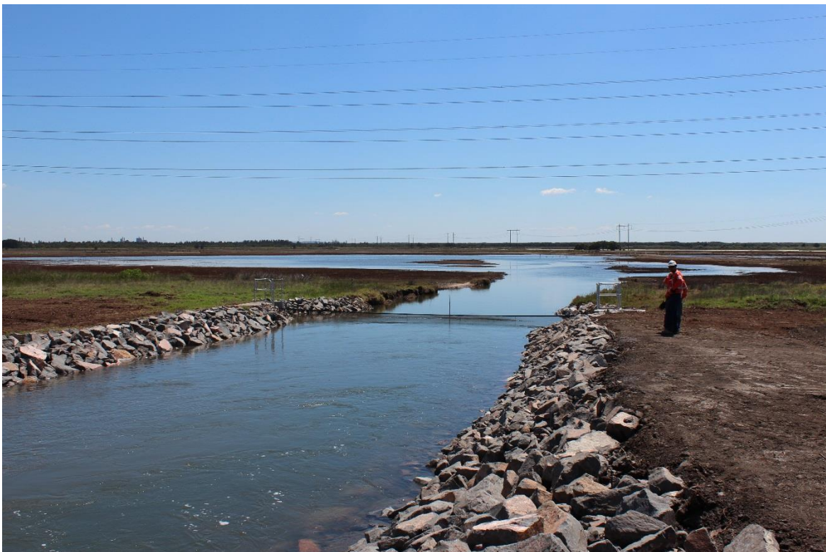
Plate 27: Rock protection along Fish Fry Creek
