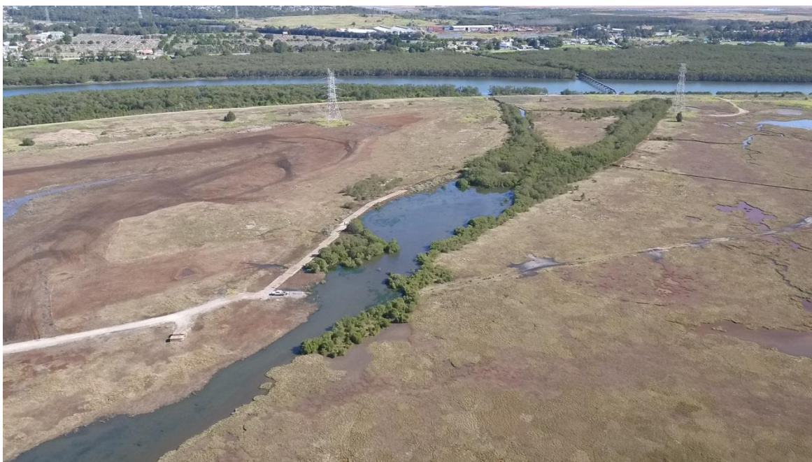
Plate 6: Wader Creek, mangroves partially removed
