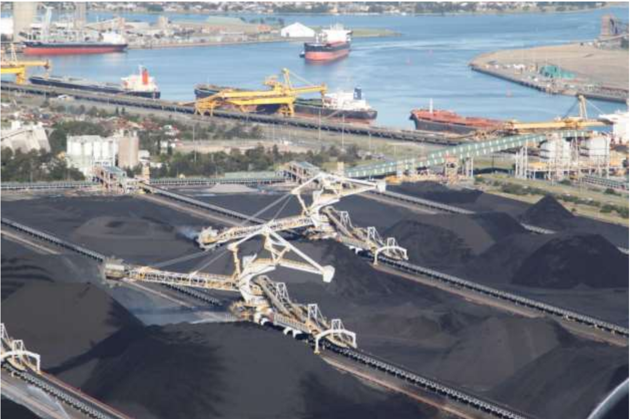
Figure 2-3: Stockyard with Stacker Reclaimers in Operation
