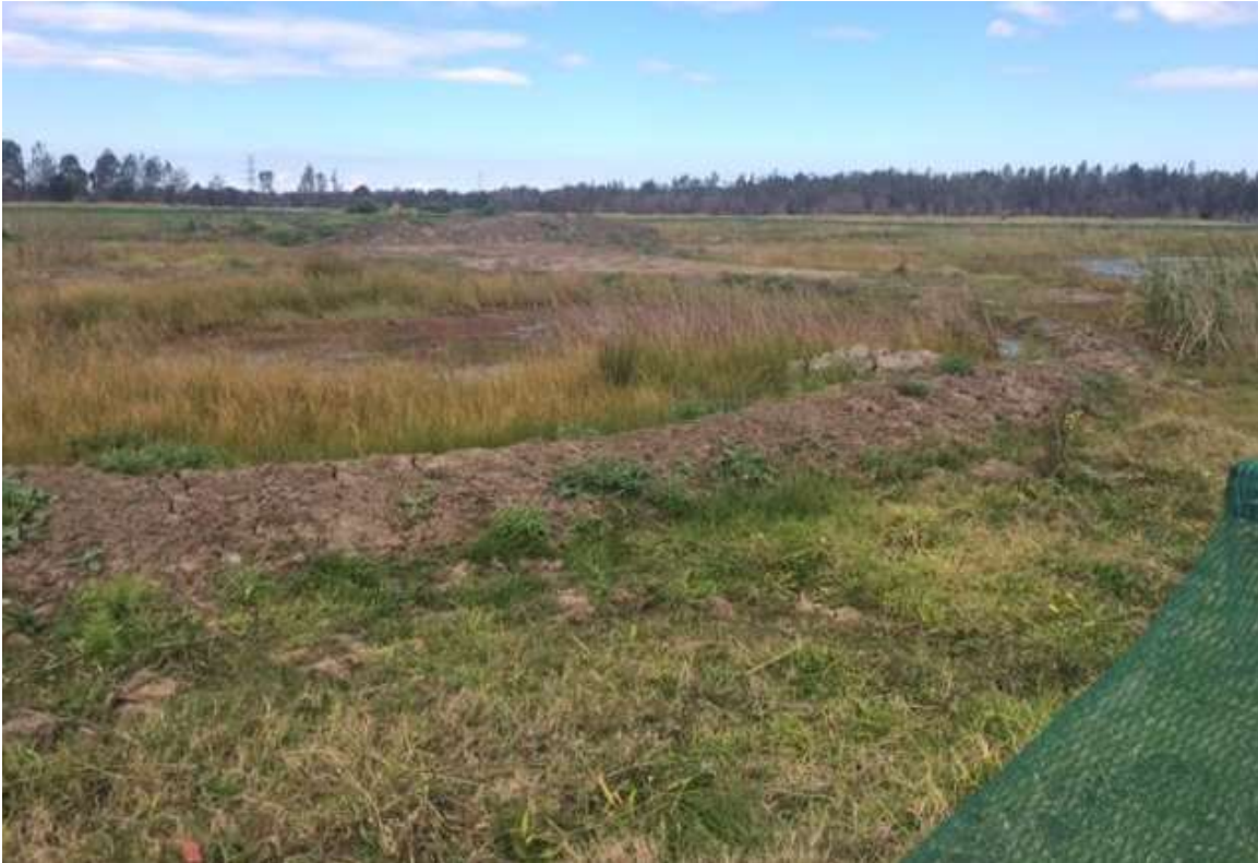
Figure 4-15: New Bunding at Stage 1
