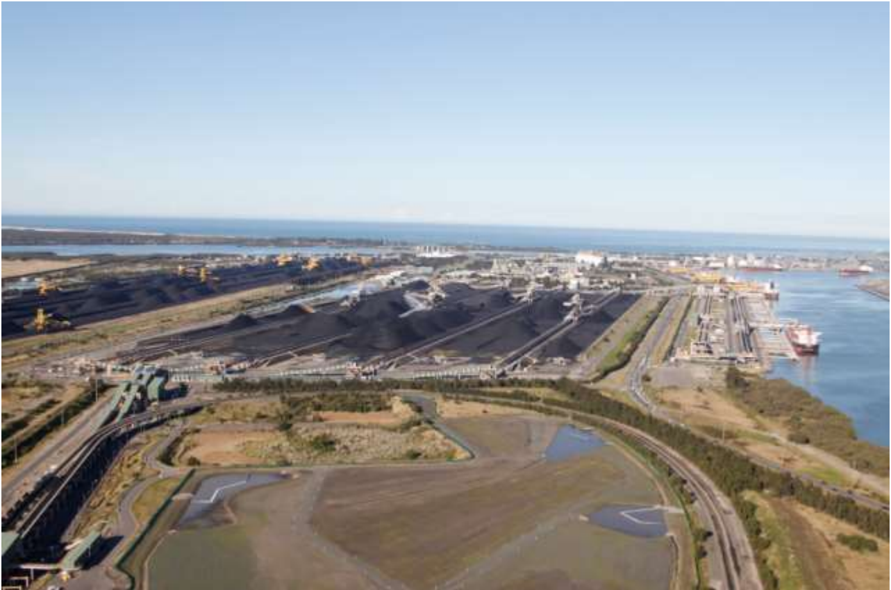
Figure 2-1: NCIG Site Overview Facing East
