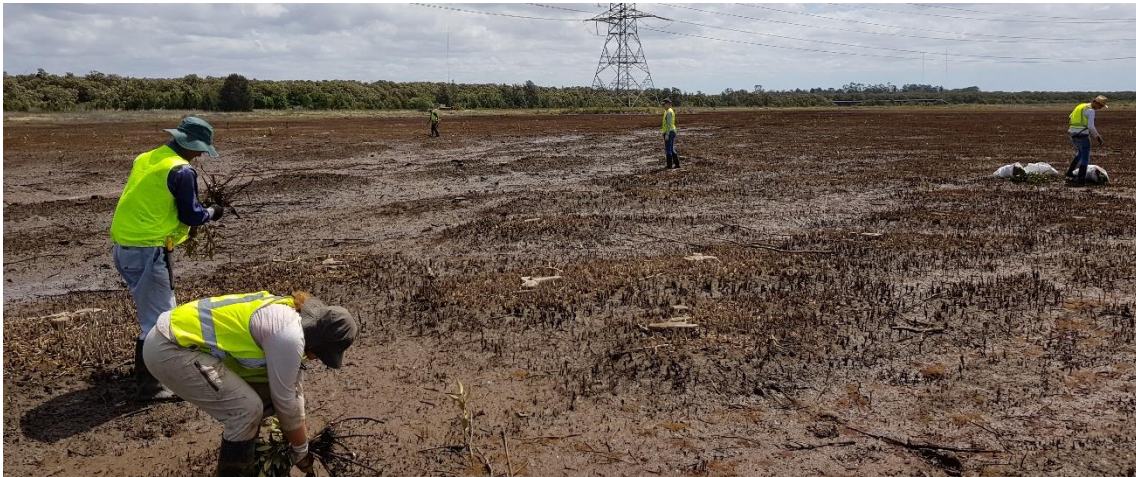
Figure 7: Conservation Volunteers Australia removing the mangroves
