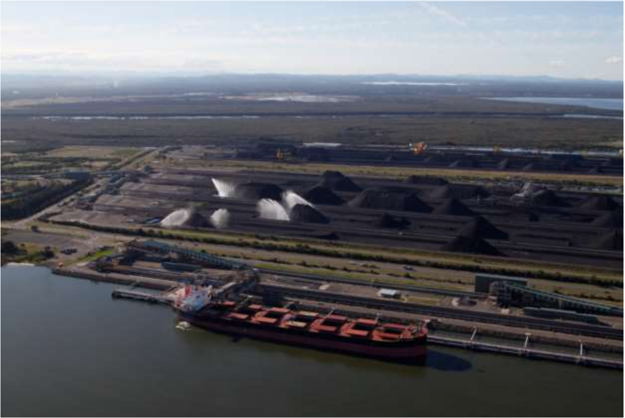
Figure 2-2: NCIG Site Overview Facing North
