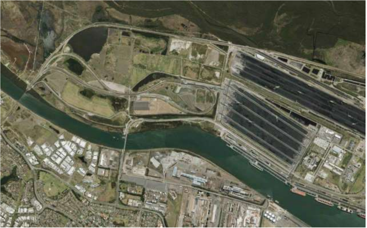
Figure 2-4: Aerial Photograph of NCIG Terminal
