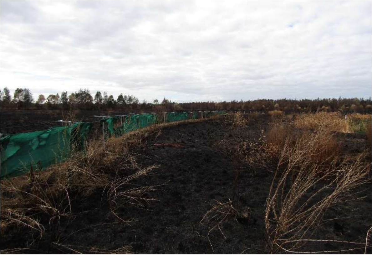
Figure 4-13: Damage to frog fencing at Stage 1 after the fire
