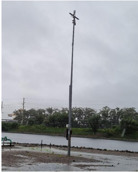
Photograph 7- Meteorological Station (taken 3/3/22)
