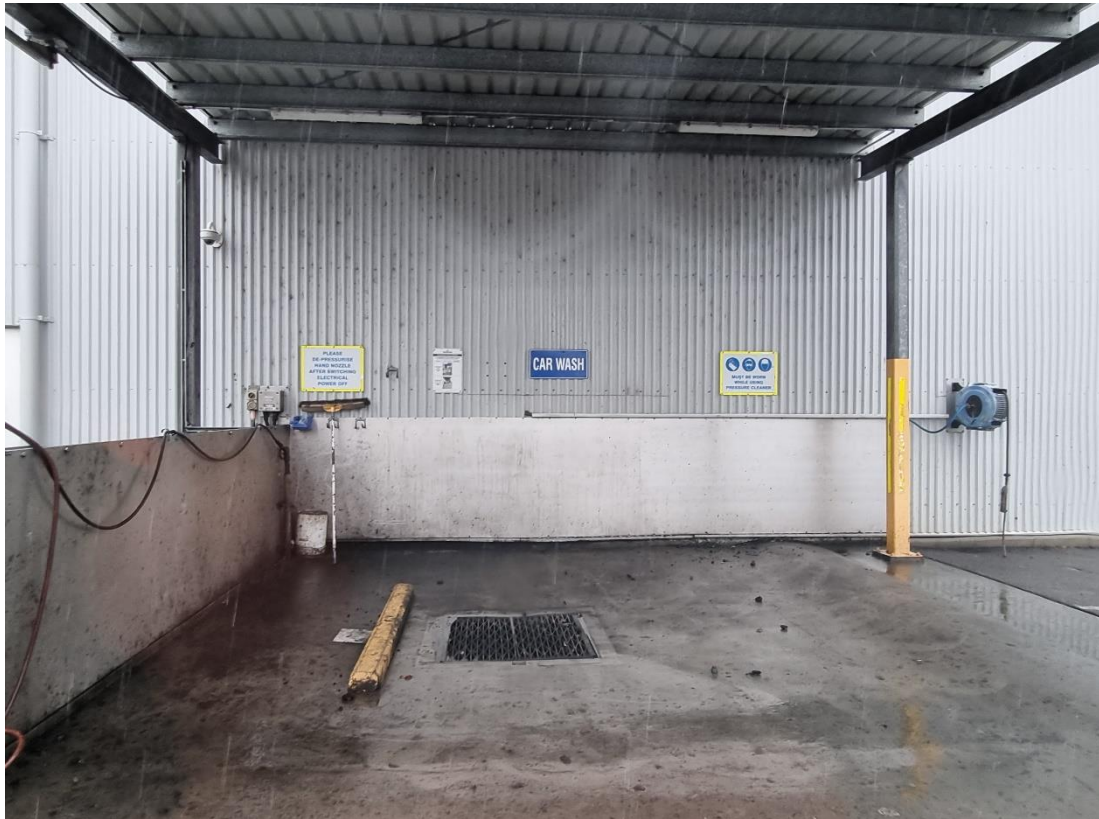
Photograph 1 - Light Vehicle Wash Bay (taken 3/3/22)
