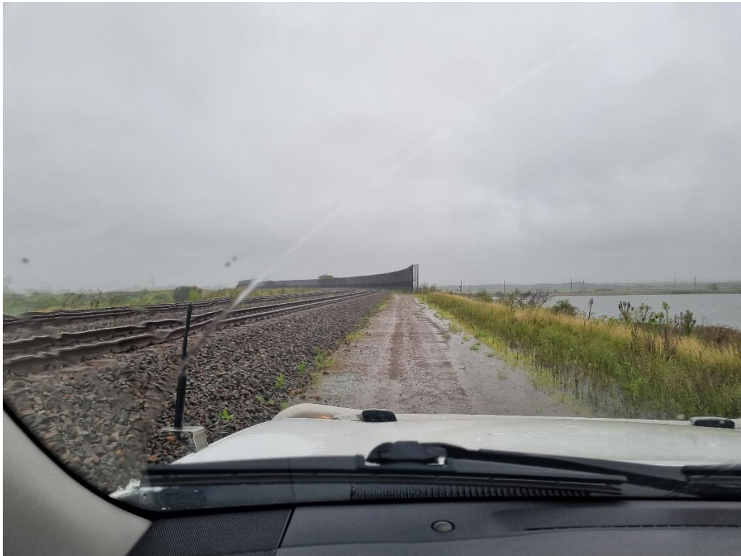
Photograph 3 - Rail Loop Lighting Screen (taken 3/3/22)
