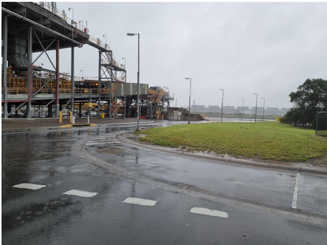
Photograph 2 - Sealed internal roads (taken 3/3/22)
