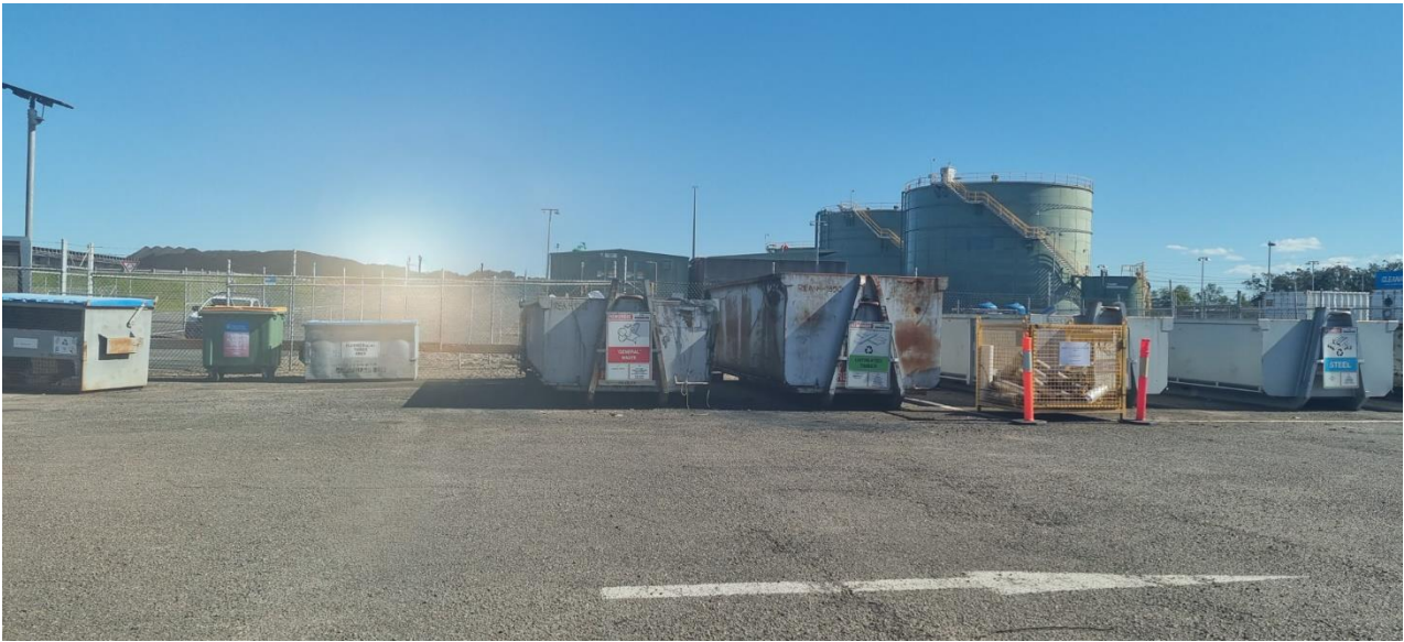
Photograph 10 Bulk Waste Management Area
