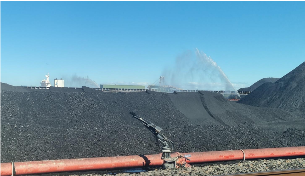
Photograph 3 - Dust suppression sprays operating on the coal stockpiles.
