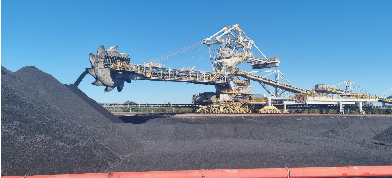
Photograph 1 Operational Coal Stacker
