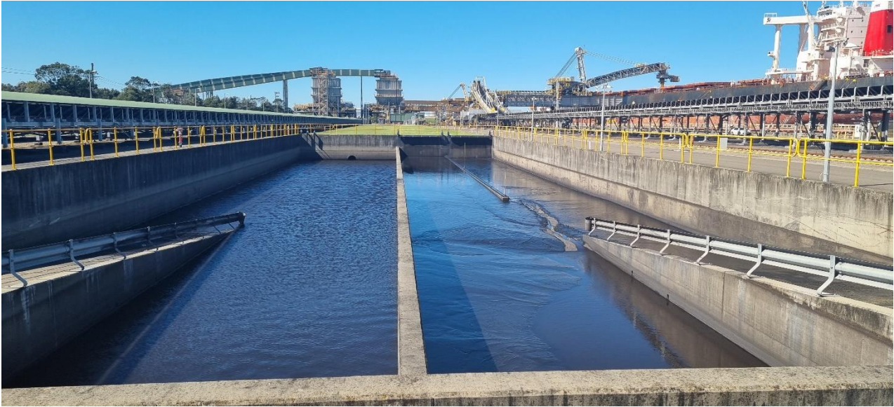
Photograph 7 – stormwater collection / sediment basins located at NCIG's wharf facility adjacent to shiploading operations.
