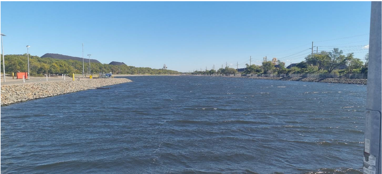
Photograph 8 – main stormwater collection / storage (lined) pond (WT30)
