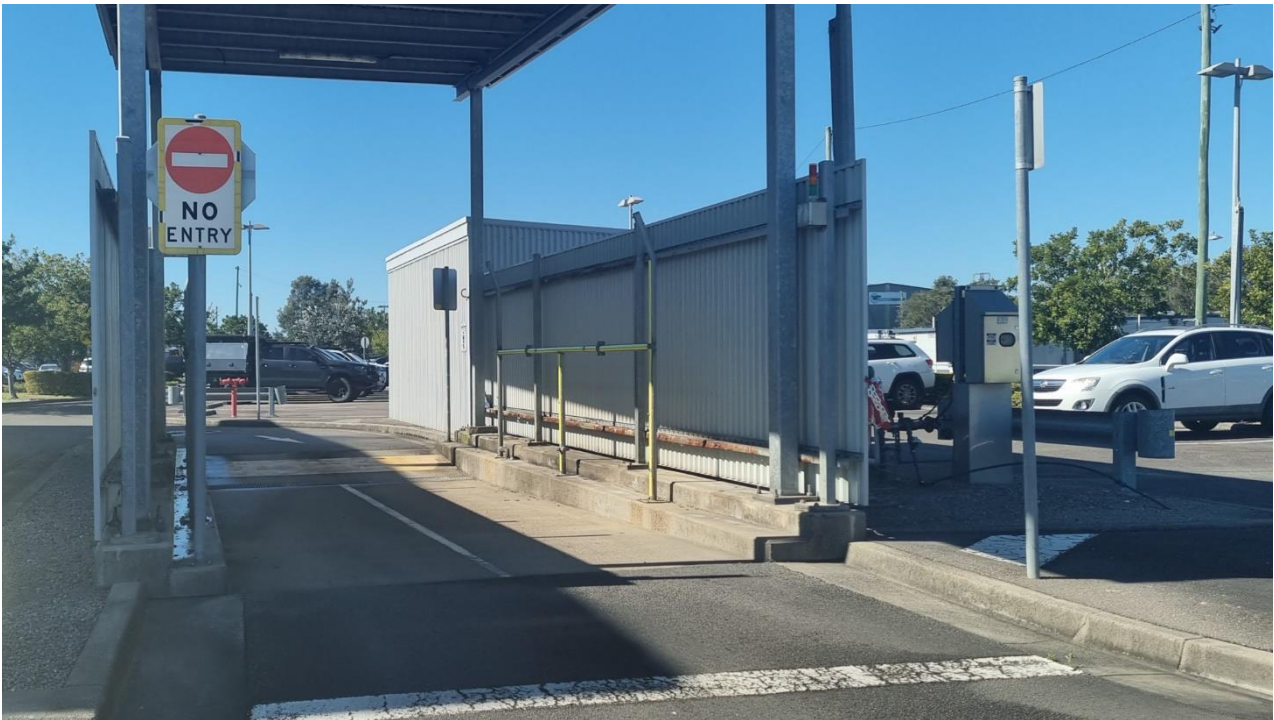
Photograph 6 –Vehicle wash station adjacent NCIG administration building.
